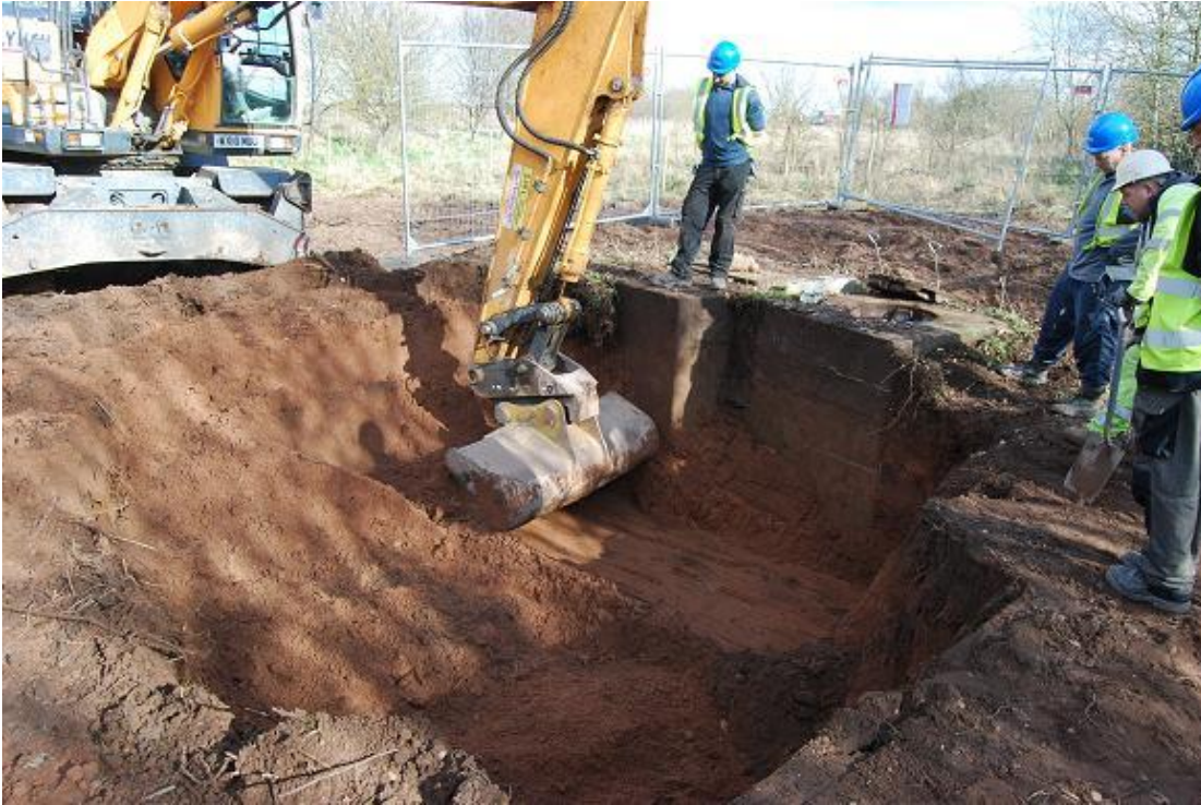
Plate 1 Trench during excavation, view north-east
