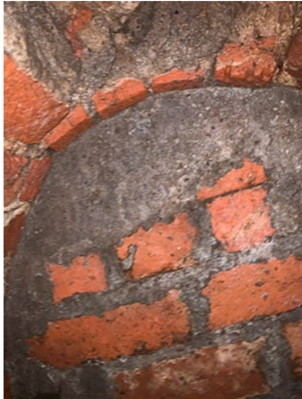
Plate 21a/b: Internal views of brick culvert 1017: (a) inserted pipe to south-east; (b) brick wall blocking to north-east, possibly inserted due to damage from modern drainage
