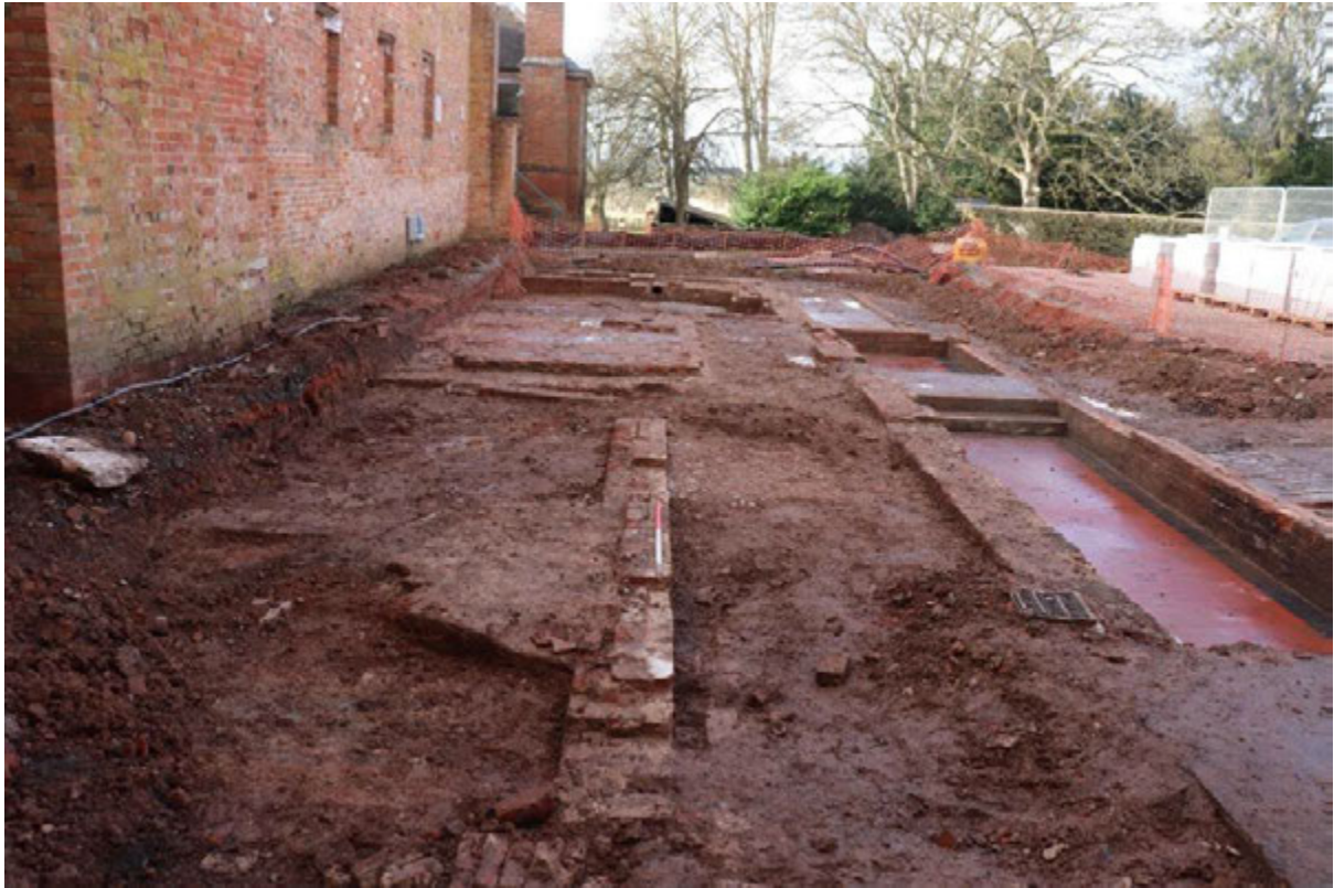
Plate 3: Wall 2026 (south-east end) cut by later scullery floor 1024 and pipes, butted by cobbles 1037, view north-west; 1m scale
