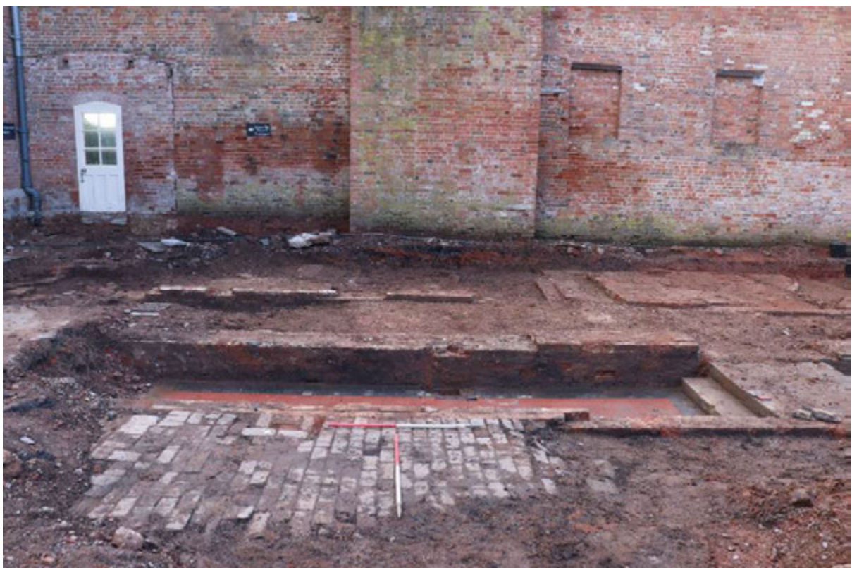
Plate 16: Coal stained grey brick floor 1009 to north-east side of building, view south-west to parterre wall; 2x 1m scales
