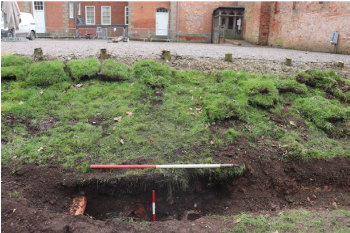
Plate 20: Top of culvert brick arch 1017, disturbed by modern services, on turfed slope at north-west edge of main excavation area, view south-east; 0.4m and 1m scales (initially exposed during the watching brief for the Biomass Boiler; WSM 77814; Arnold and Vaughan 2022)
