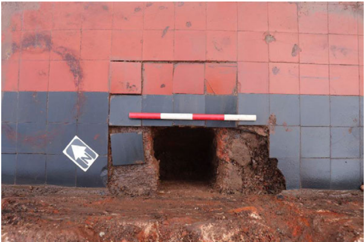
Plate 6: Tiled surface of porch corridor 1013 (south-east), with BA evaluation sondage to culvert 1017, view north-east; 0.4m scale
