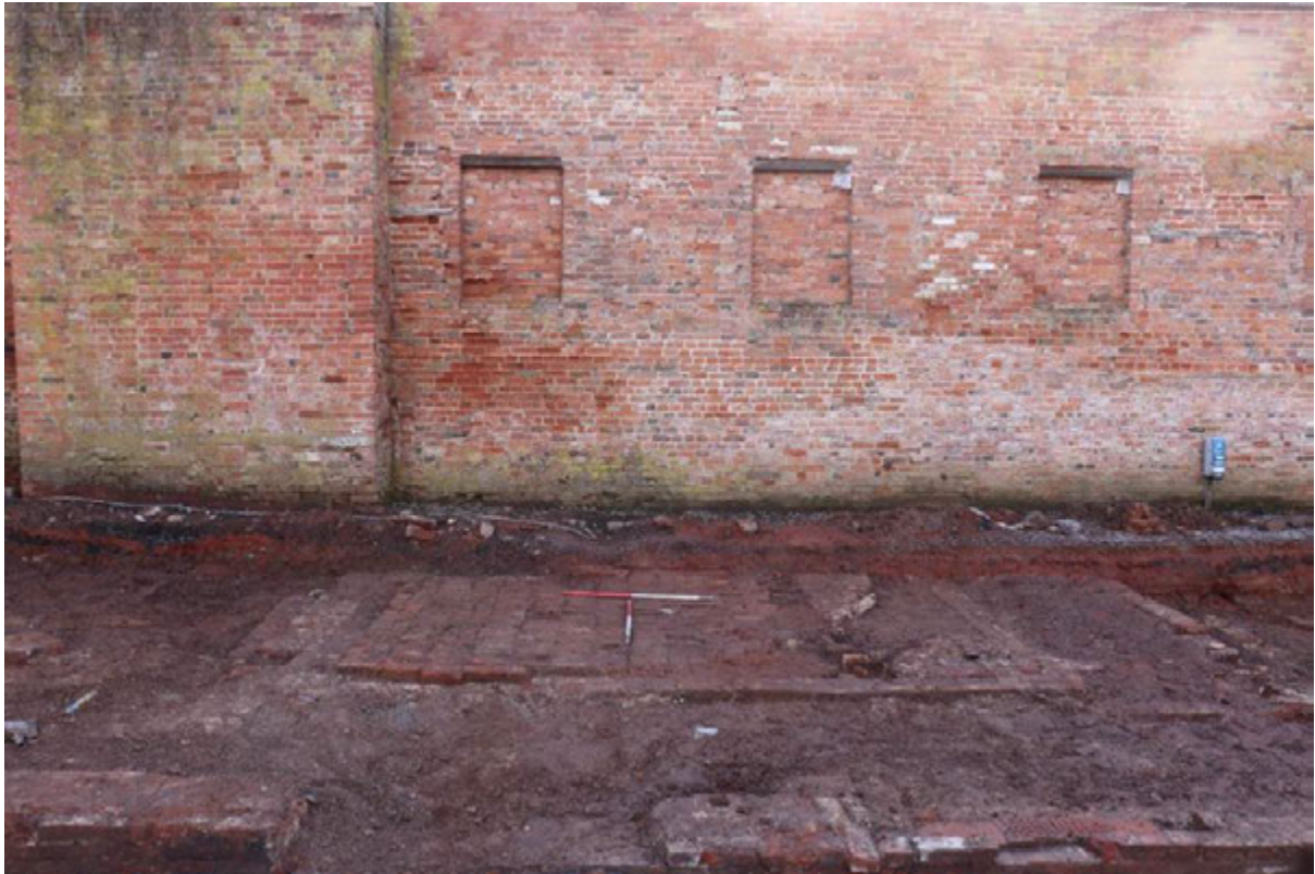
Plate 17: Brick floor of Scullery 1024, view south-west to parterre wall; 2x 1m scales
