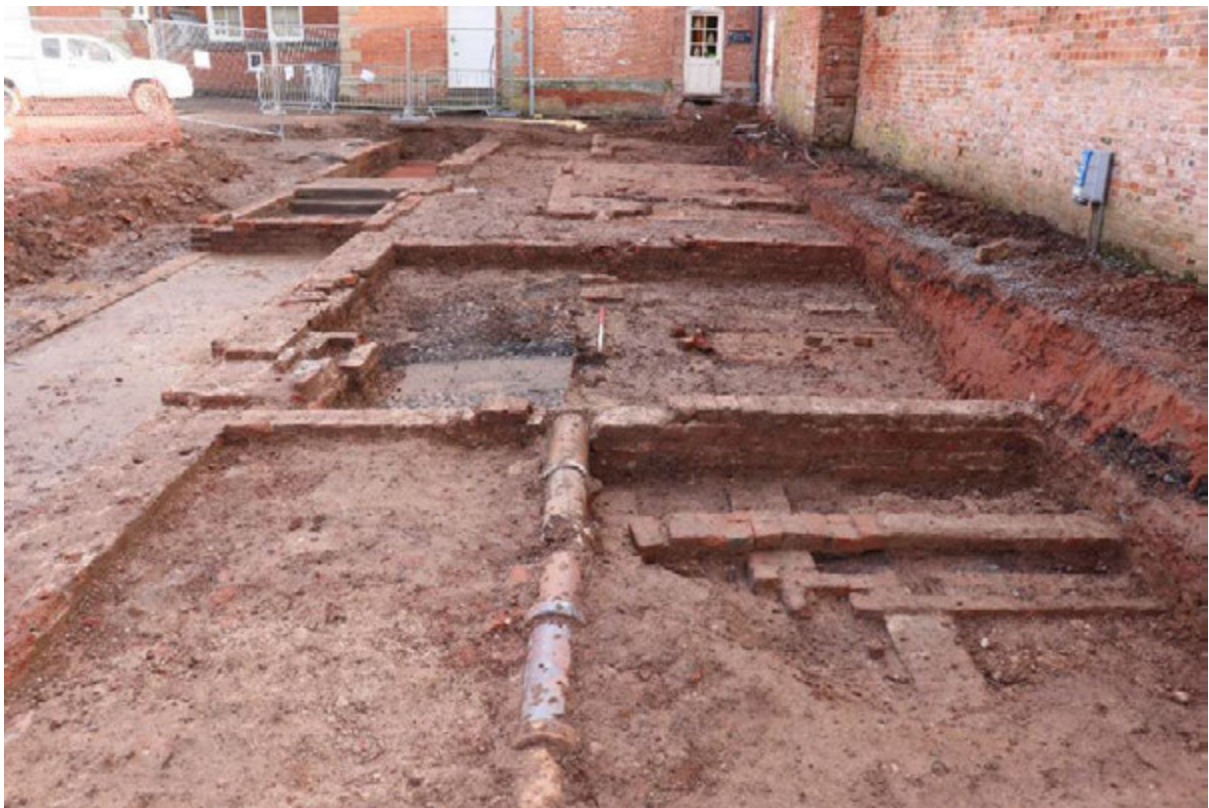
Plate 4: Alignment of wall 1020, cut by later drainage 1046 from scullery, abutted by cobbles 1022 and slab 1023, in the background; walls 1018, 1039 and 1041 in the foreground; view south-east; 1m scale
