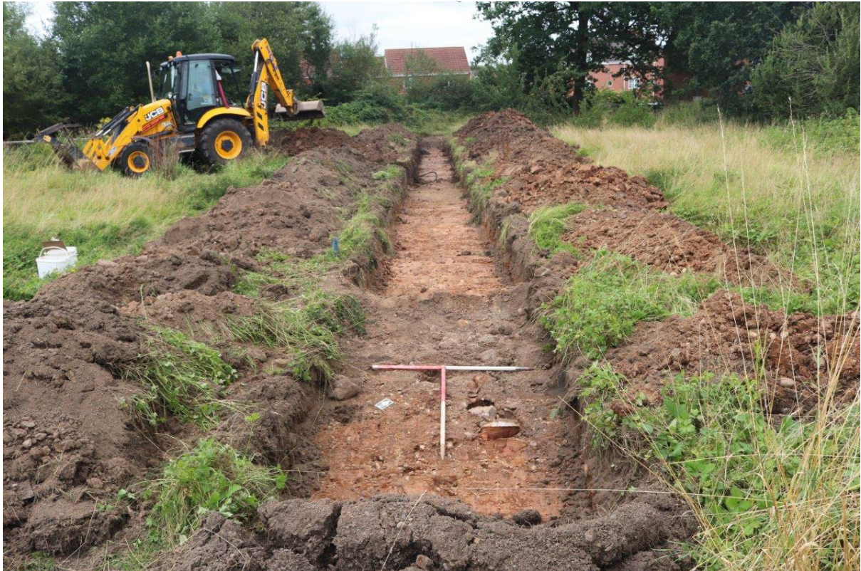
Plate 1 Trench 1 looking north (1m scales)
