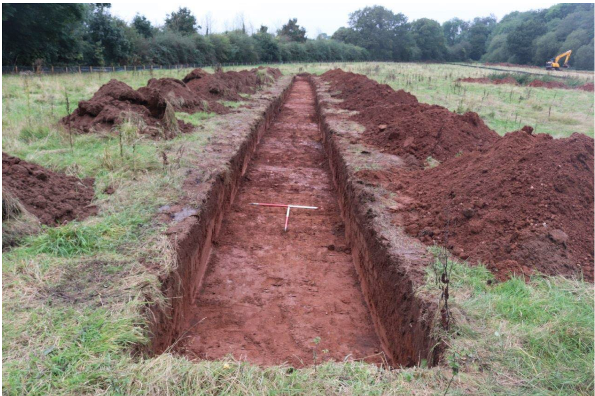
Plate 8 Trench 4 looking west. 1m scales
