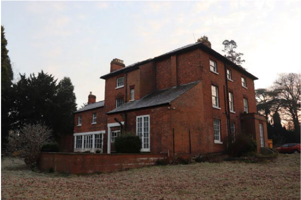
Plate 3 External, looking north-east, 1m scale
