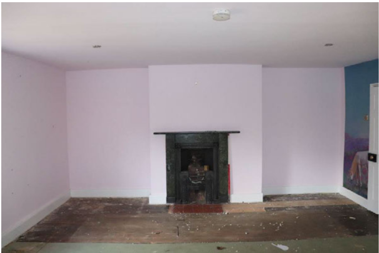
Plate 60 Room S4, looking west, 1m scale
