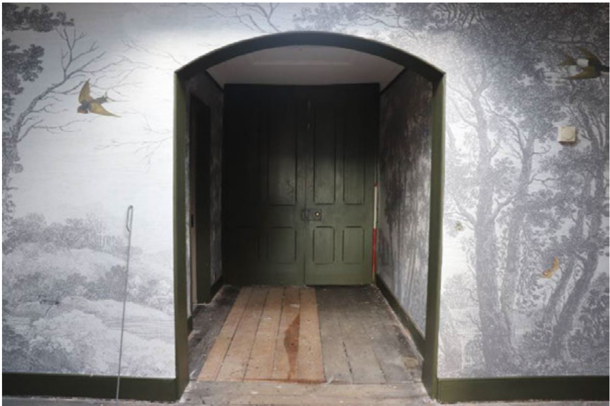
Plate 56 Room S1, looking north, 1m scale
