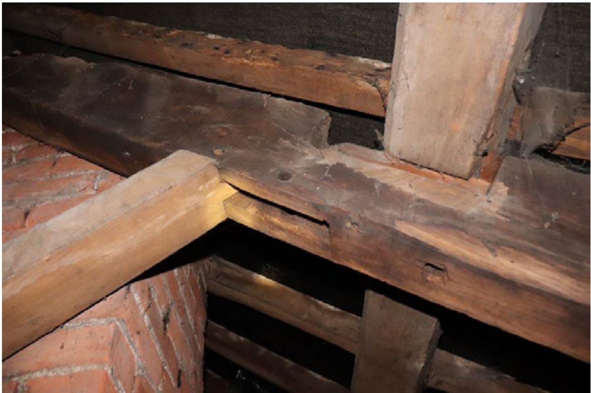
Plate 67 Roof space above Room S1, looking north-east
