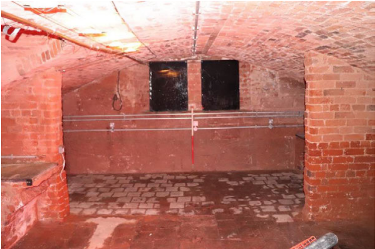
Plate 35 Room B1, looking east, 1m scale
