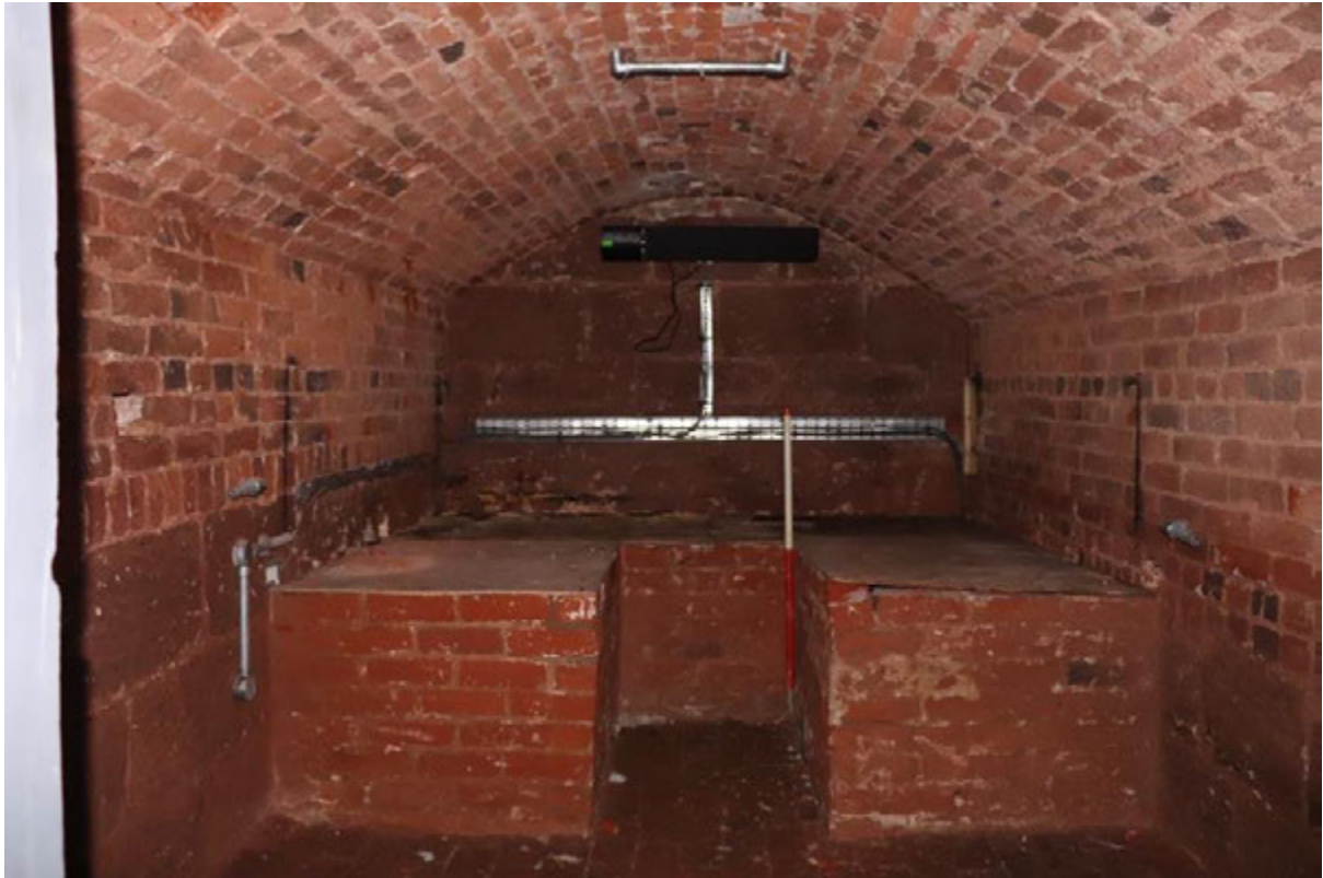
Plate 31 Room B7, looking east, 1m scale
