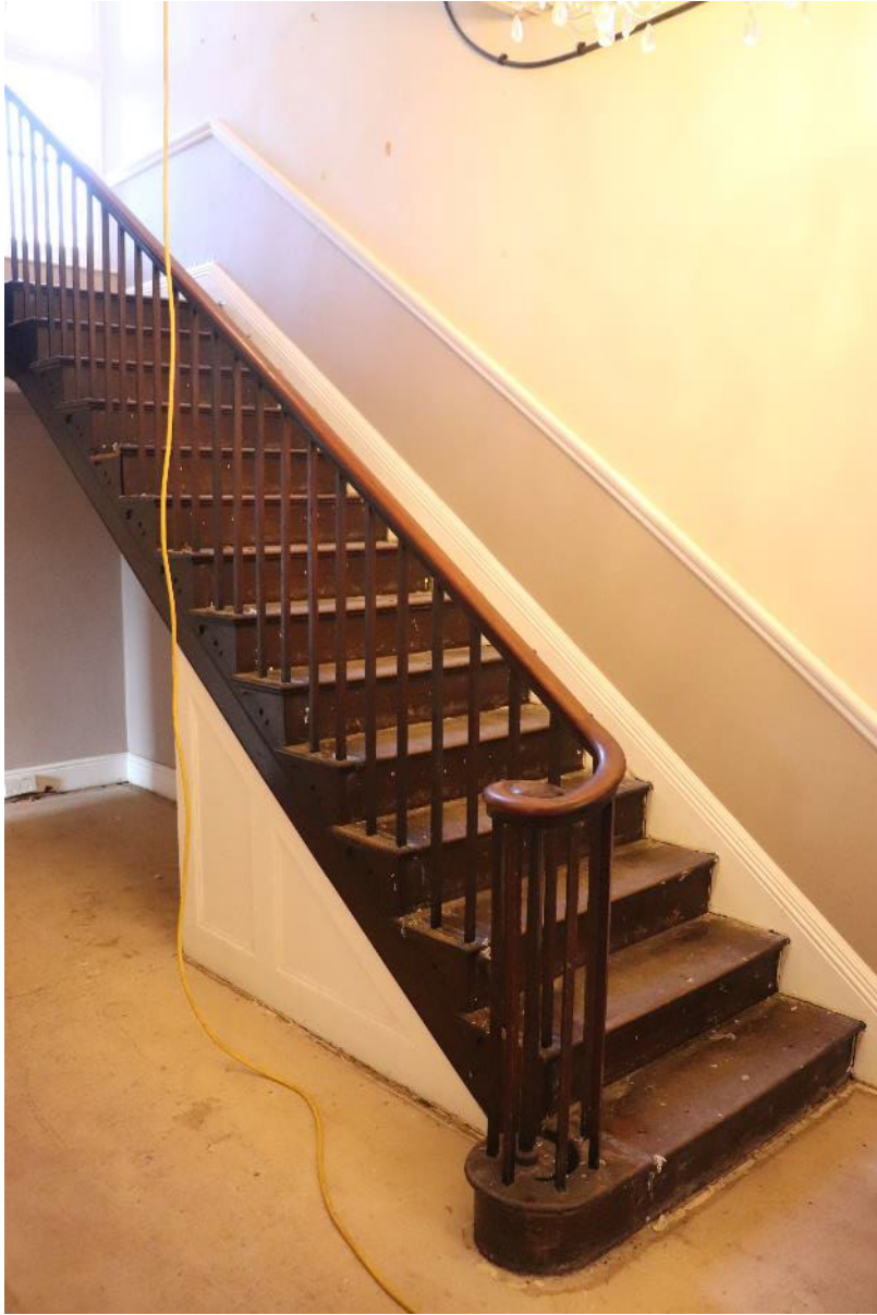
Plate 14 Room G1, looking north-west, 1m scale
