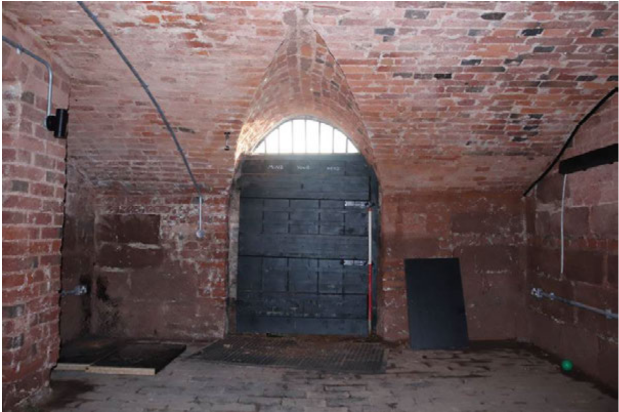
Plate 39 Room B4, looking south, 1m scale
