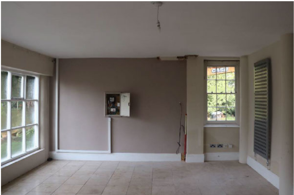
Plate 74 Room G5, looking north, 1m scale
