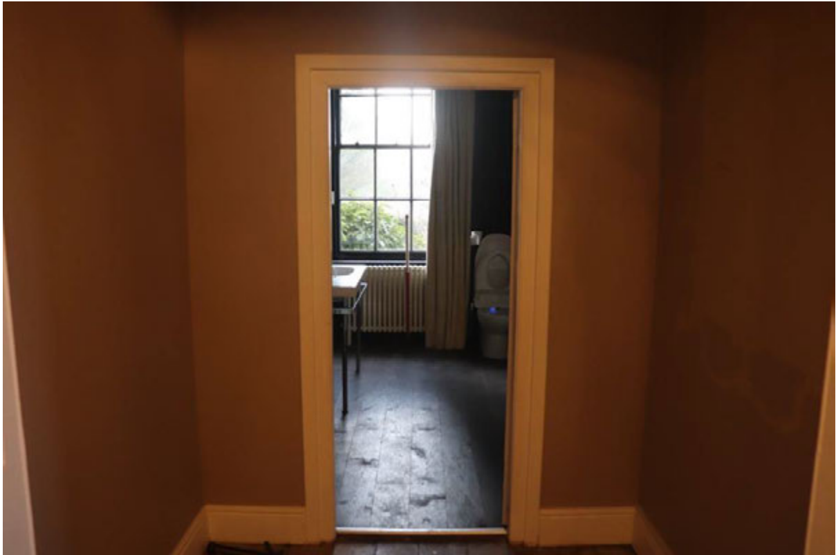
Plate 10 Room G9, looking south, 1m scale
