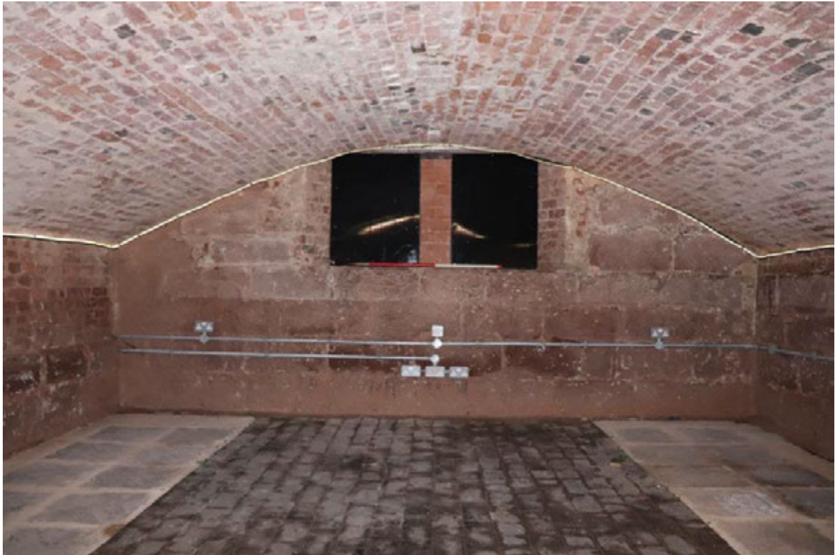
Plate 37 Room B6, looking east, 1m scale
