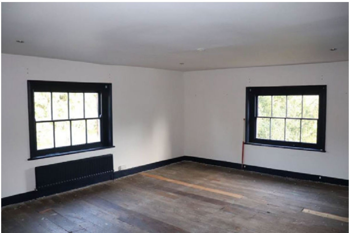
Plate 58 Room S2, looking north-east, 1m scale
