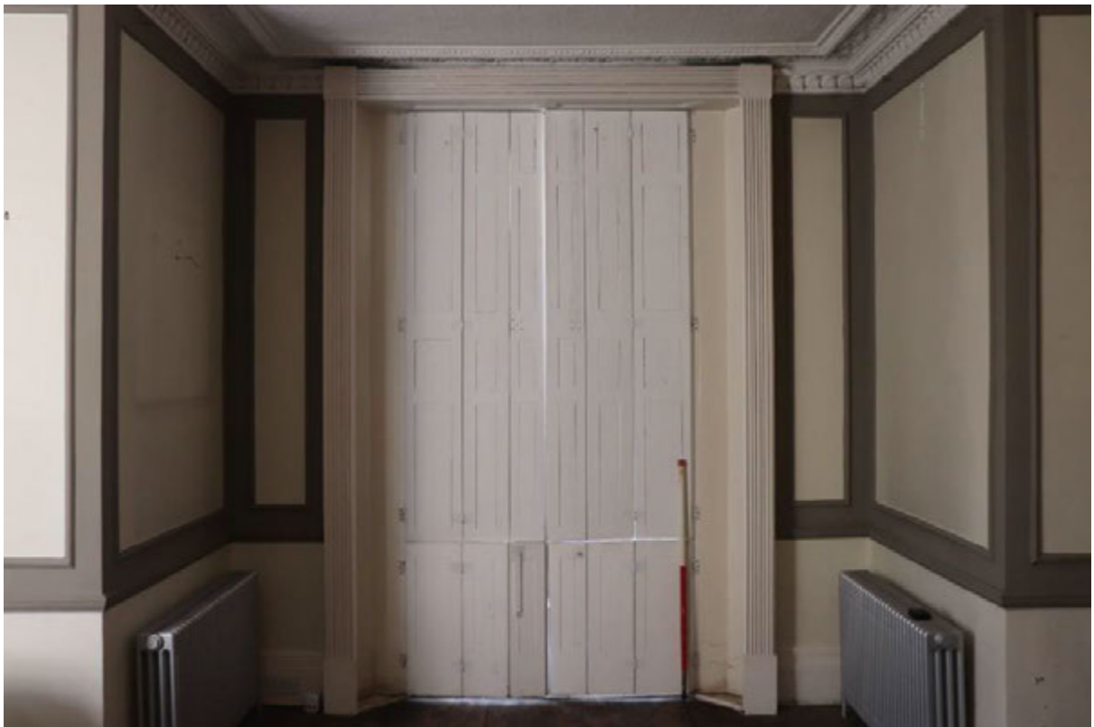
Plate 70 Room G2, looking south, 1m scale
