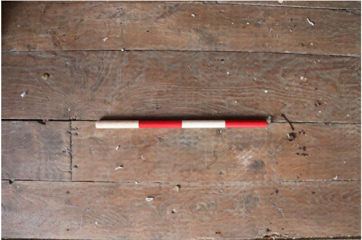
Plate 69 Elm floor boards room S4, 0.4m scale
