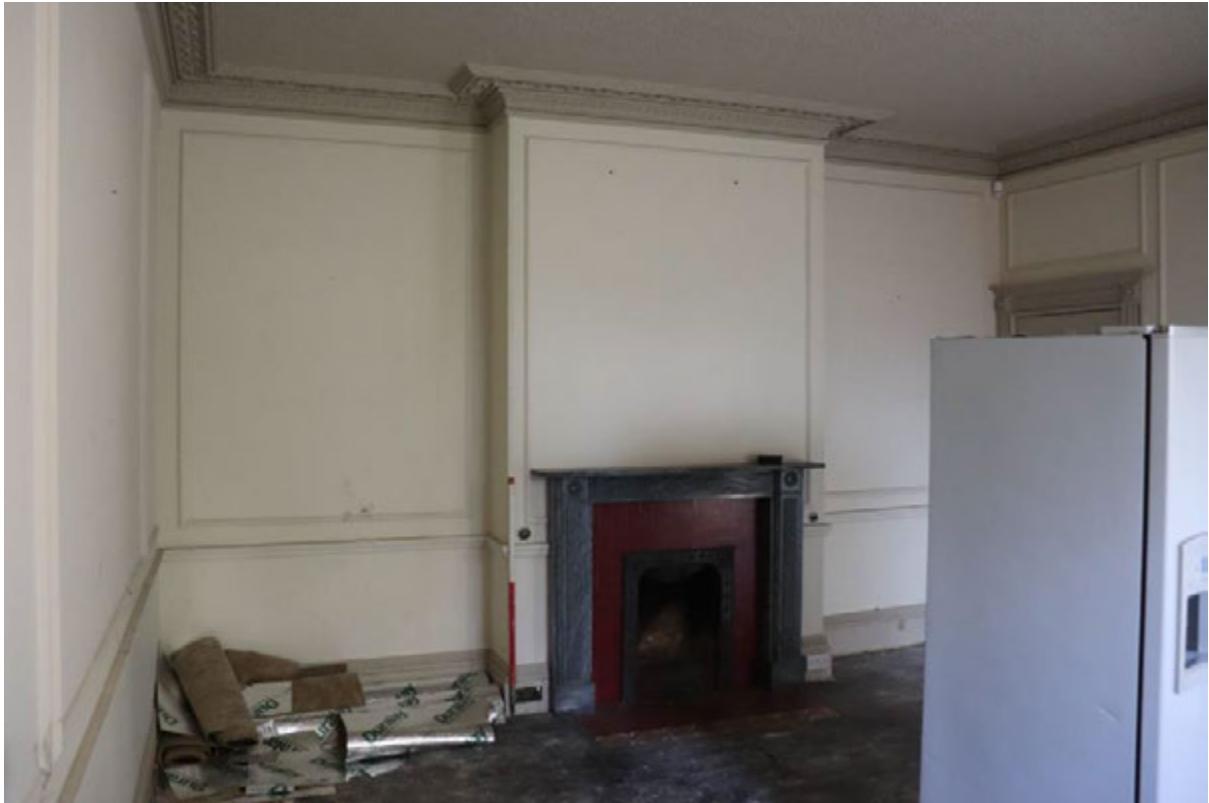
Plate 19 Room G8, looking north-west, 1m scale
