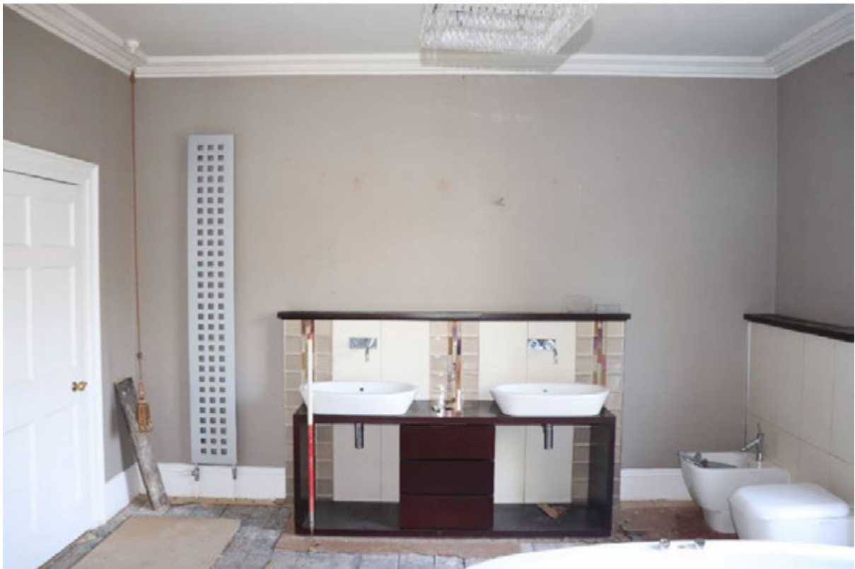
Plate 52 Room F2, looking south, 1m scale
