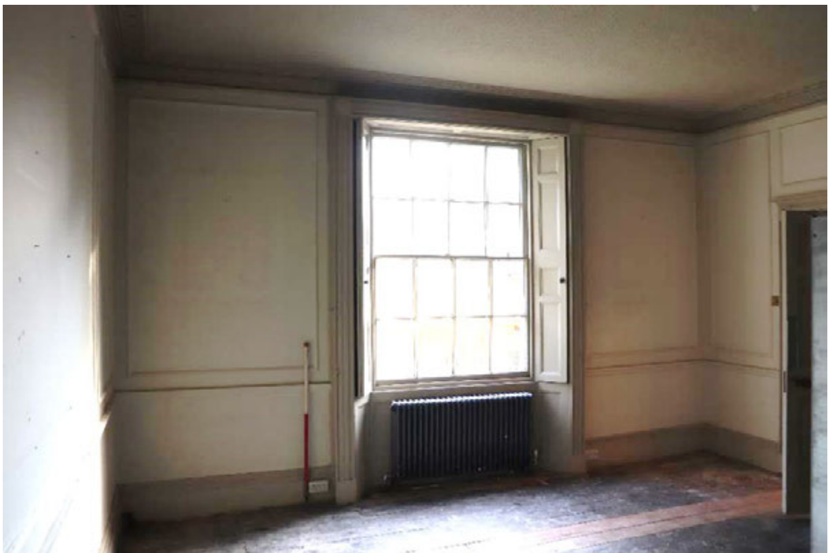
Plate 20 Room G8, looking south-east, 1m scale
