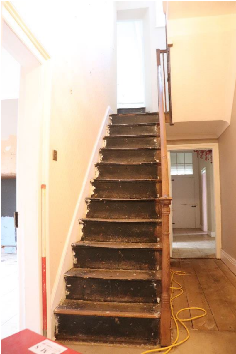
Plate 12 Room G1, looking north, 1m scale
