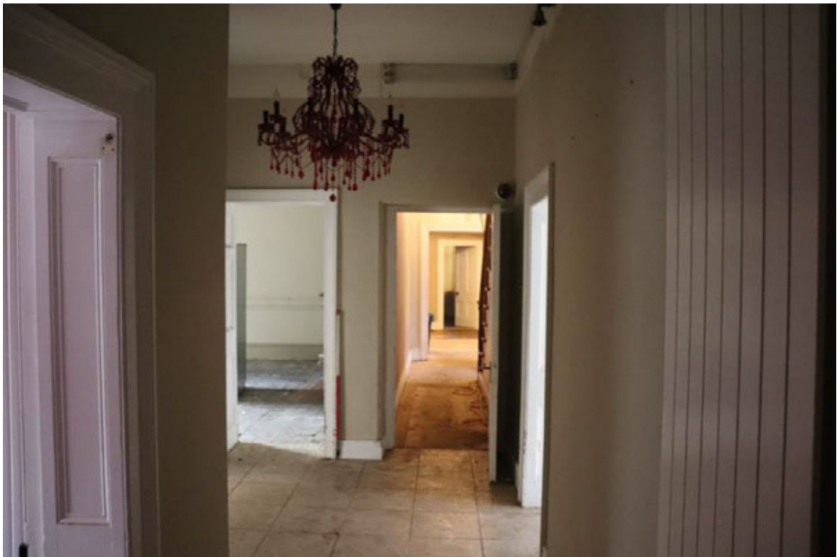
Plate 72 Room G10, looking south, 1m scale
