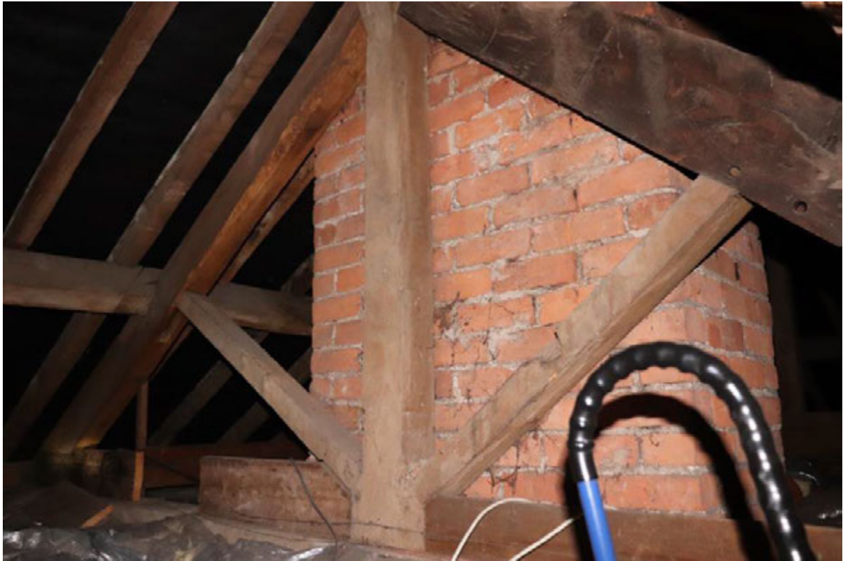
Plate 66 Roof space above Room S1, looking north-east
