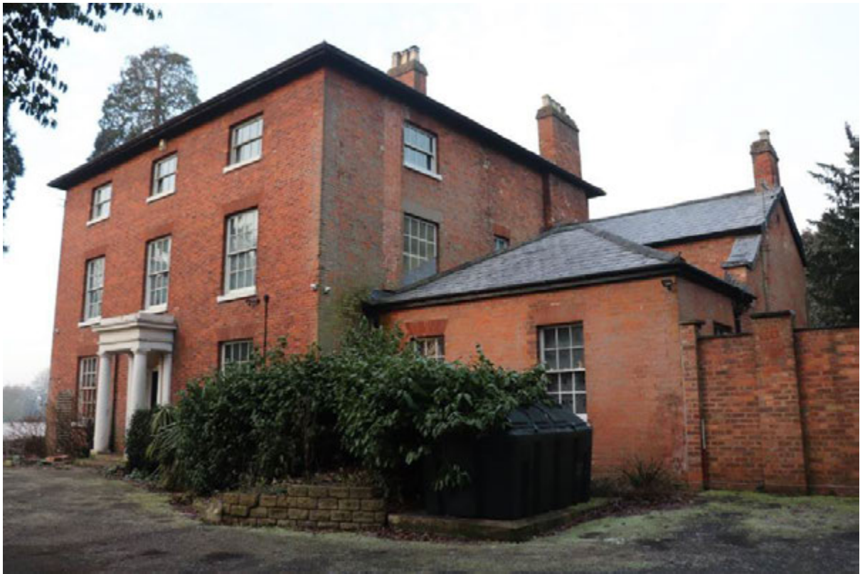
Plate 1 External, looking south-west, 1m scale
