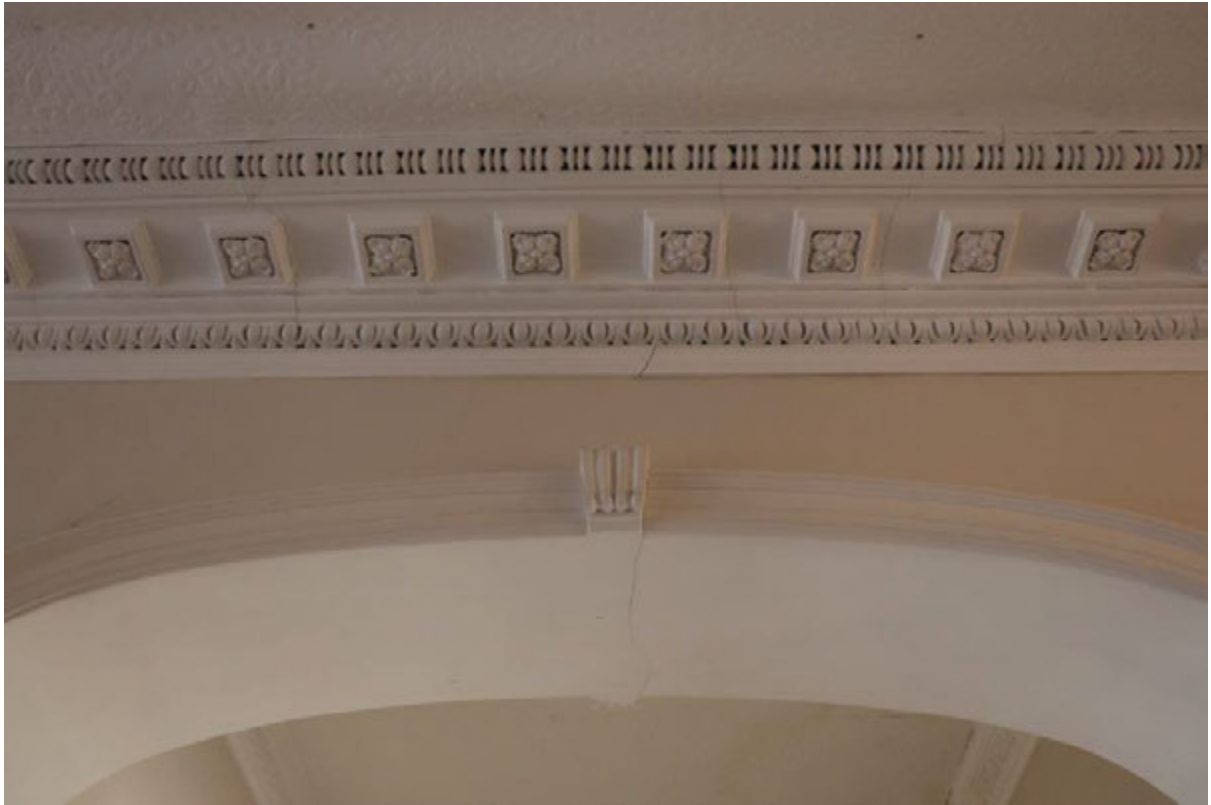
Plate 44 Room F1, looking east
