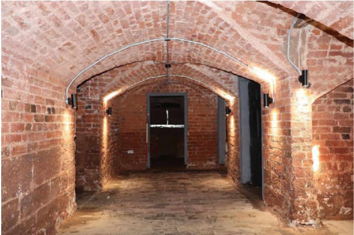
Plate 29 Room B2, looking east, 1m scale
