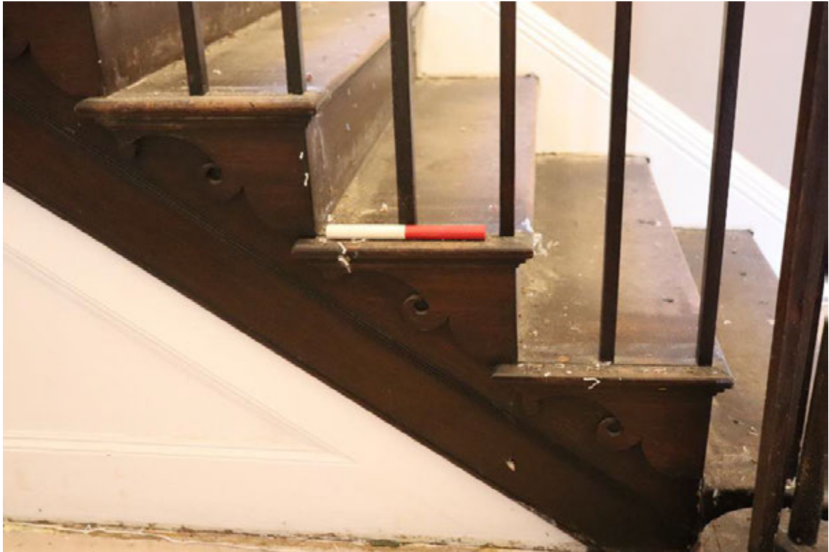
Plate 15 Room G1, looking north, 0.2m scale
