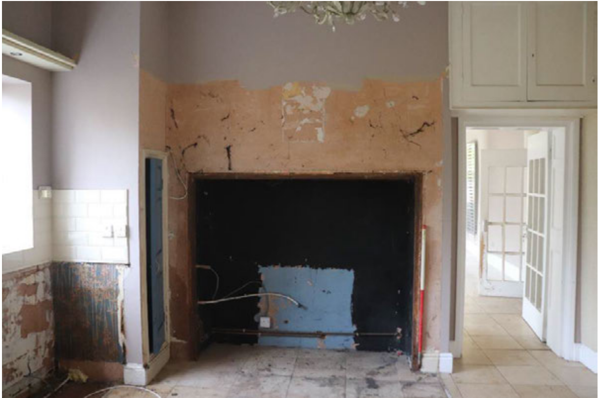
Plate 23 Room G4, looking north, 1m scale
