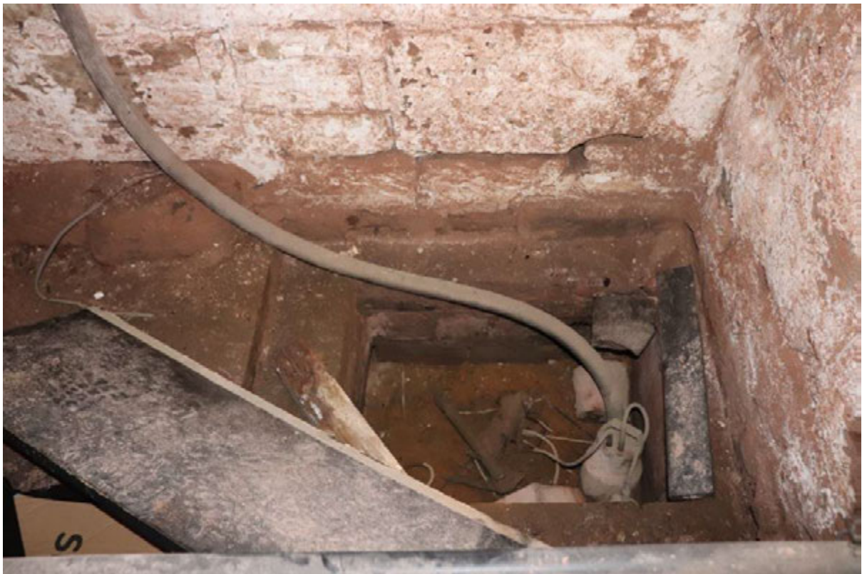
Plate 32 Room B2, looking north
