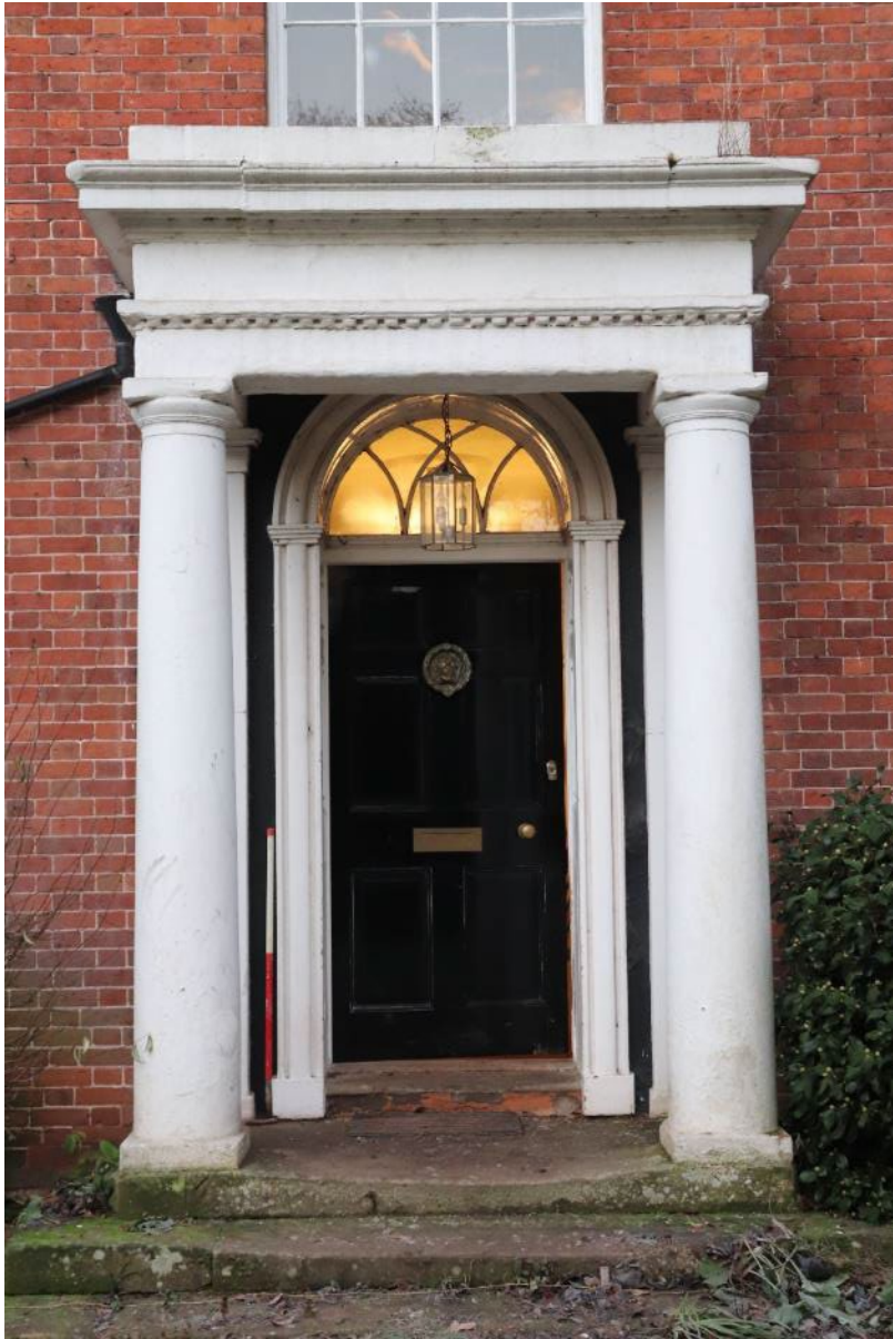
Plate 6 External, looking west, 1m scale
