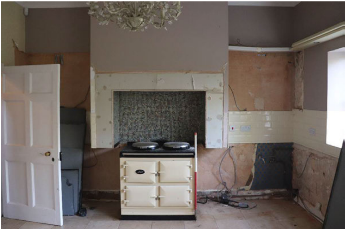
Plate 24 Room G4, looking south, 1m scale
