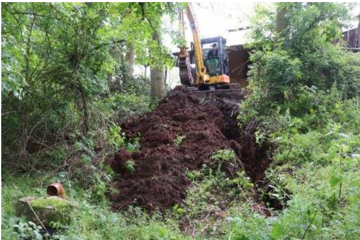
Plate 12: Trench from existing pipe to farmyard, view south-west, no scales
