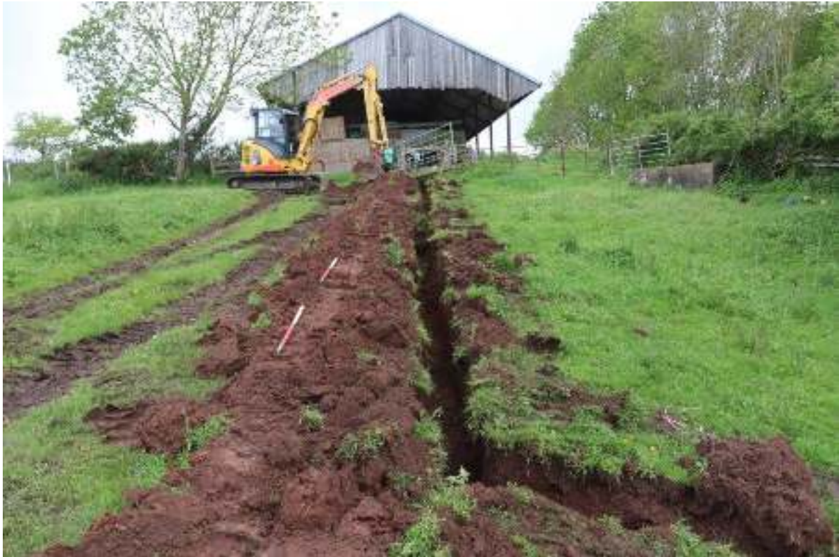
Plate 5: Trench, view north toward farmyard, 2x 1m scales
