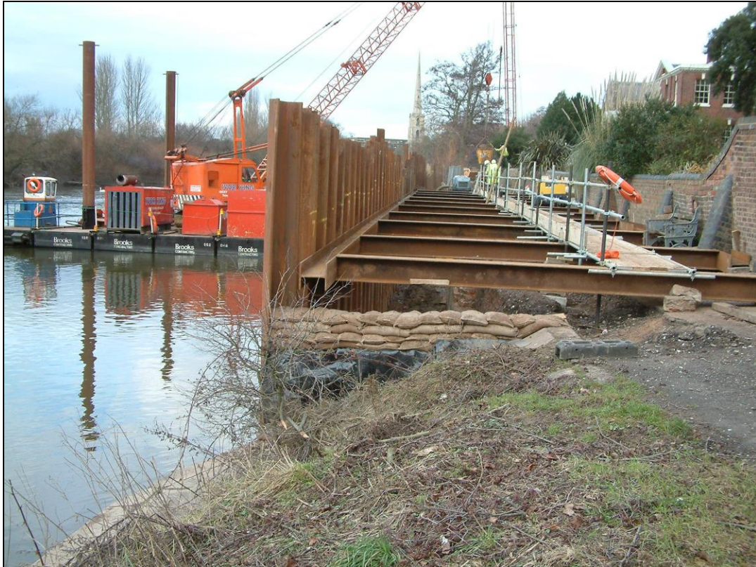
Plate 1: Cofferdam in place during repair works.
