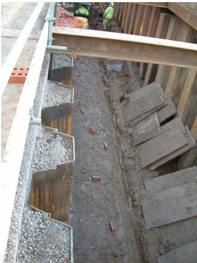
Plate 6: Remains of river walk wall after demolition.
