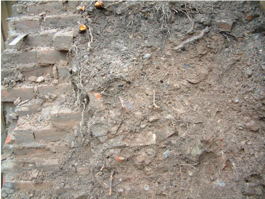
Plate 5: The river walk wall and made ground behind
