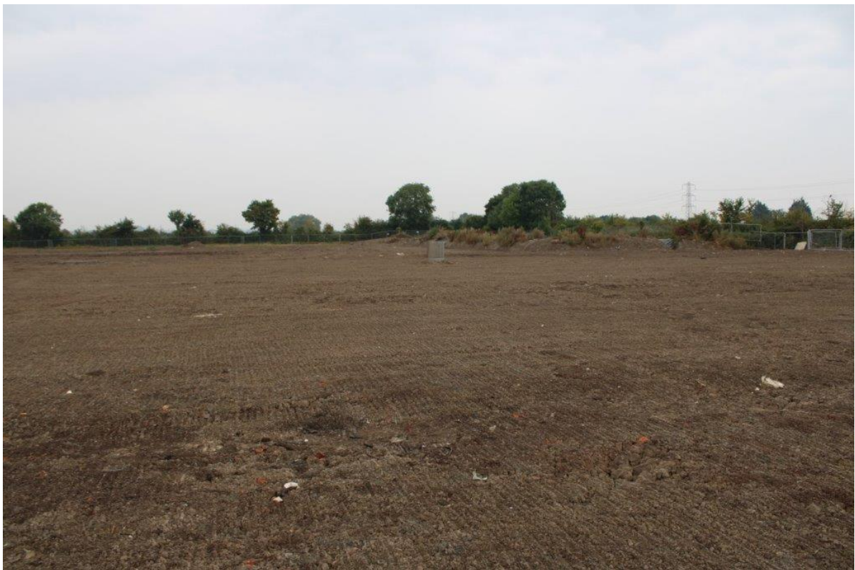
Plate 10: View across site after greenhouse demolition, view northeast towards balancing pond
