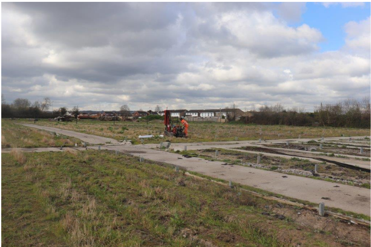
Plate 4: BH 6 location during drilling, view southwest
