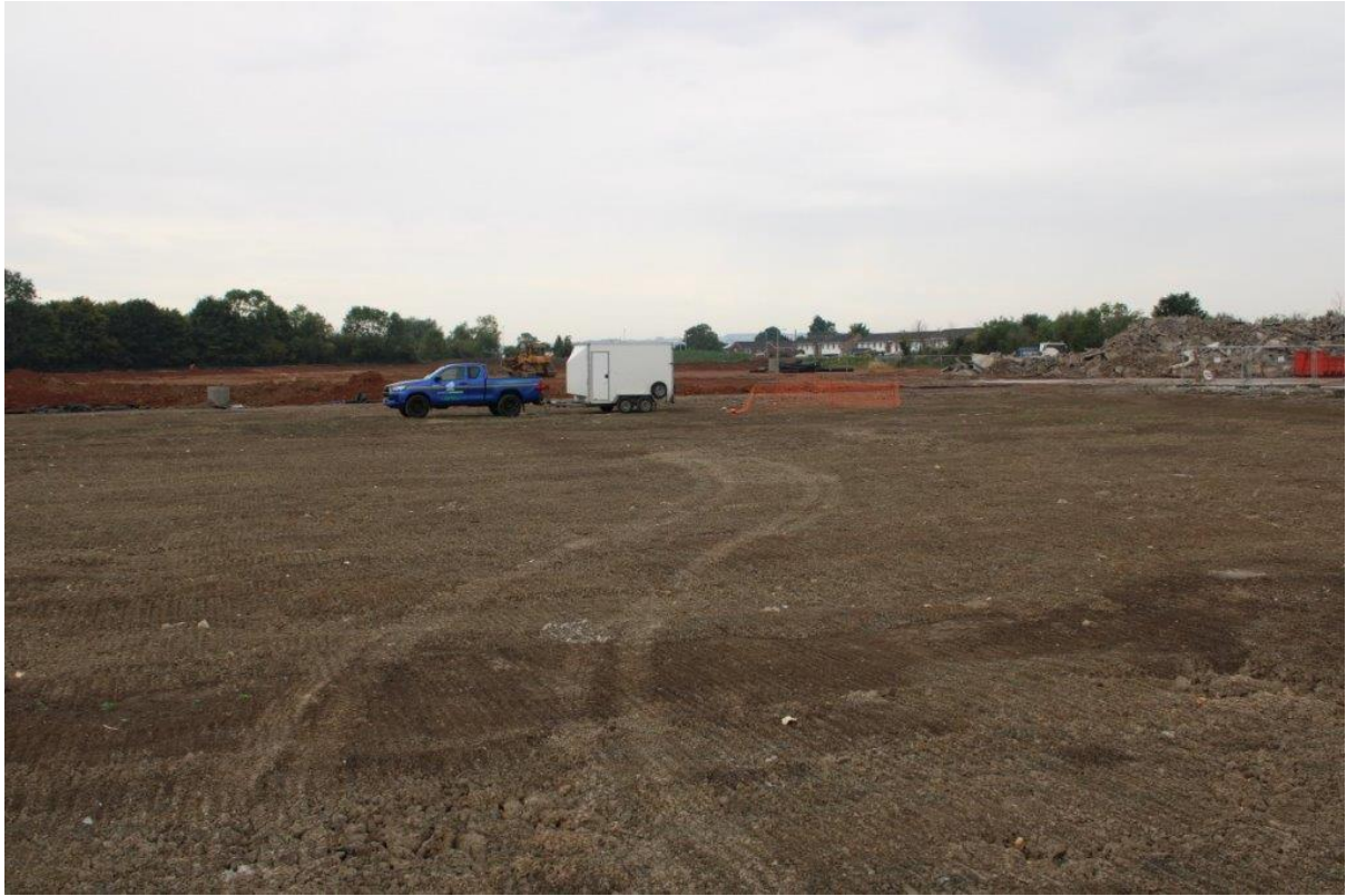
Plate 7: View across site after greenhouse demolition, August 2022, view southwest
