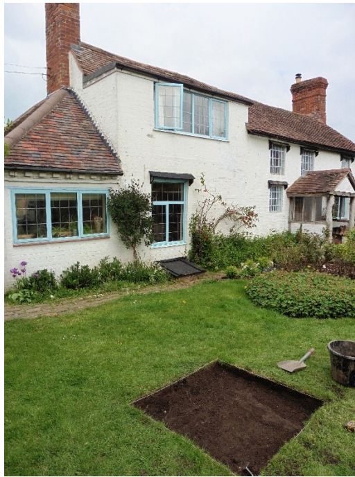
Photo 16. Location of Test Pit 17
