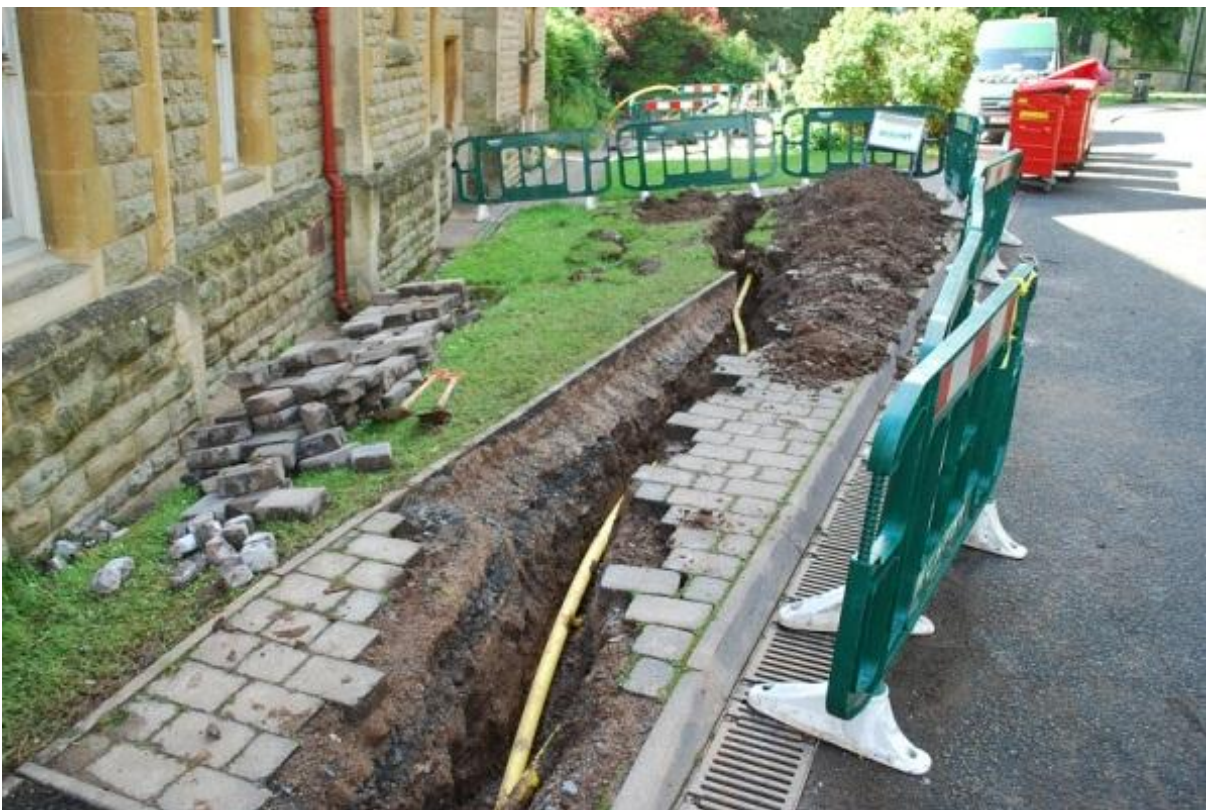
Plate 2 Continuous Trenches 1-3, view south
