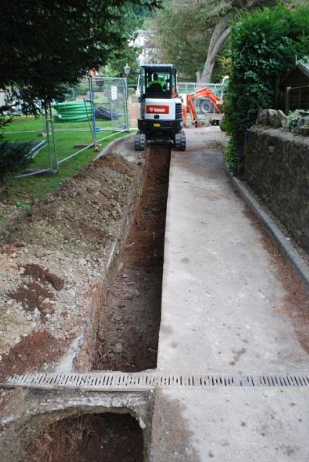
Plate 5 Trench 9, modern surfaces and services, view west
