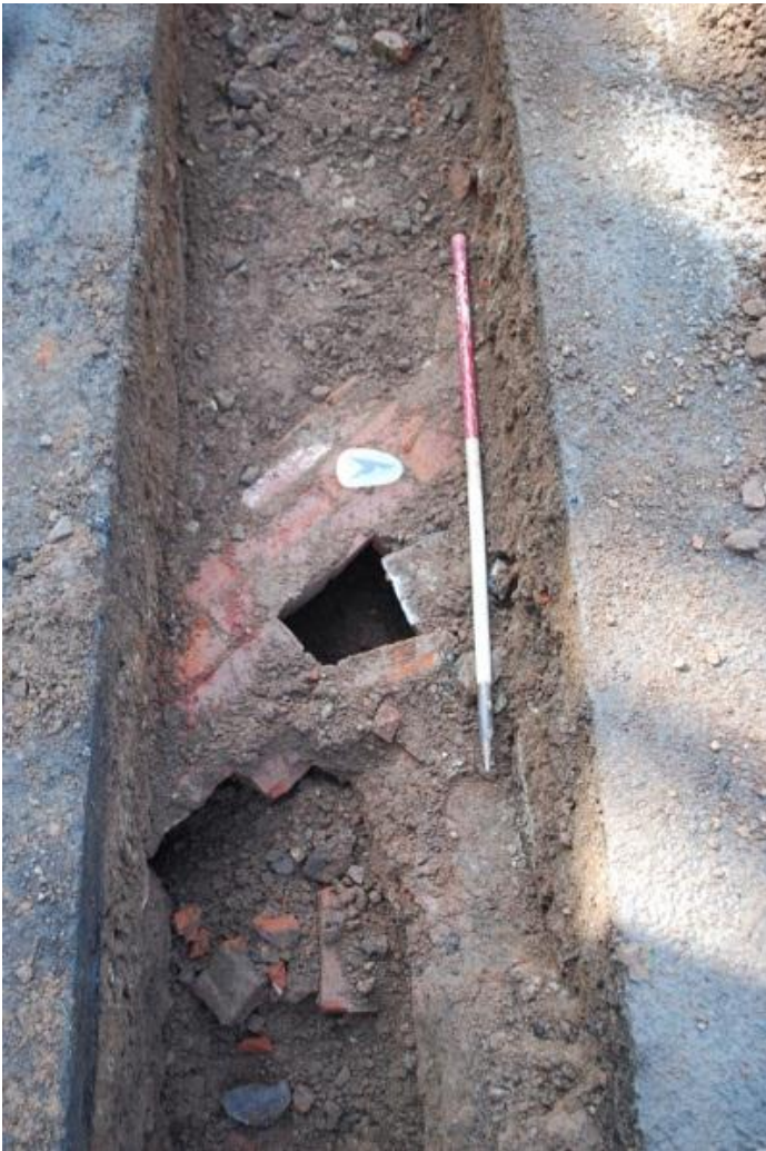
Plate 9 Trench 10, 19 th century brick culvert across trench, view west
