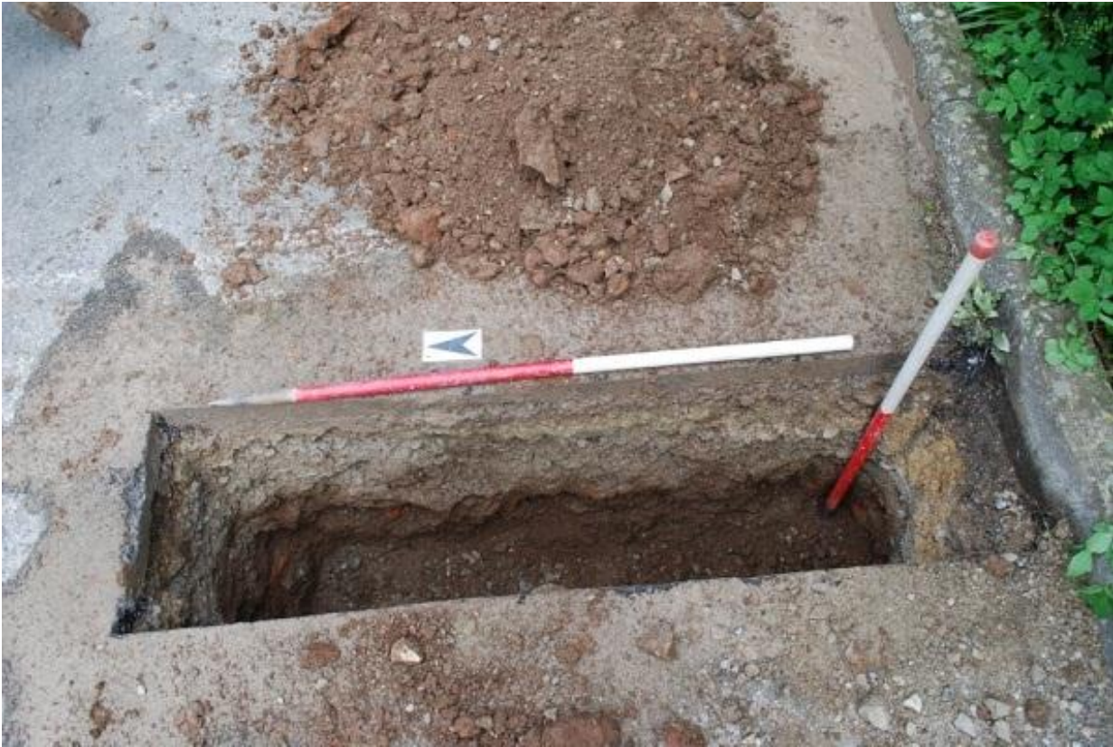
Plate 4 Trench 5 pit for moling machine, view east
