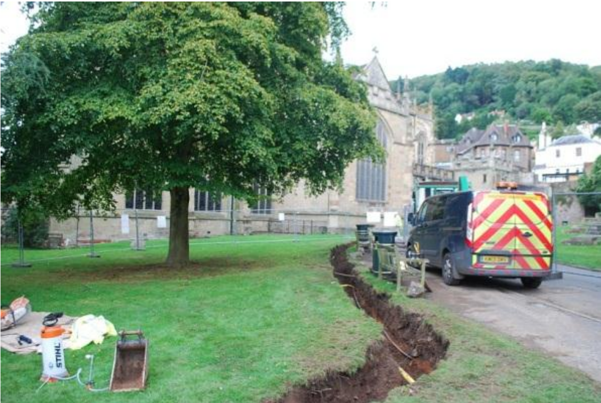
Plate 6 Trench 8 existing water and gas pipes visible, view south-west
