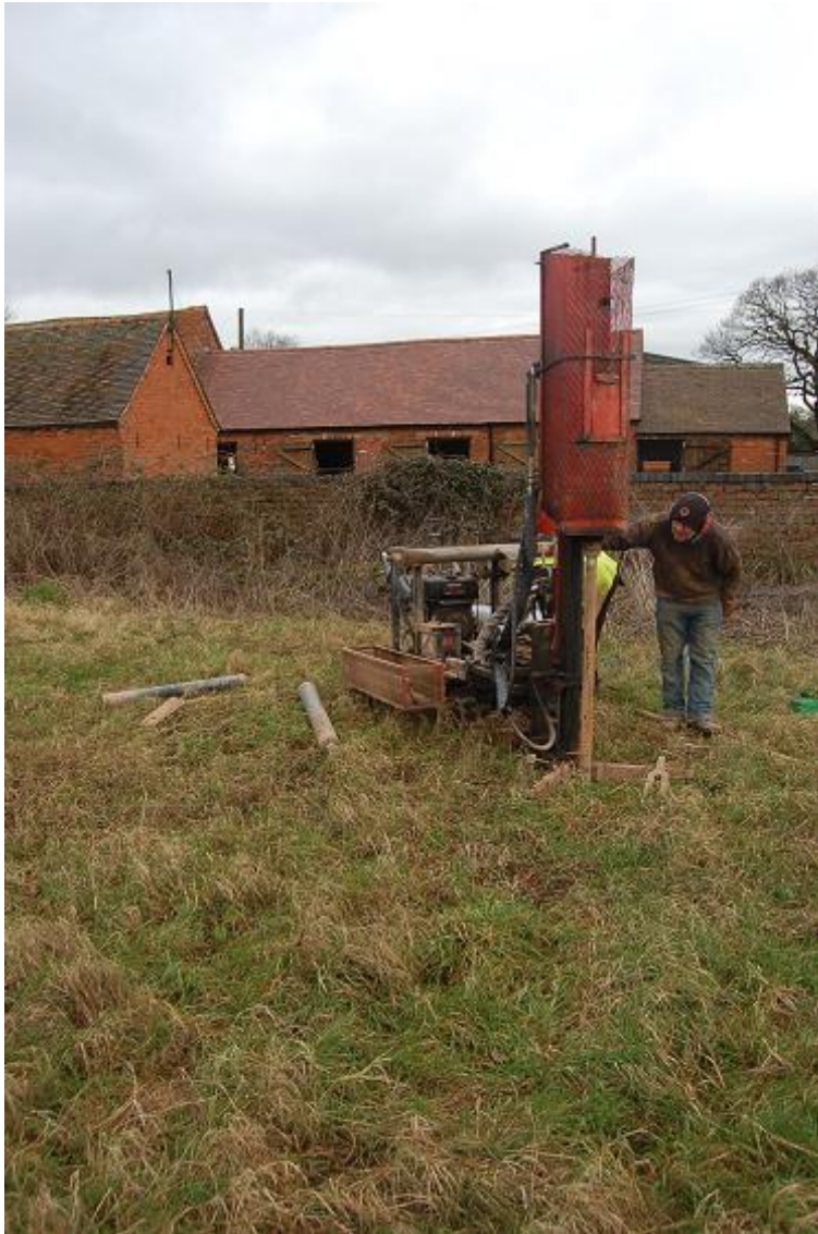
Figure 1 Borehole 1 facing north
