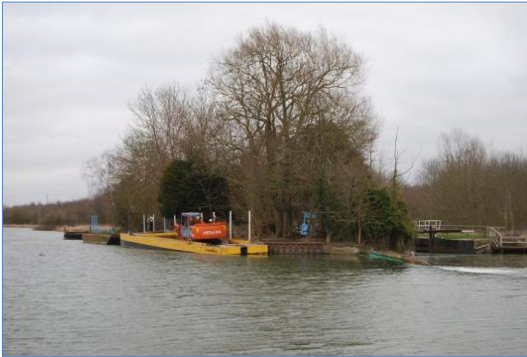
Plate 1, Wyre Mill site location, view north-east
