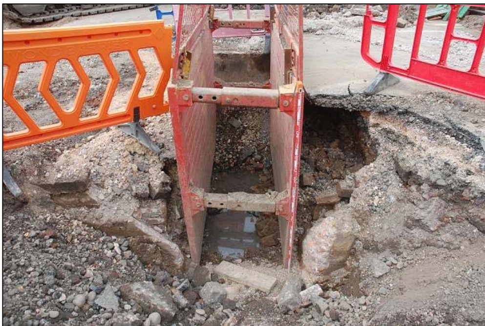
Plate 23 Cellar 41 close up of void and backfill 39 looking south west
