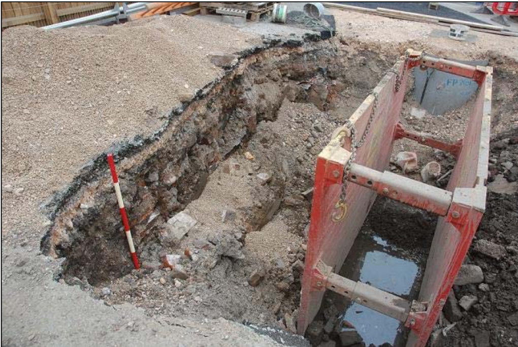
Plate 24 Made ground 42 cut by modern services looking northeast
