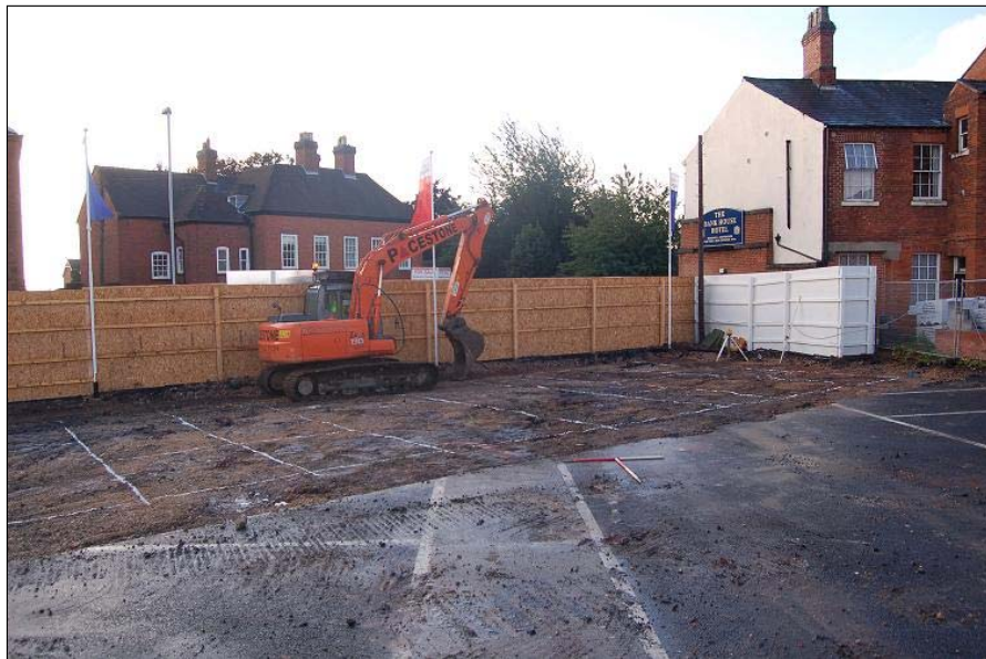
Plate 2 Units 81-84 foundations marked out, looking south east
