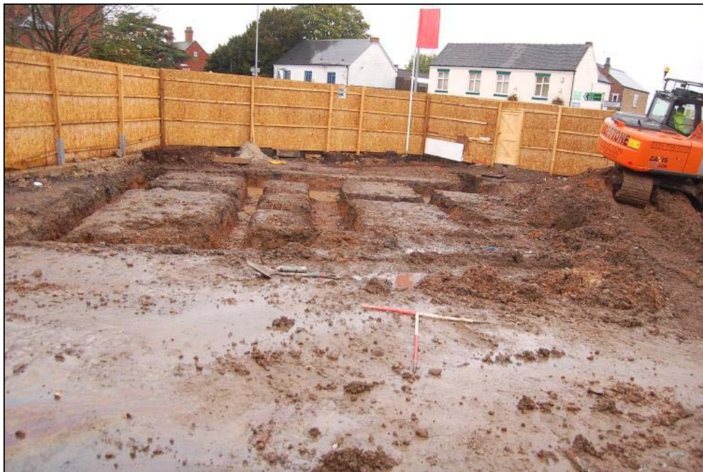
Plate 22 Location of Units 87-88 during excavation looking East
