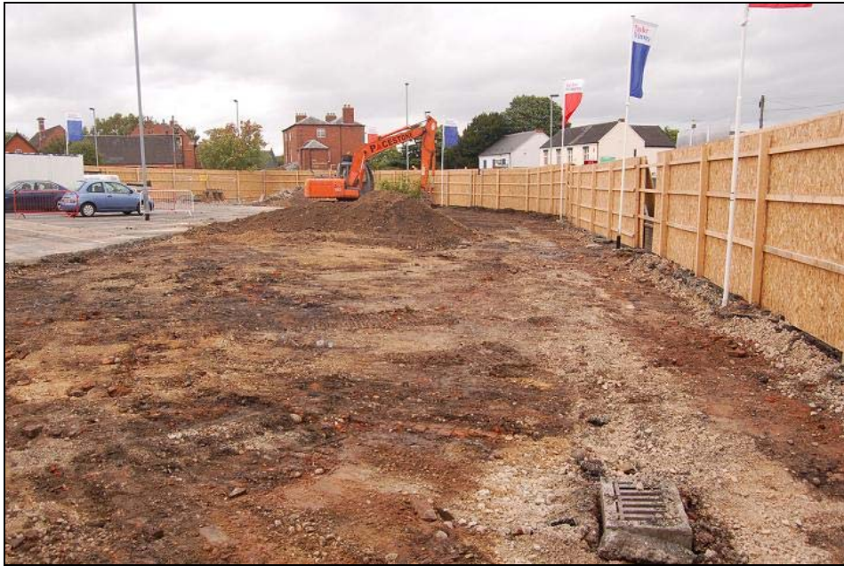
Plate 1 General location shot before work began, looking north
