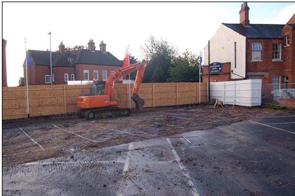
Plate 2 Units 81-84 foundations marked out, looking south east
