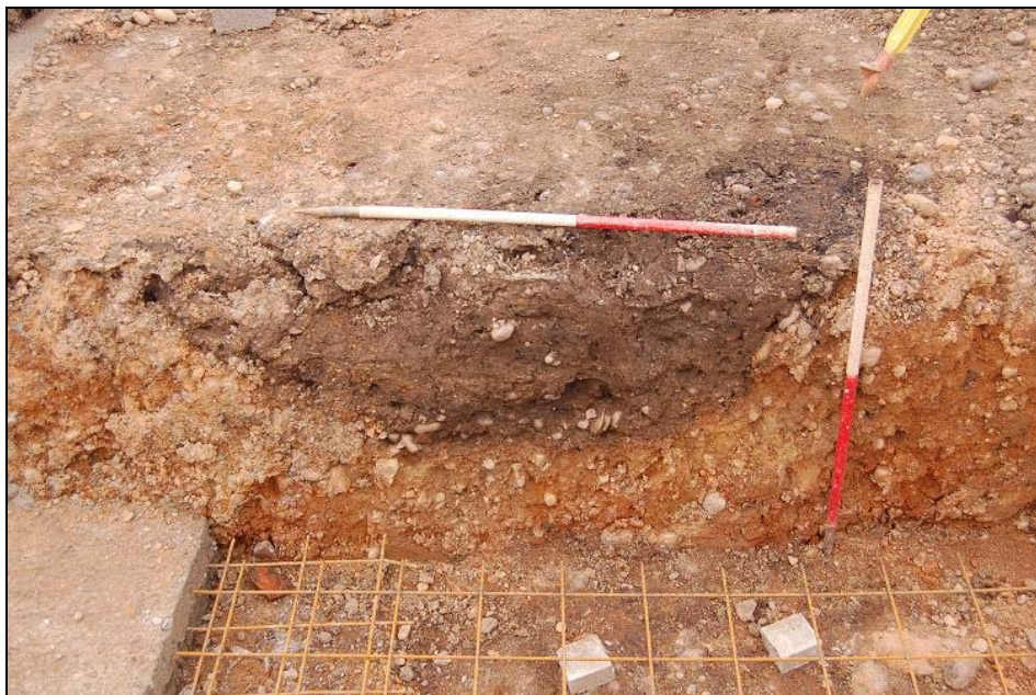
Plate 10 Pit [20] East facing section within Lullington foundations
