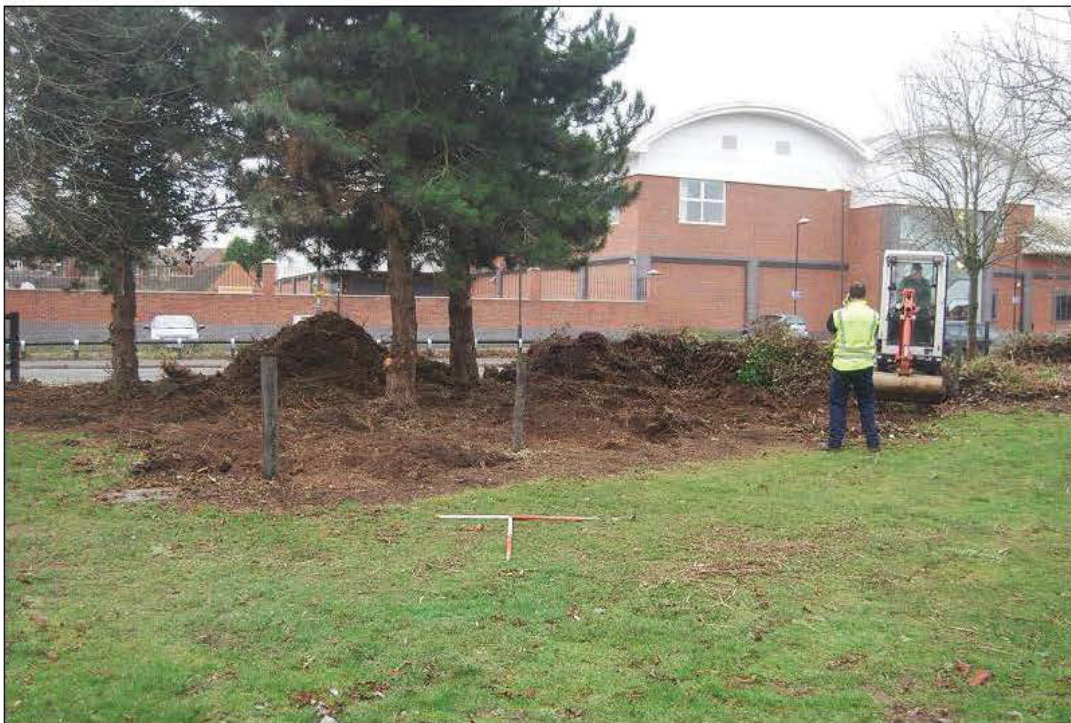
Plate 12: Scrub clearance, Trench 16 in progress, looking south
