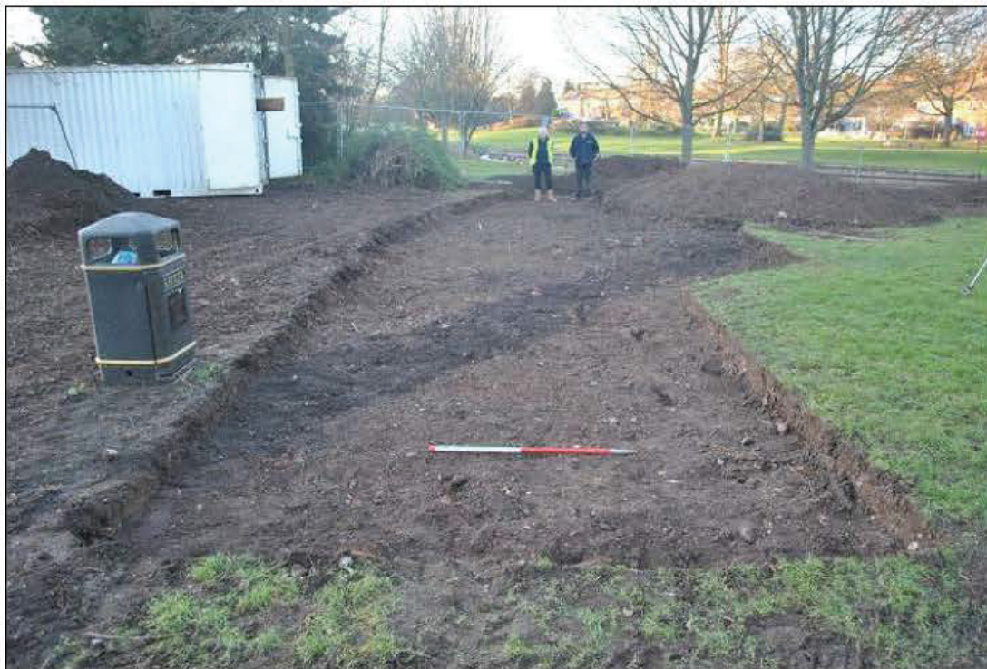
Plate 4: Trench 2, play area, showing modern service trench, looking west
