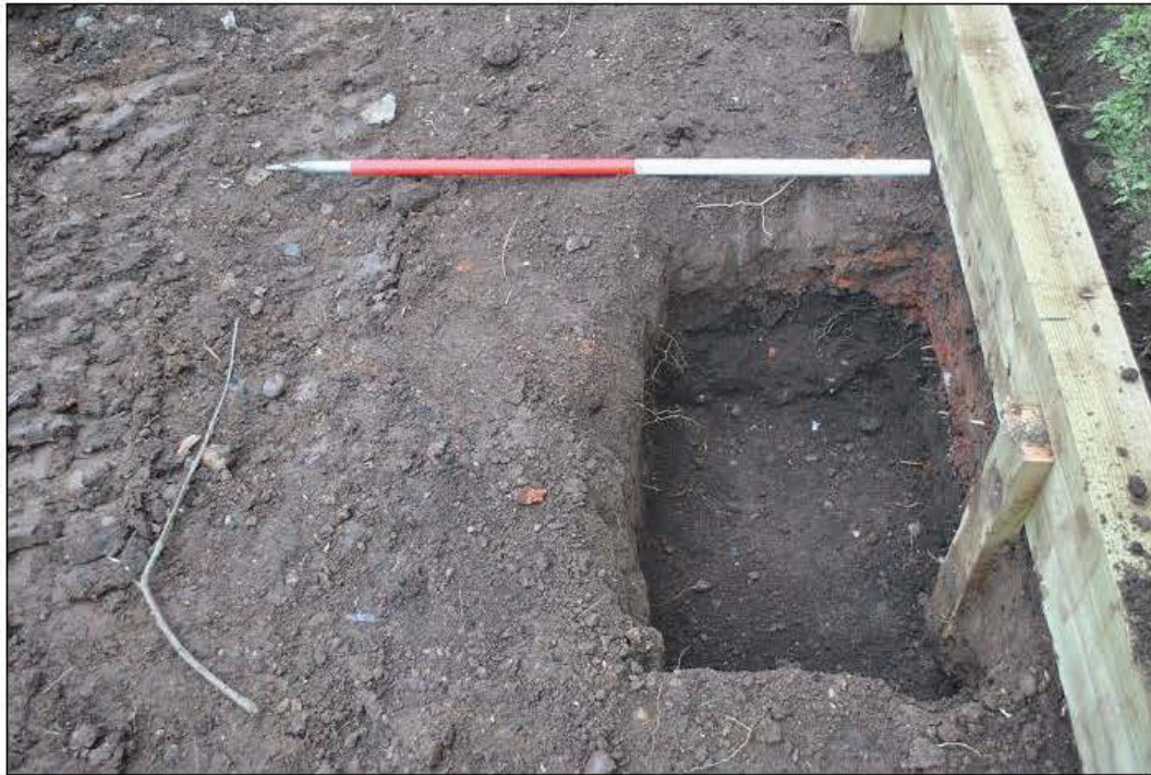
Plate 3: Foundations for swings in Trench 1, play area
