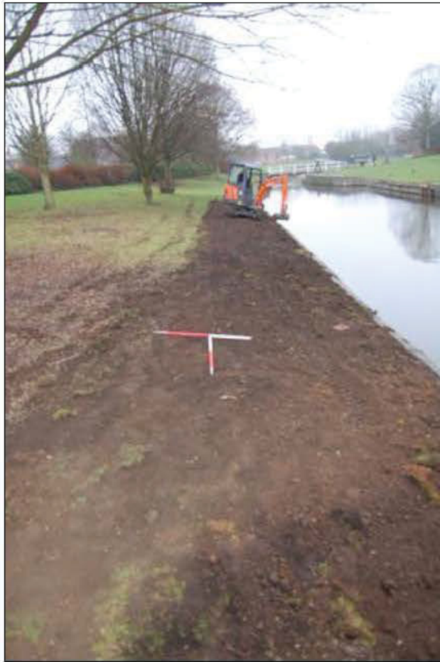
Plate 8: Trench 15, landscaping ground next to canal basin, looking west
