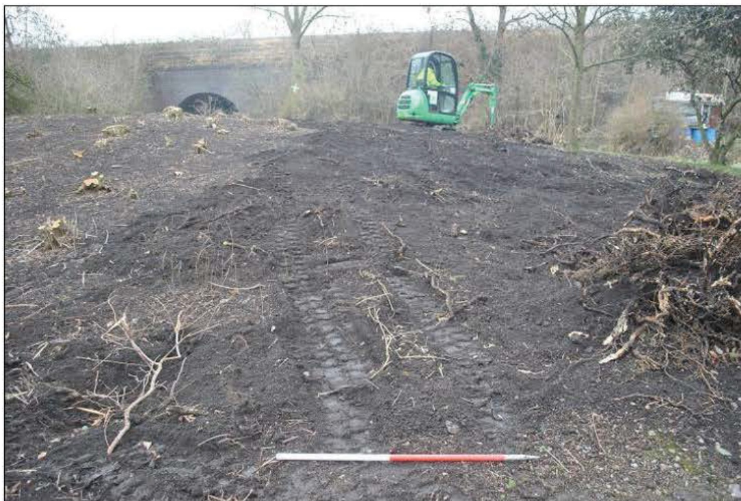
Plate 10: Scrub clearance in Area 6 showing topsoil, looking north-west
