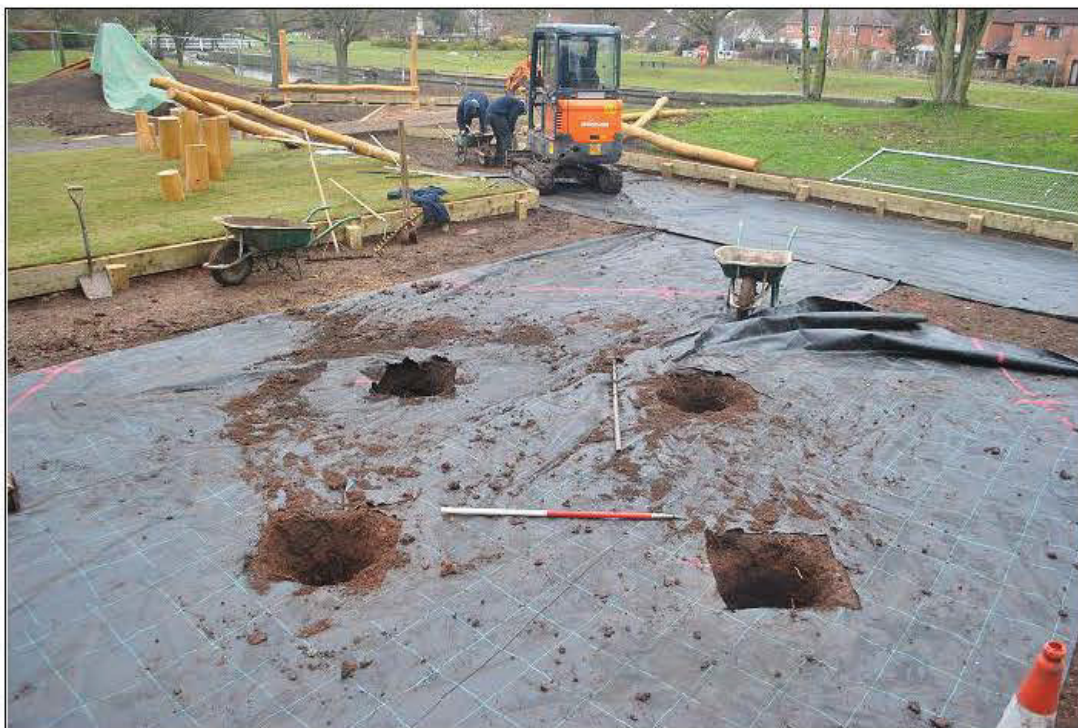
Plate 2: Post holes for climbing frames in Trench 1, play area, looking north-west
