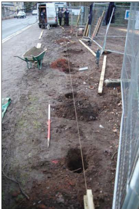
Plate 9: Post holes for fencing facing onto the Saltway (Trench 12) , play area, looking west
