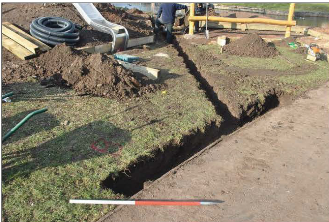
Plate 6: Trench 11, play area drainage channel, looking north-west
