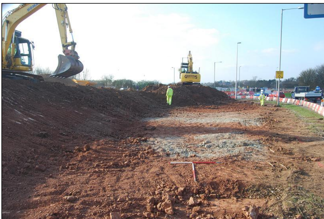
Plate 6 Trench 6 topsoil strip and bank re-grading, looking north-west
