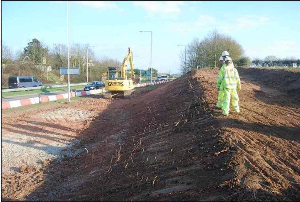
Plate 7 Trench 6 topsoil strip and bank re-grading, looking south-east
