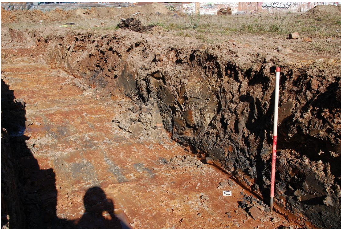
Plate 4; made ground and contaminants in trench 3, facing east, 1m scale
