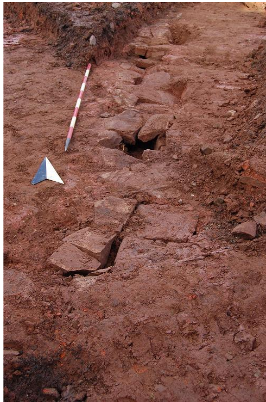
Plate 2, Sandstone culvert 3006 truncated in foreground by modern service 3005; looking northeast; scale 2m
