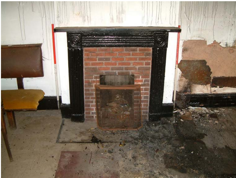
Plate 20. The public house, east wing, fireplace in south wall, view south
