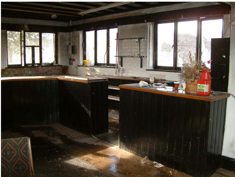
Plate 24. The public house, west wing, room space, view north-west
