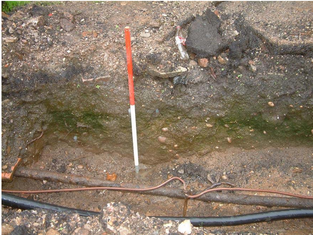
Plate 47. Trench associated with electrical sub-station within car park on west side of site, south section, view west-south-west
