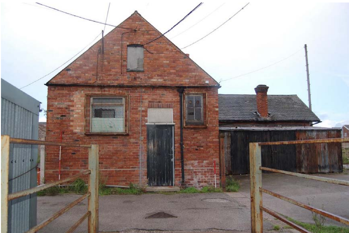
Plate 14. The public house, west wing, south elevation/gable end, view north
