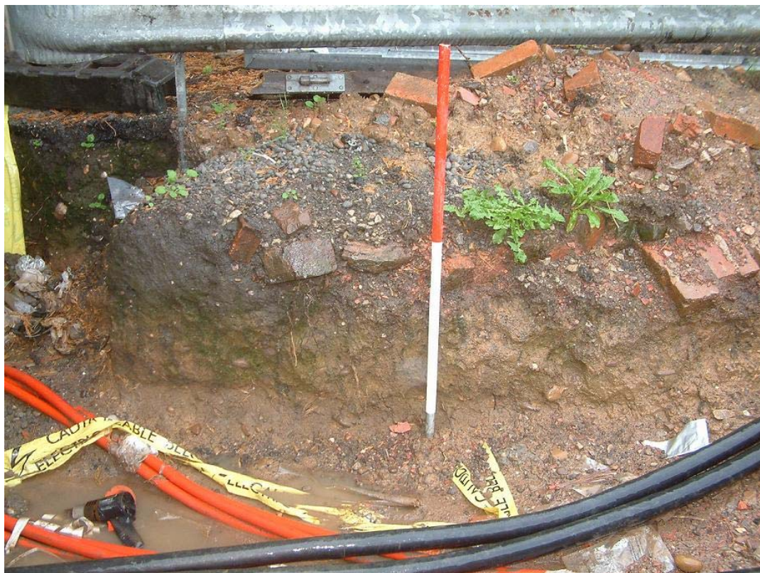
Plate 48. Trench associated with electrical sub-station within car park on west side of site, north section, view west-south-west
