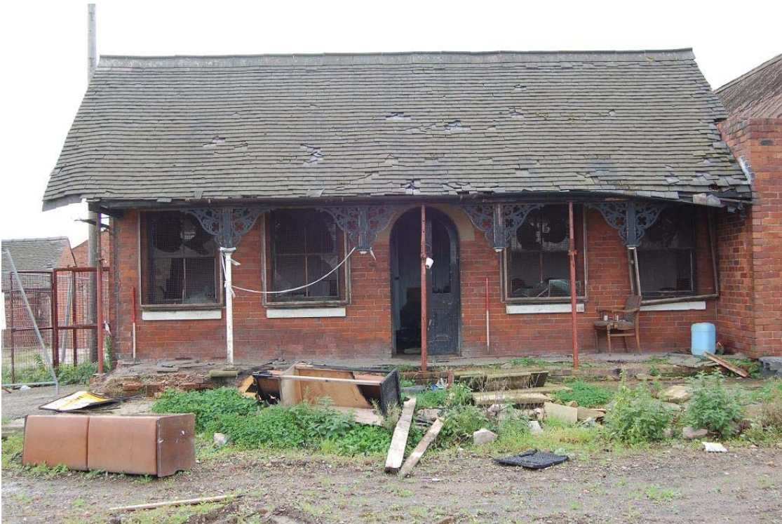
Plate 2. The public house, east wing, north elevation and porch, view south
