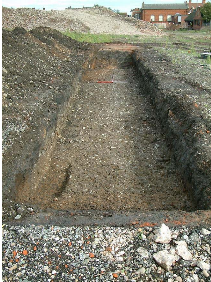
Plate 38. Trench 9, general view east
