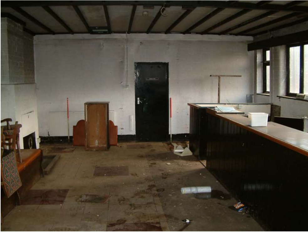
Plate 27. The public house, west wing, room space and partition, view south
