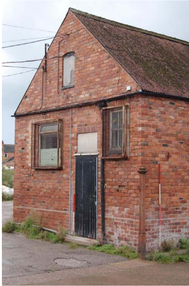
Plate 13. The public house, west wing, south elevation/gable end
