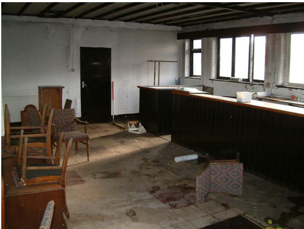
Plate 26. The public house, west wing, room space, view south-south-west
