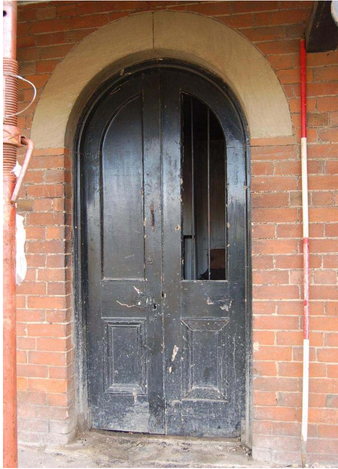
Plate 5. The public house, east wing, entrance under porch, view south-south-east
