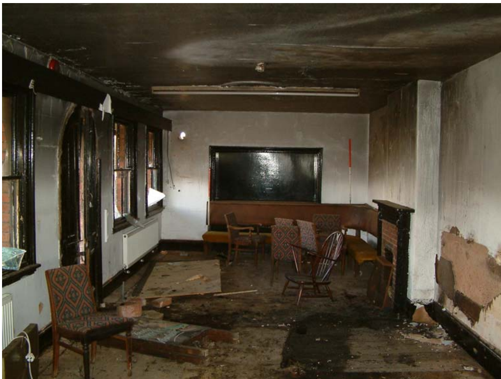
Plate 18. The public house, east wing, room space, view east
