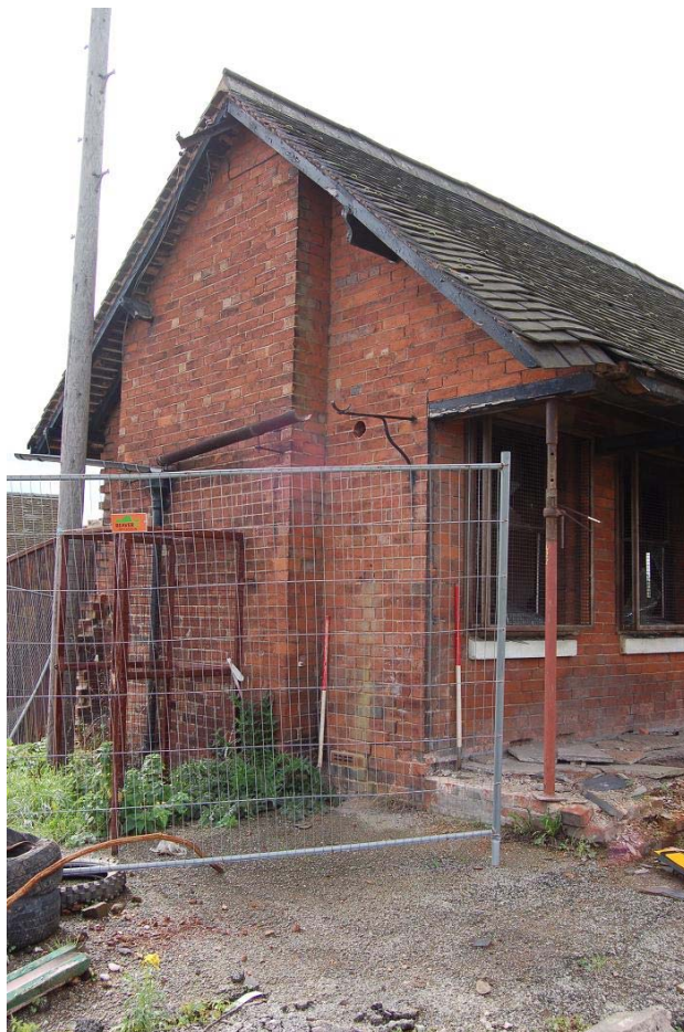
Plate 8. The public house, east wing, east elevation/gable elevation, view south-west
