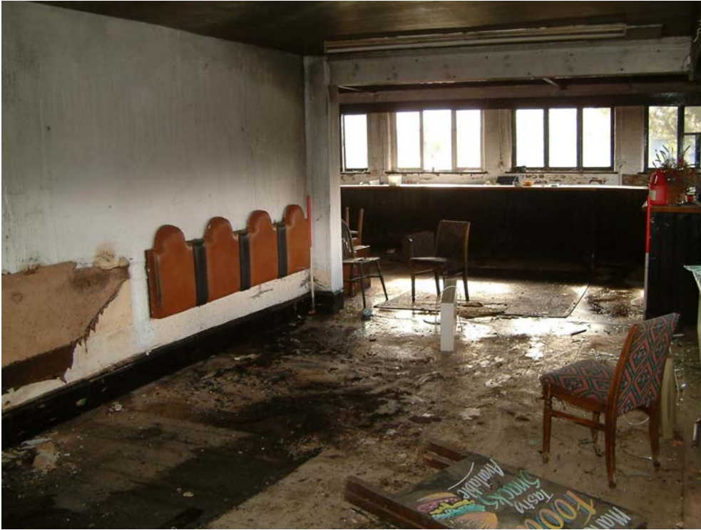
Plate 21. The public house, east wing, room space, view west-south-west
