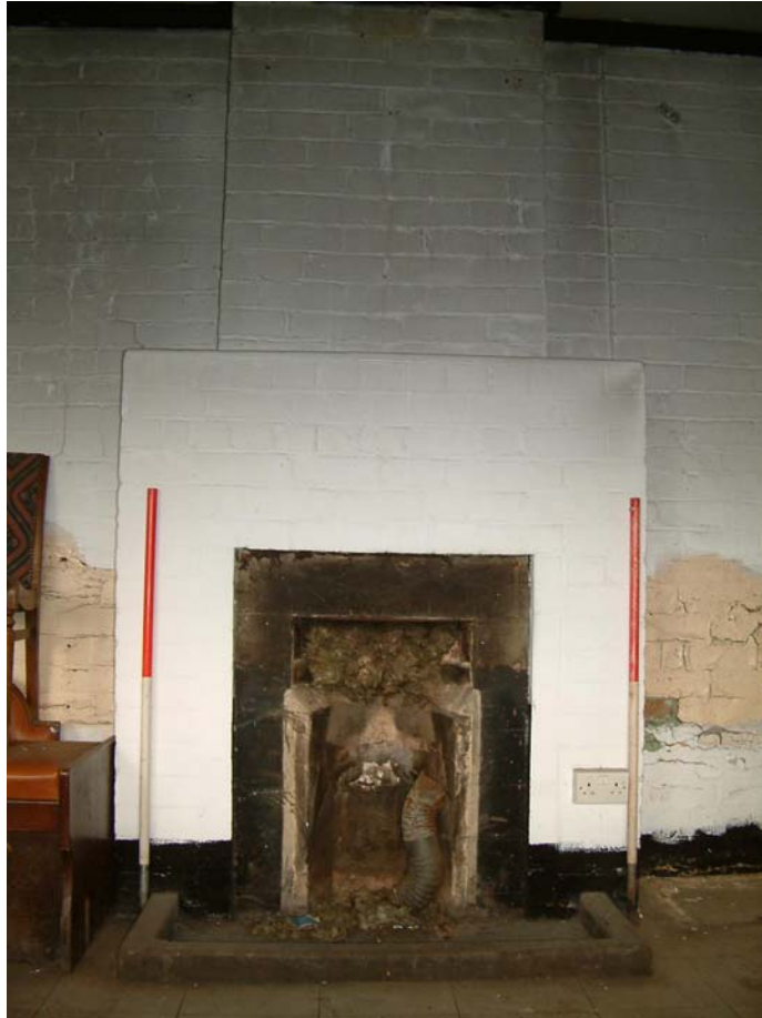
Plate 29. The public house, west wing, fireplace in east wall, view east
