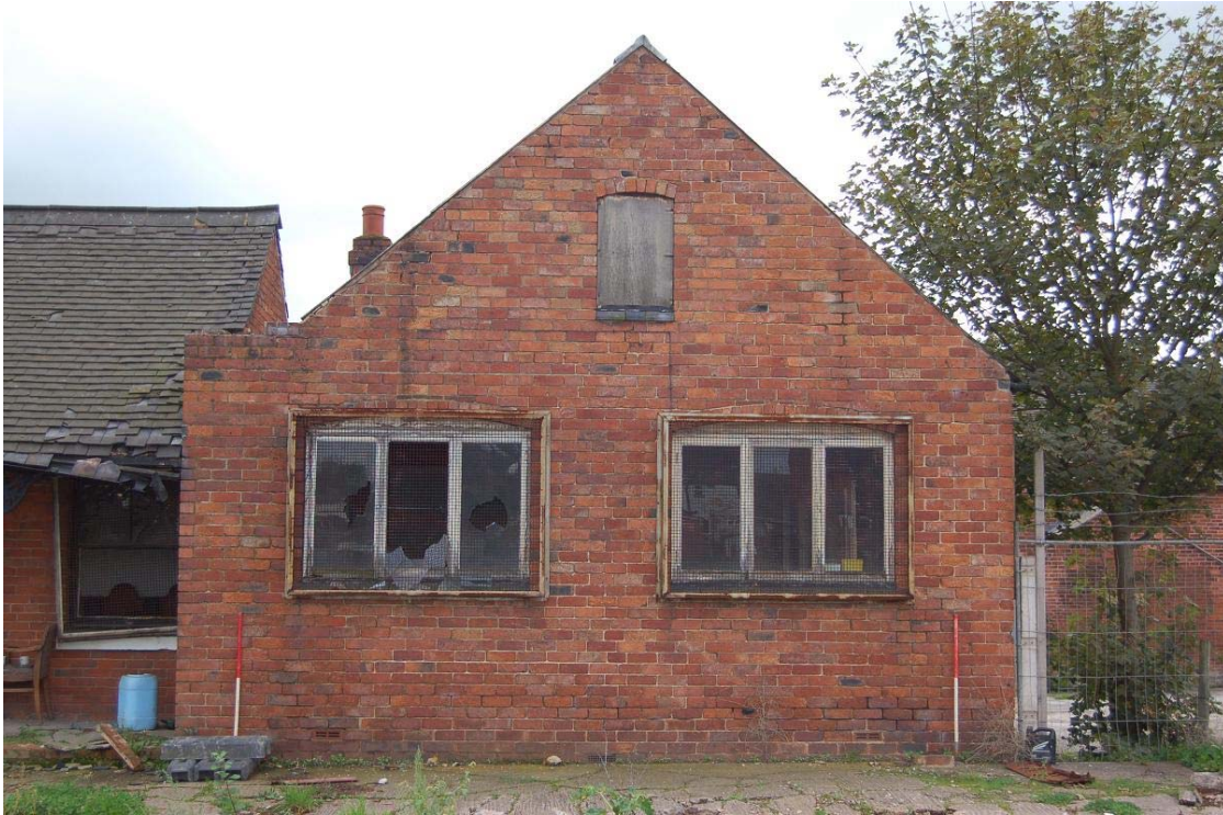
Plate 17. The public house, west wing, north elevation/gable end, view south
