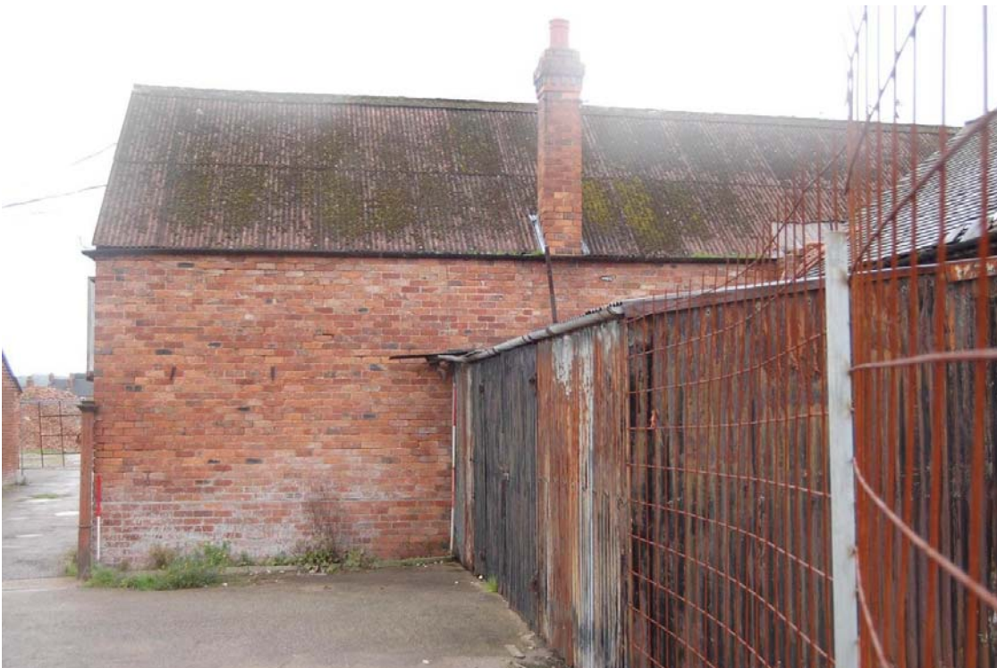
Plate 12. The public house, west wing, east elevation, view west
