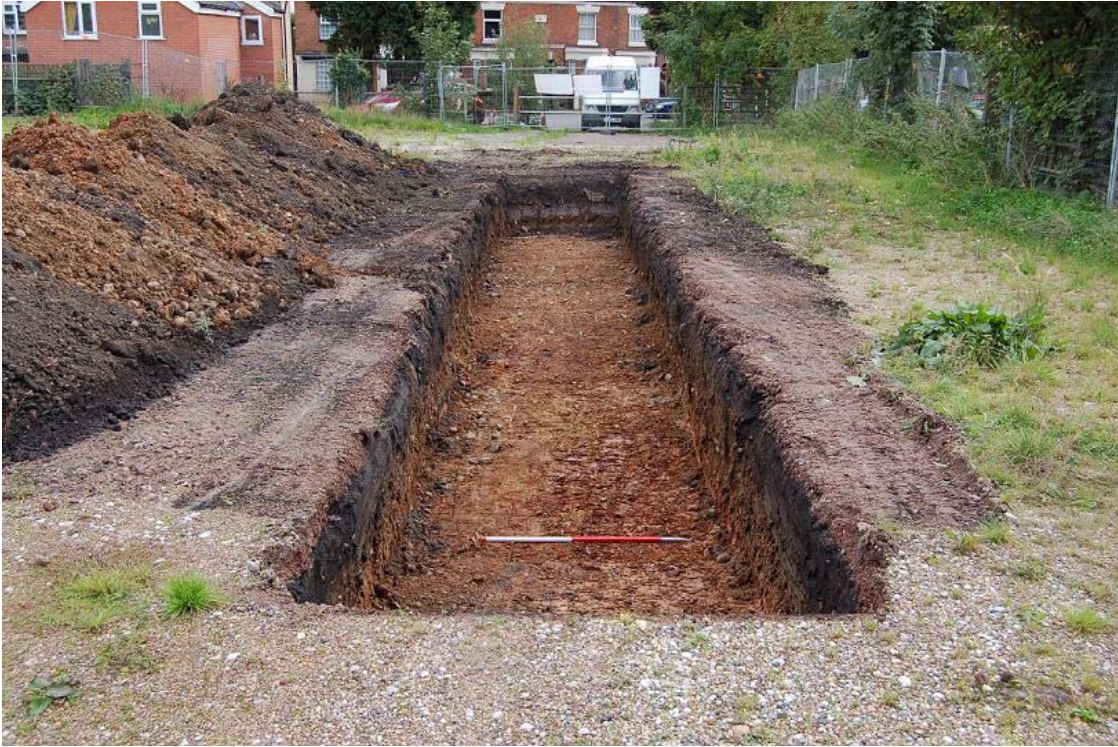
Plate 45. Trench 15, general view south-south-east
