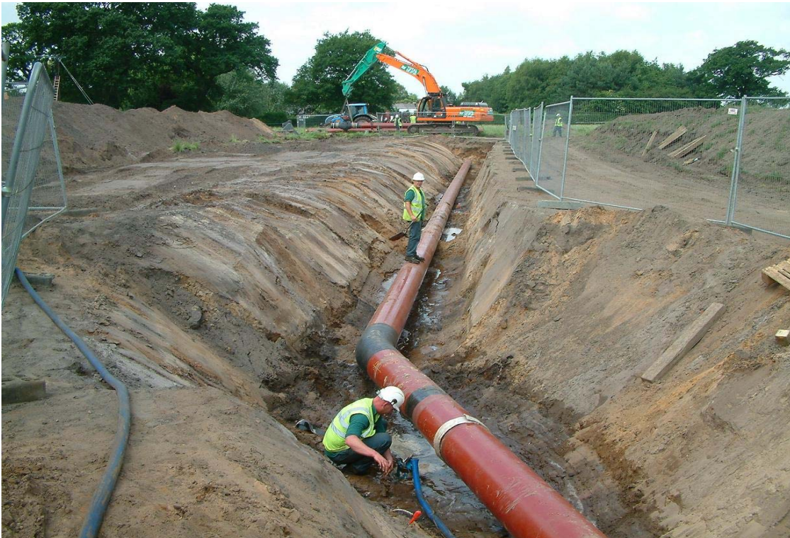
Plate 14: The pipe trench and pipe in field 5, Looking West
