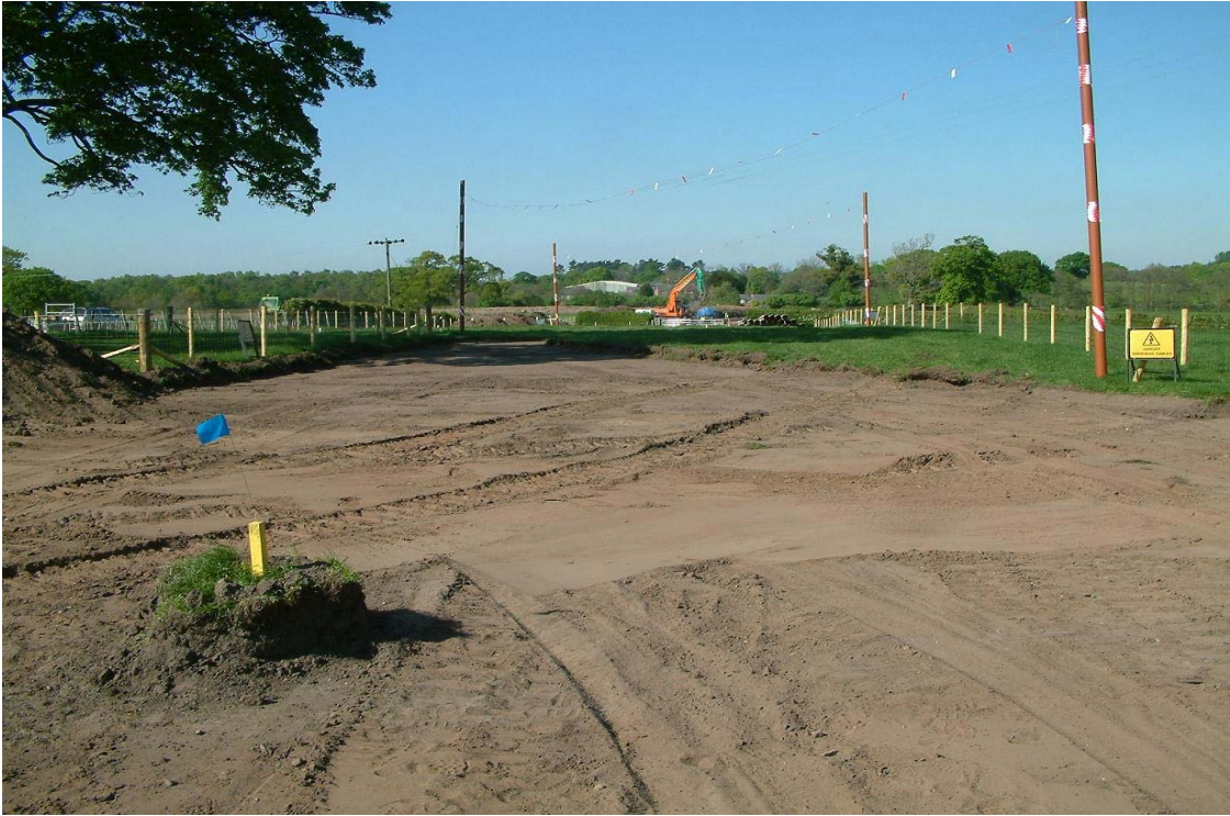
Plate 5: The stripped easement in field 3, looking NE
