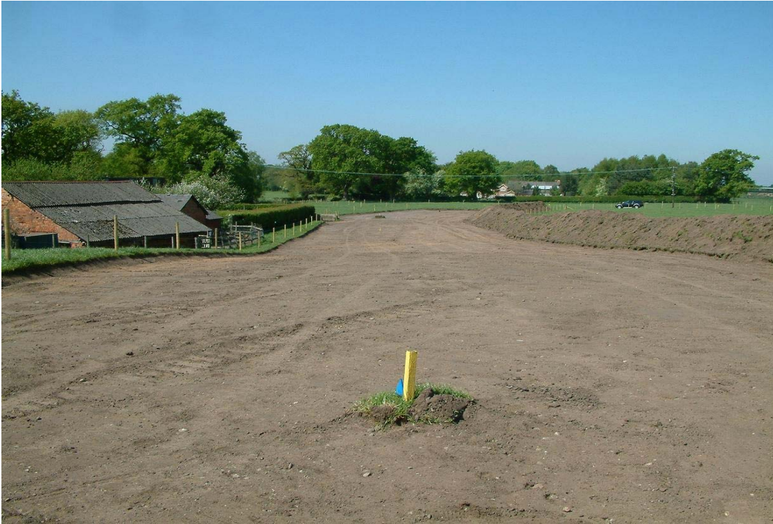
Plate 13: The stripped easement in field 5, looking West
