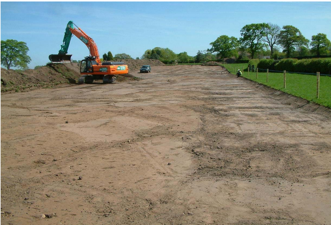
Plate 8: The easement in field 4, looking East
