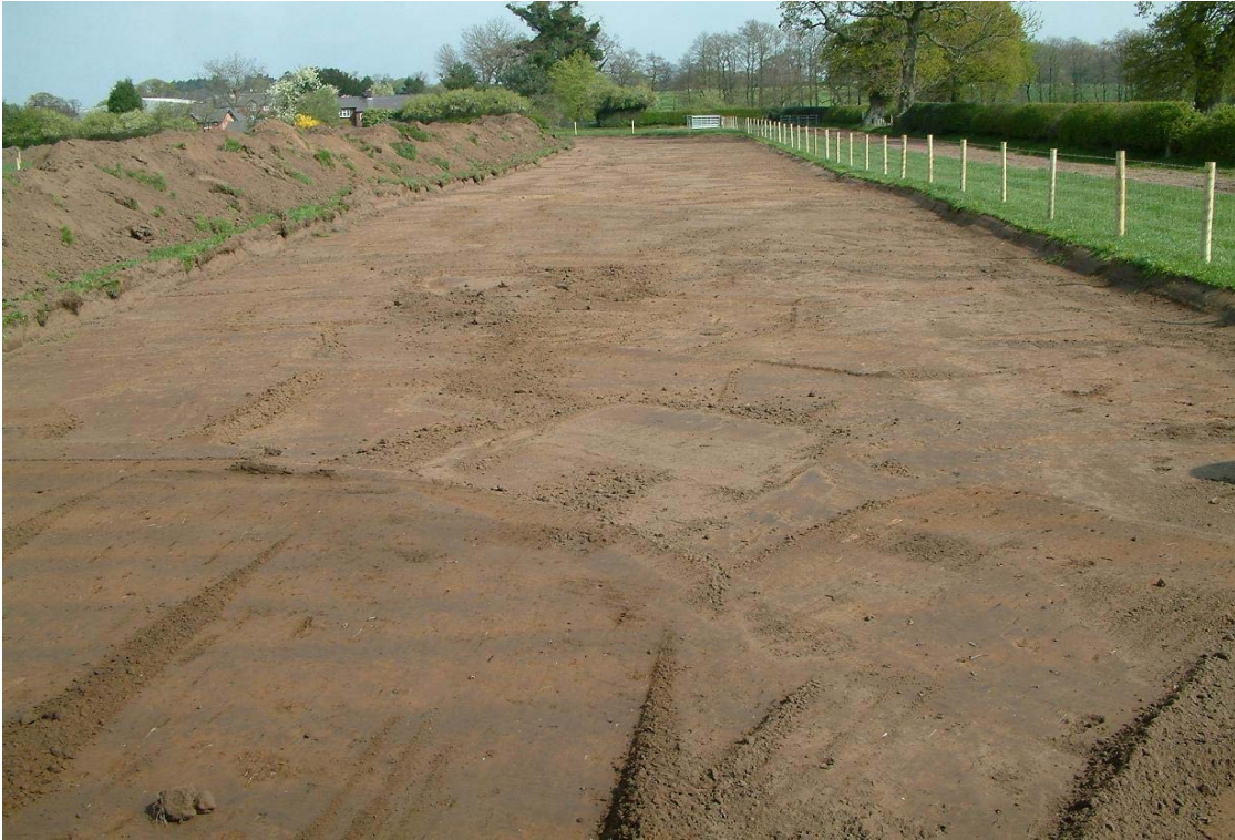
Plate 3: The stripped easement in field 2, looking NE
