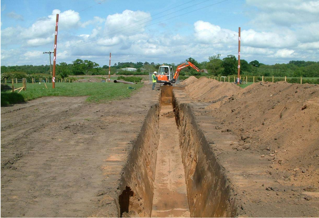
Plate 7: Excavation of the pipe trench in field 3, looking NE
