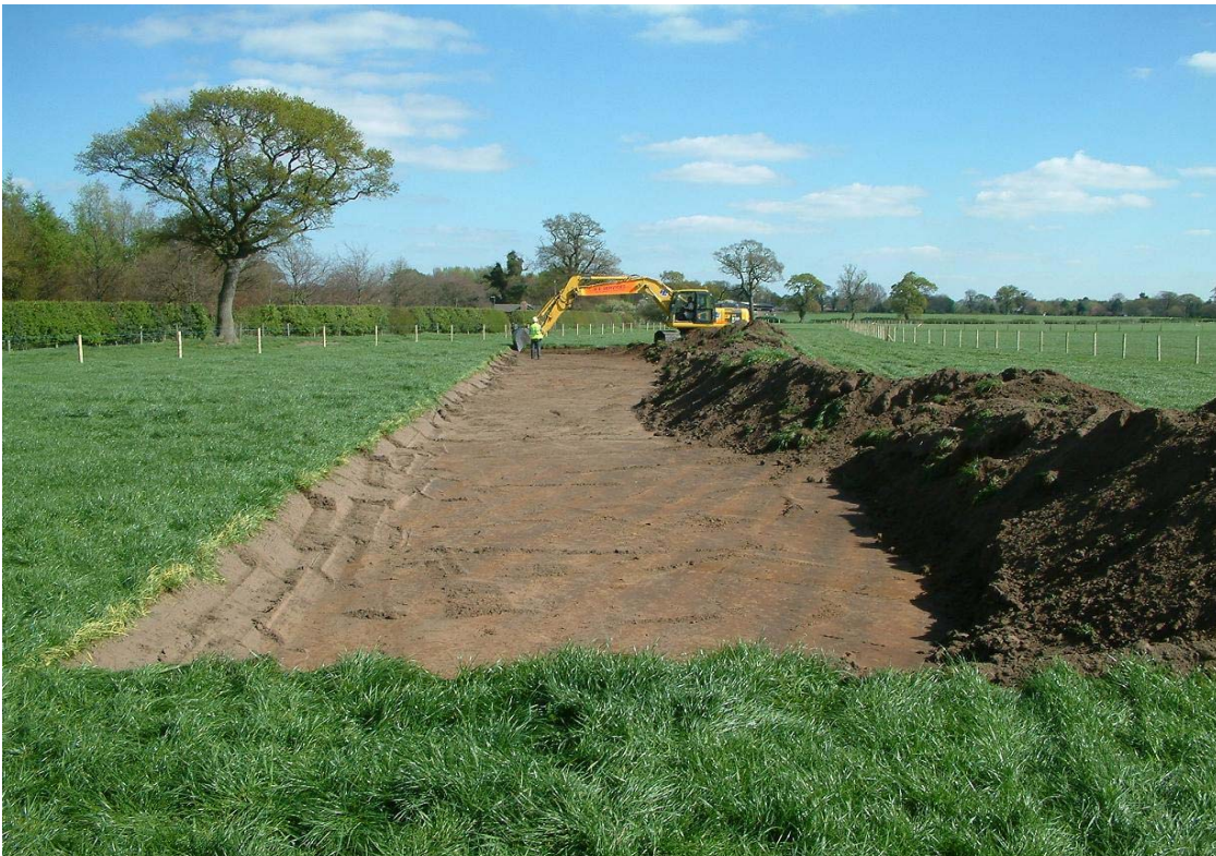
Plate 2: Stripping the easement in field 1, looking SE
