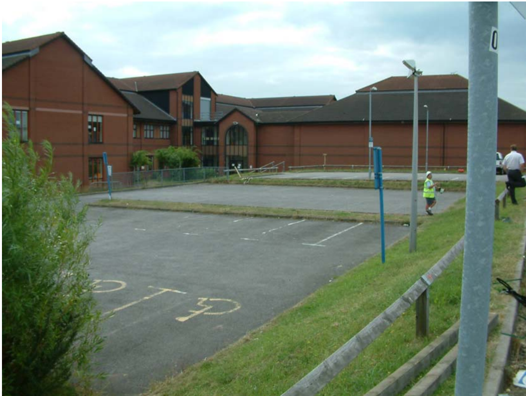
Plate 1: Pre-excavation, view east-south-east
