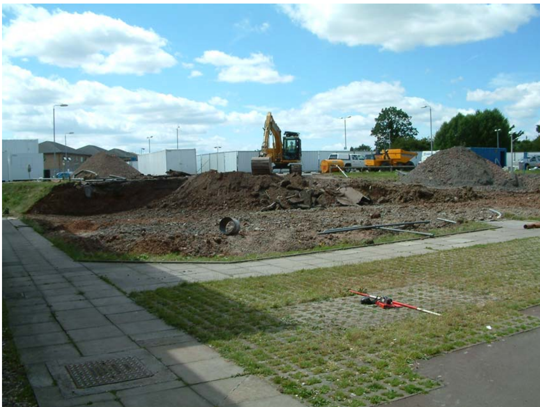
Plate 2: Excavation in progress, view north-west
