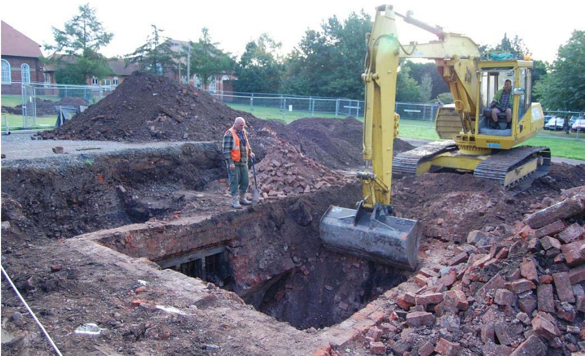
Plate 16, Trench 10, general view east of work in progress
