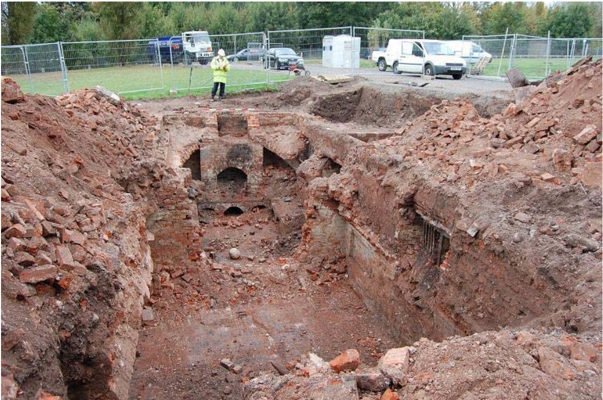
Plate 17, Trench 10, general view northwest of northeast compartments
