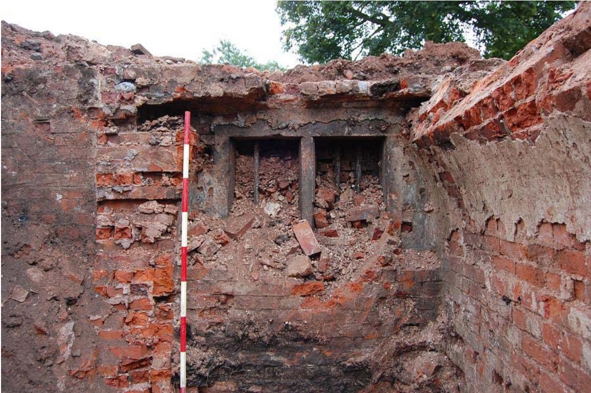
Plate 26, Trench 10, view southeast of window to light-well at southeast end of cellar corridor
