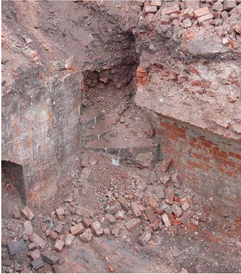
Plate 22, Trench 10, detail of stone spiral staircase in south corner of east compartment, view south
