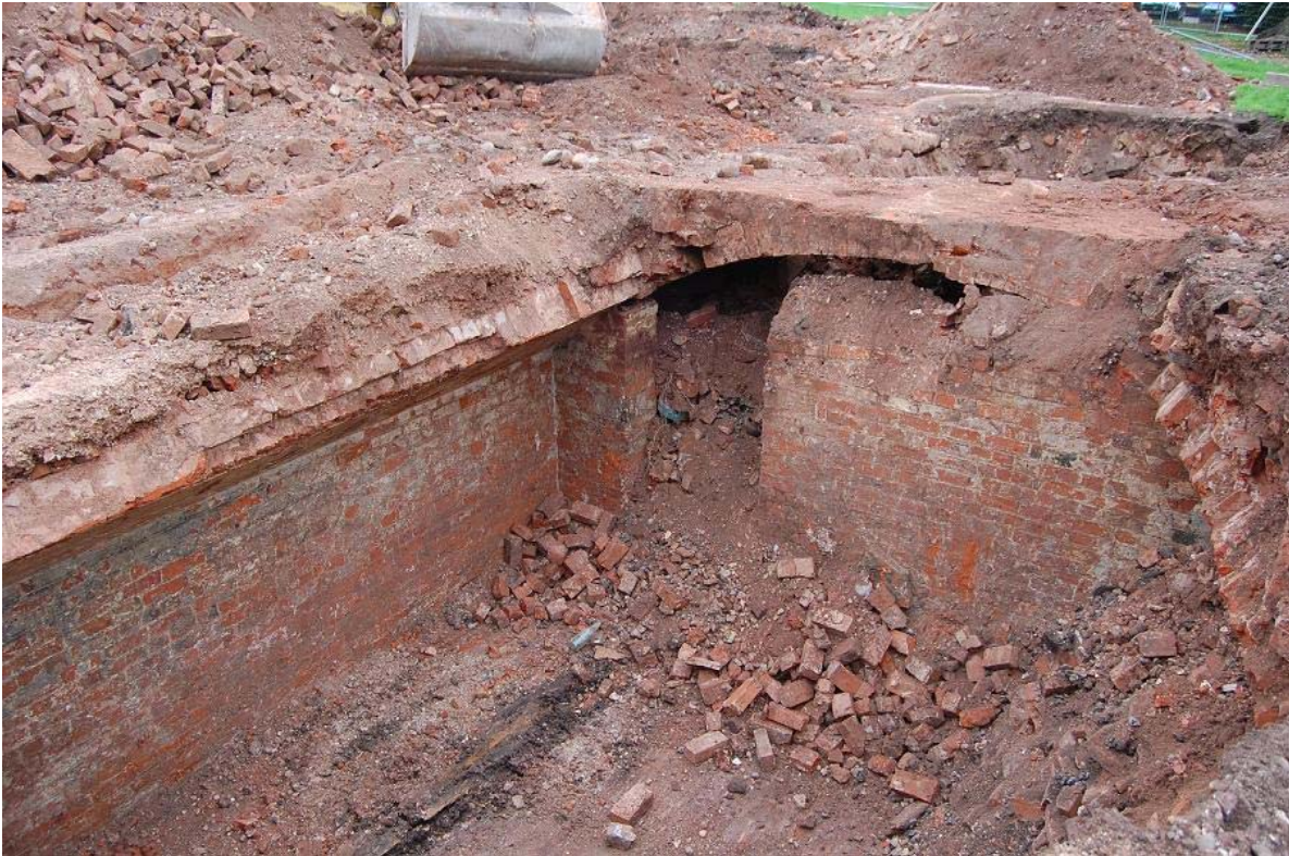
Plate 27, Trench 10, general view east of southwest compartments
