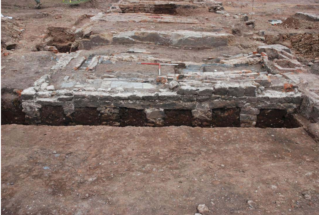
Plate 9: Detail of the sandstone piers supporting wall 1052. Scales at 2m, facing north-west.
