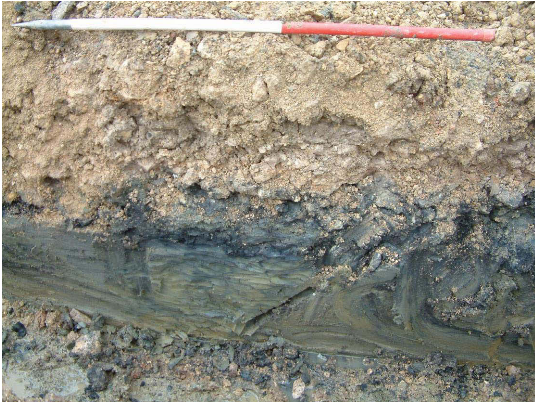
Plate1: Barn C foundation: Trench 1, east section
