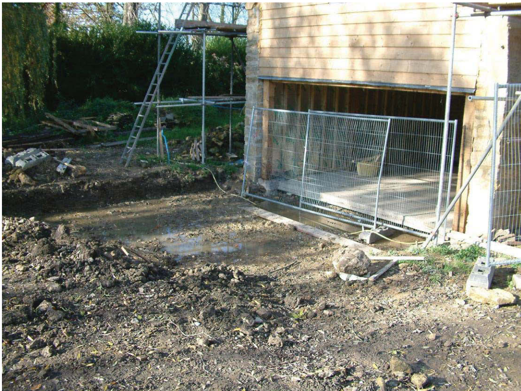
Plate 4: Farmhouse patio strip: Area 3, view north-west
