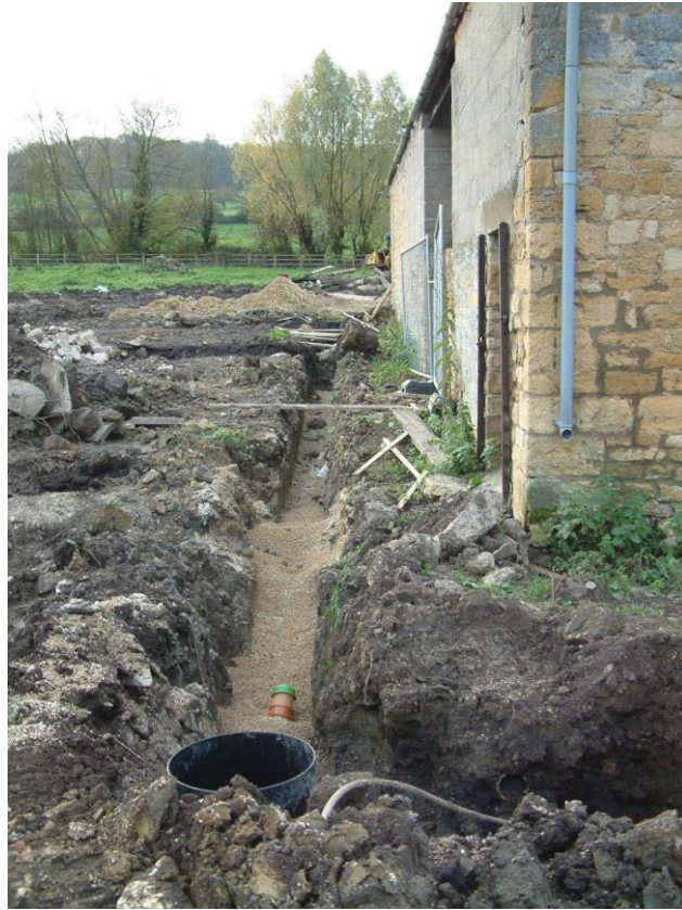
Plate 7: Barn A service: Trench 5, east of barn, view south
