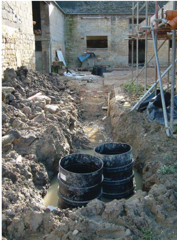
Plate 6: Barn A service: Trench 5, west of barn, view south
