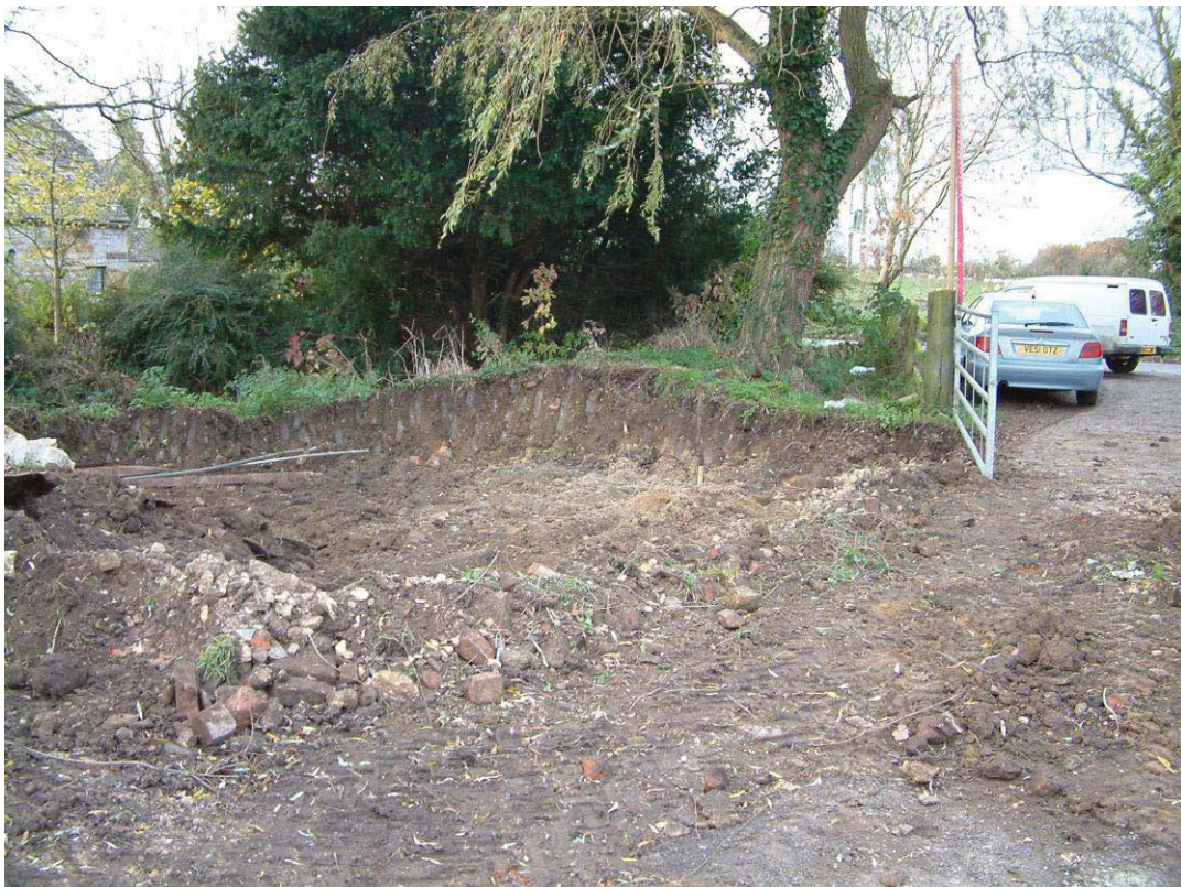
Plate 9: Car park strip: Area 8, view south-west
