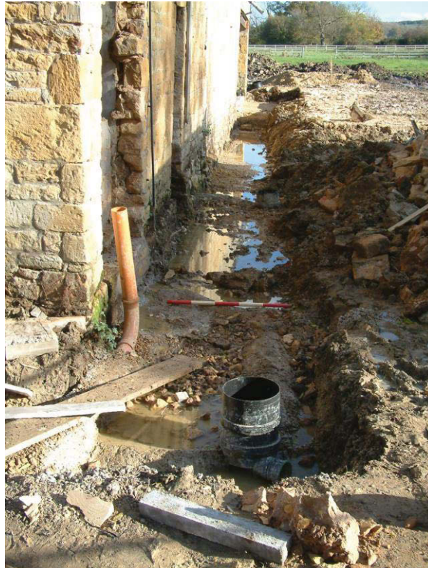
Plate 5: Barn B service: Trench 4, south of barn, view east
