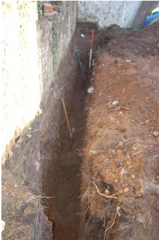
Plate 7: General shot of North Trench, view east
