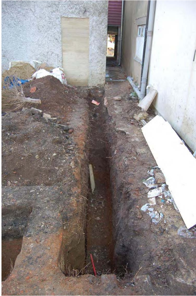
Plate 8: General shot of Southern trench, view east
