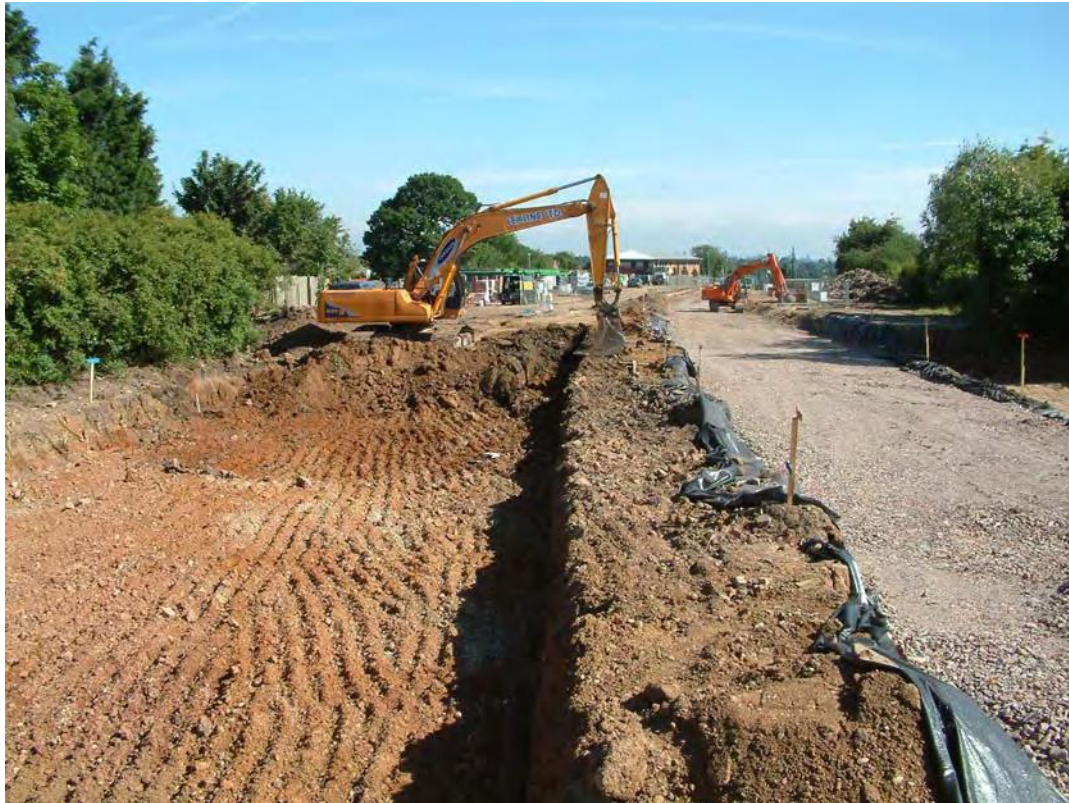
Plate 1: General view of excavations, 8 th August 2005
