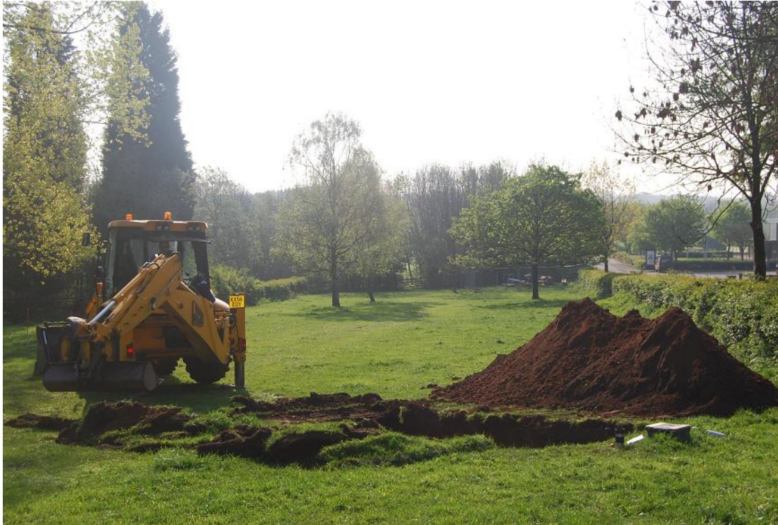
Plate 1 Trench 4 excavation with location of Trench 3 in the background. View south-east
