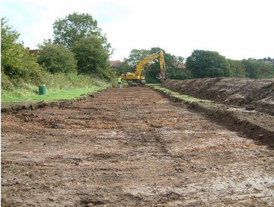
Plate 2: Area at south of access road, facing north east
