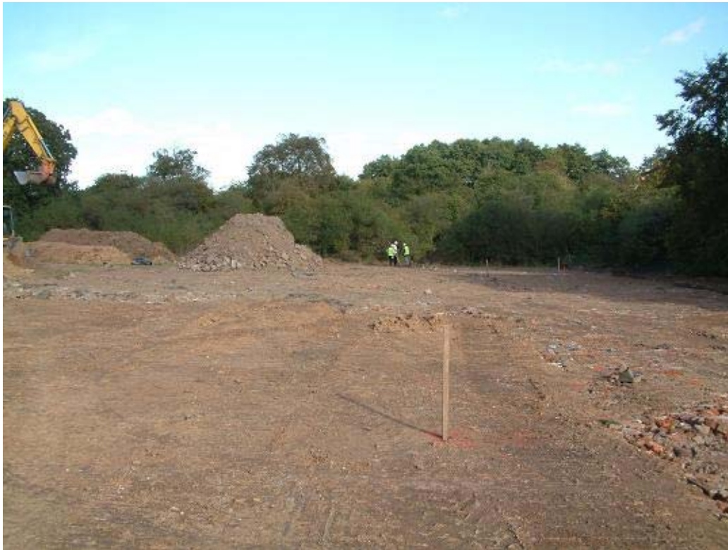
Plate 5: General shot of Site after topsoil strip, facing east
