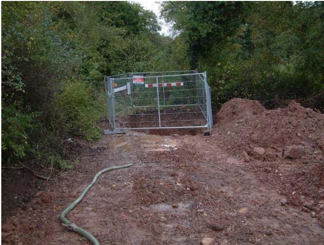
Plate 7: General shot of manhole F1, facing south east
