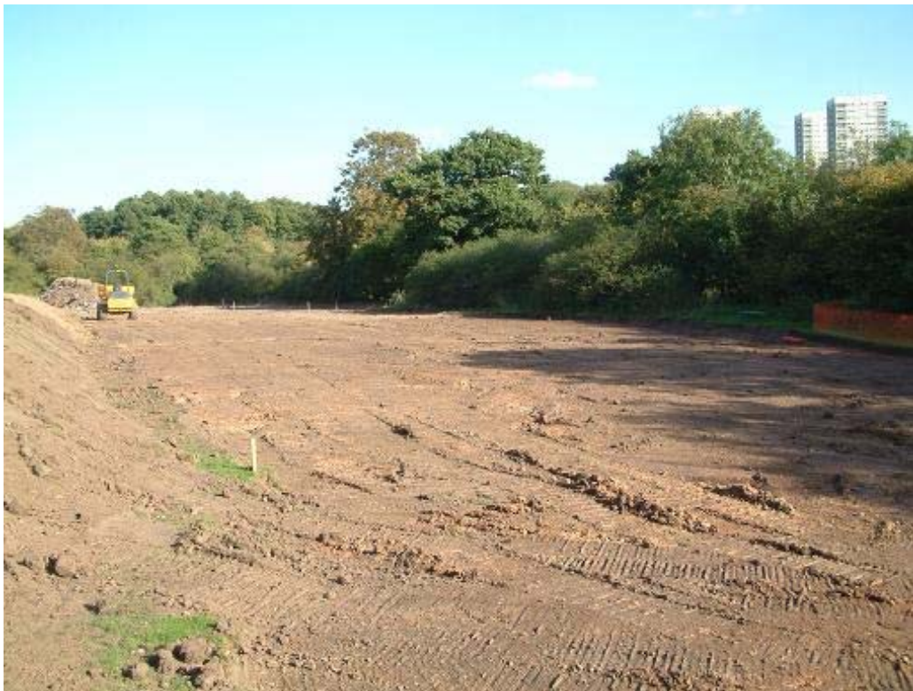
Plate 4: General shot of Site after topsoil strip, facing east
