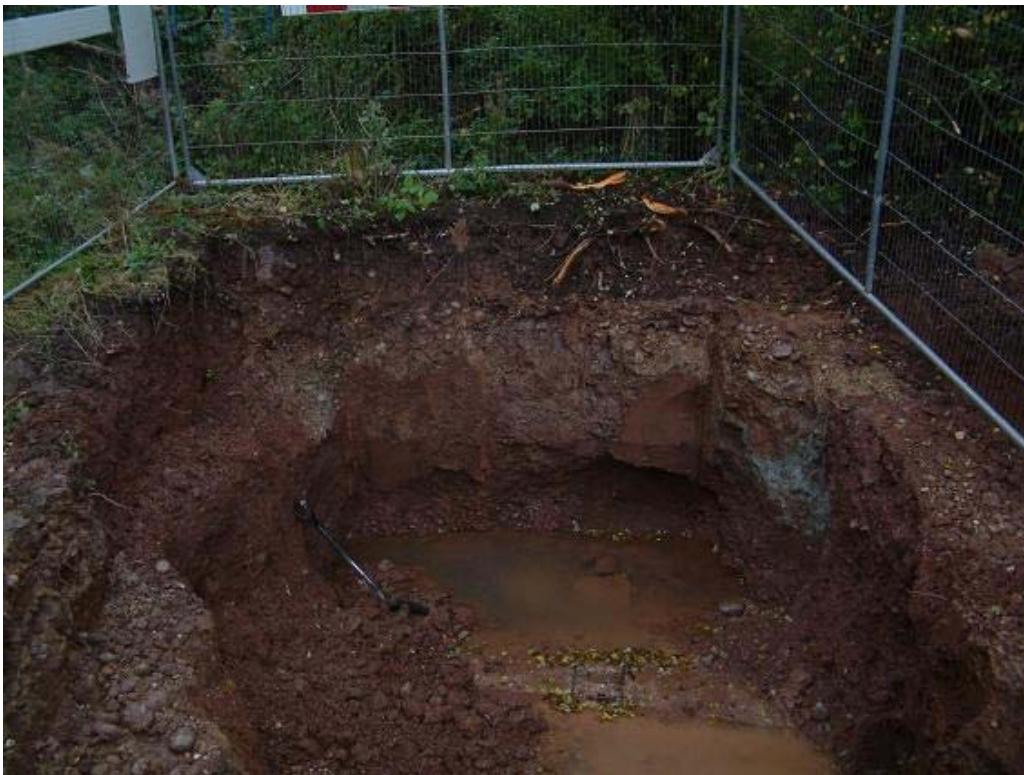
Plate 6: Northwest facing section of excavation for Manhole F1
