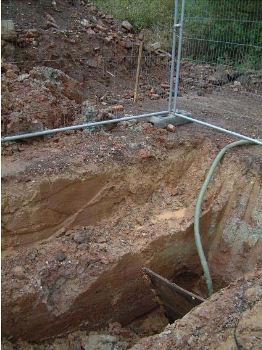
Plate 8: South facing section of trench for Manhole F2
