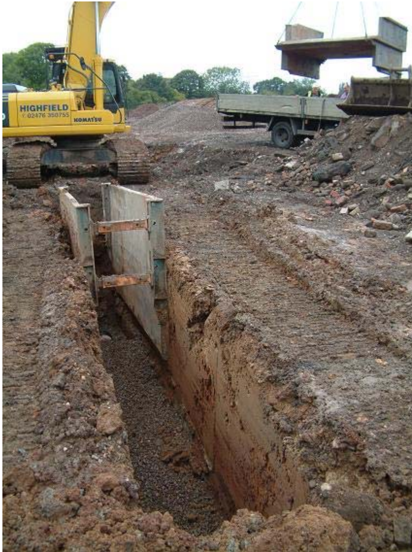
Plate 9: General shot of trench with box, west of Manhole F2
