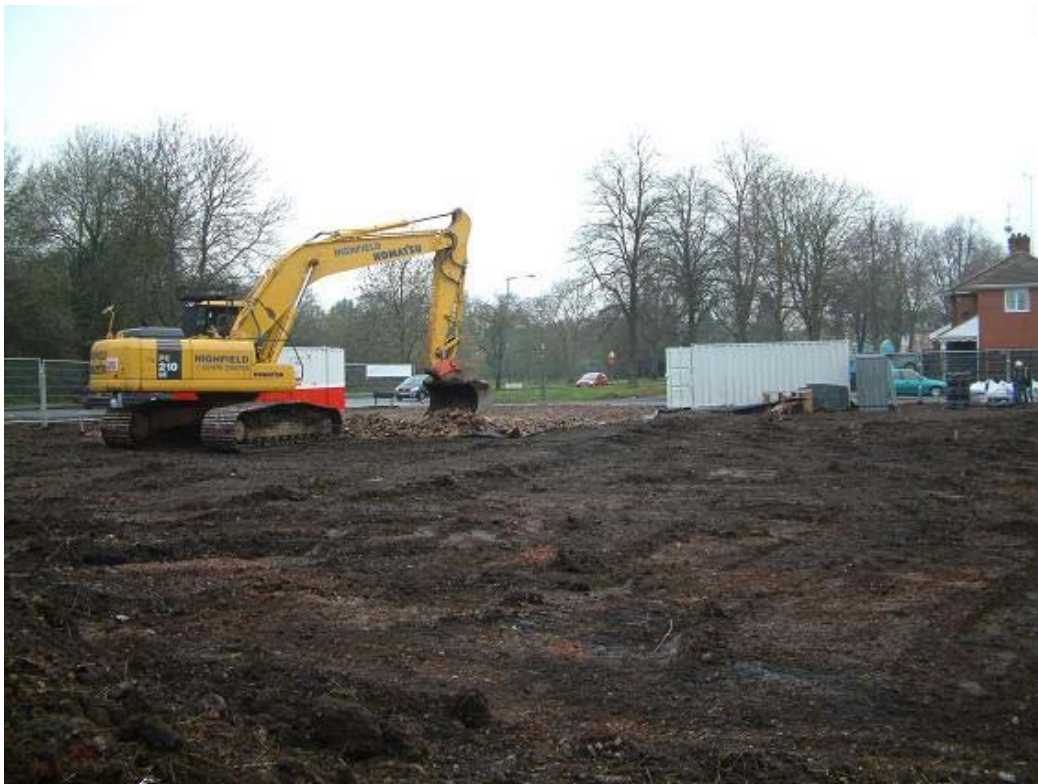
Plate 2: General shot of site after topsoil strip
