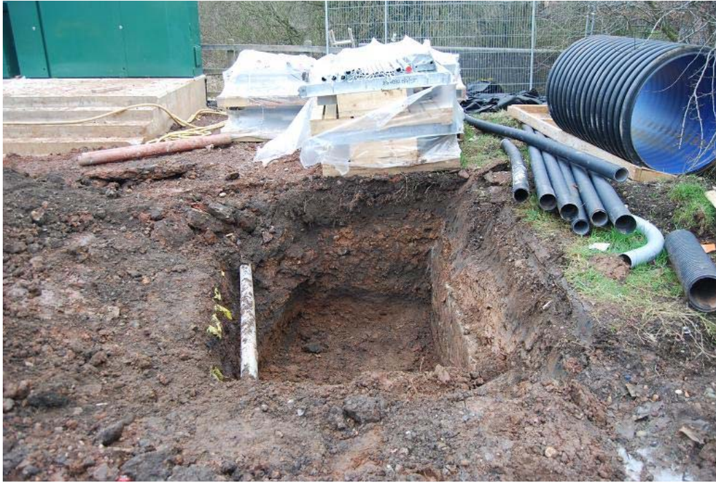
Plate 3: General shot of the Service Trench, facing east
