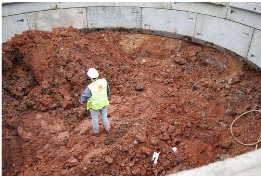
Plate 6: Excavation of the Shaft, facing north west
