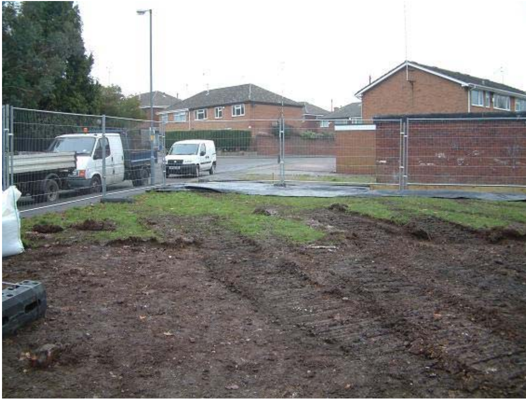
Plate 1: General shot of site after topsoil strip
