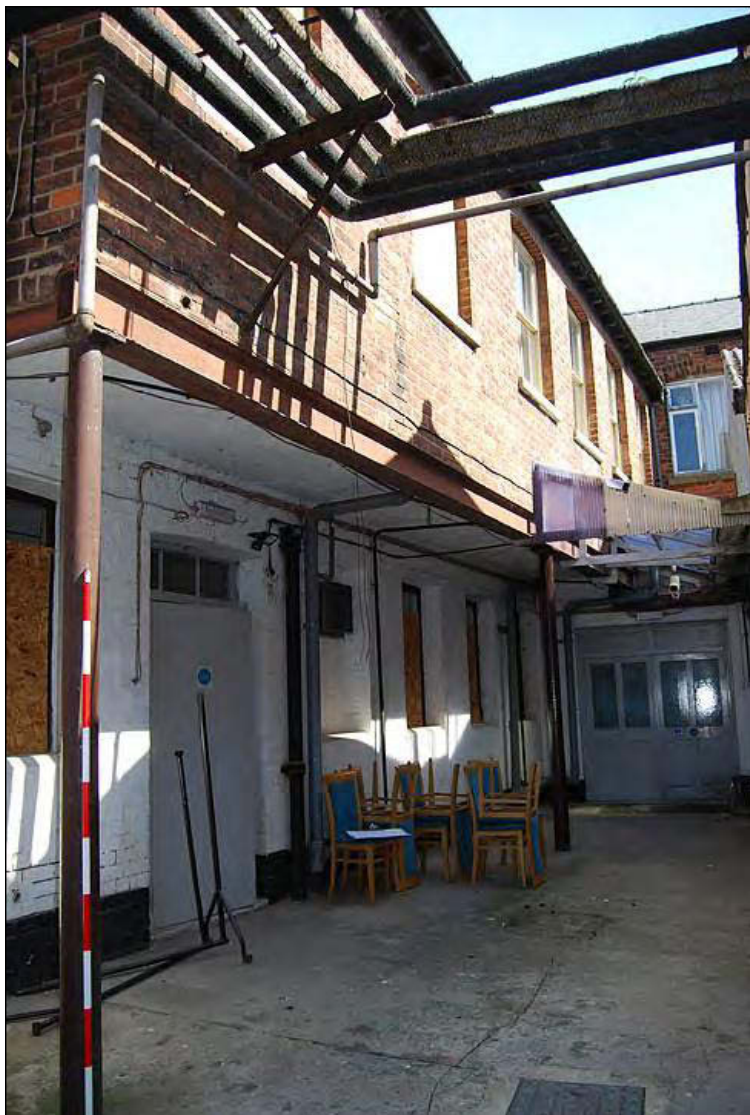
Plate 37: East elevation of building, including the ground floor alterations using reinforced steel joist and steel columns,
