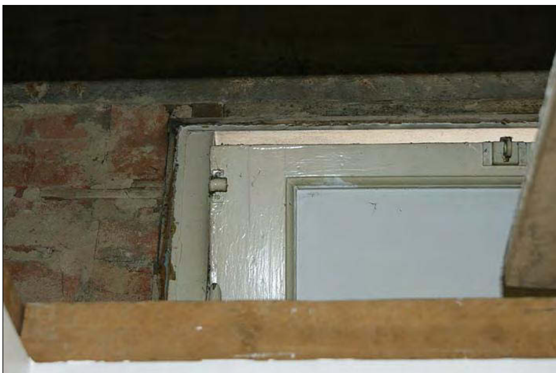
Plate 44: False ceiling concealing two-light fanlight windows on the first floor en-suite of room 20
