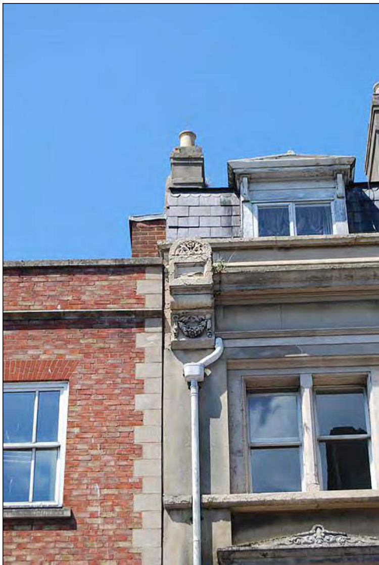
Plate 24: Third floor southern moulded and carved end bracket
