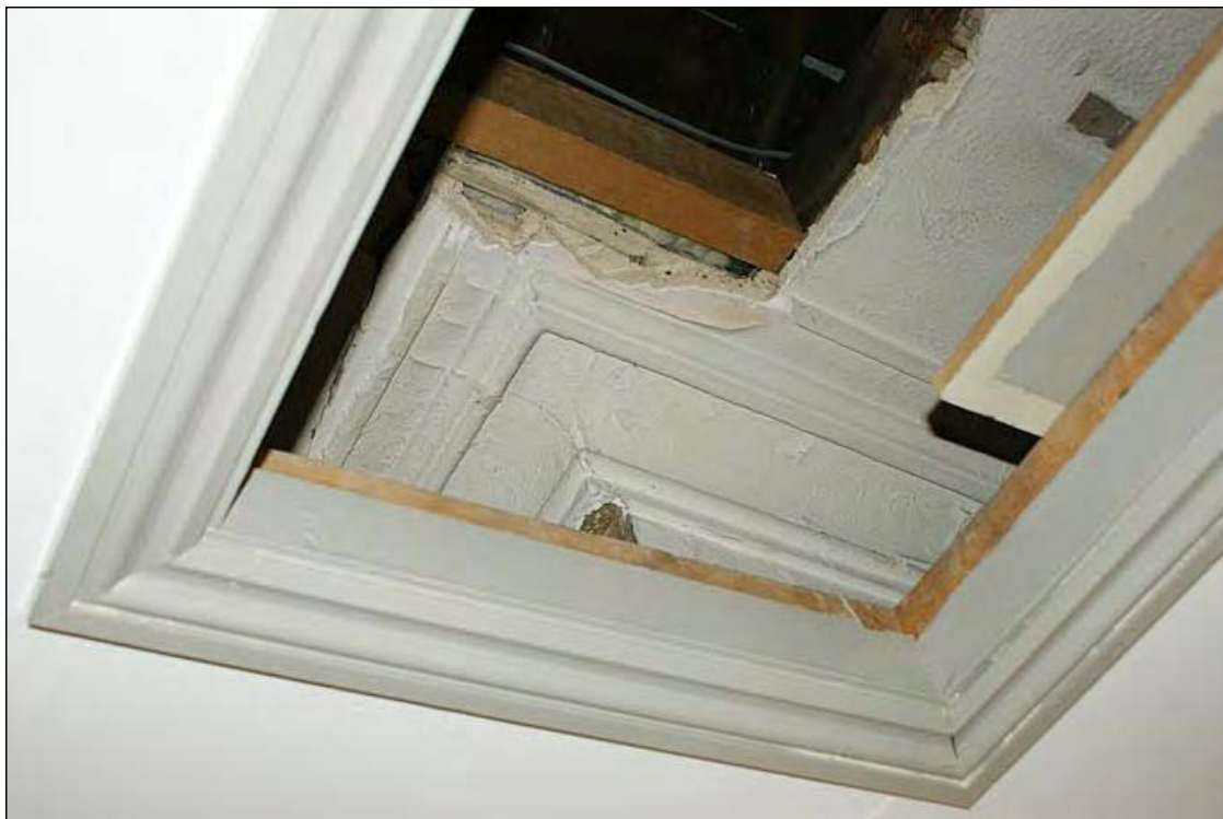
Plate 43: False ceiling concealing previous ceiling height, including coving.
