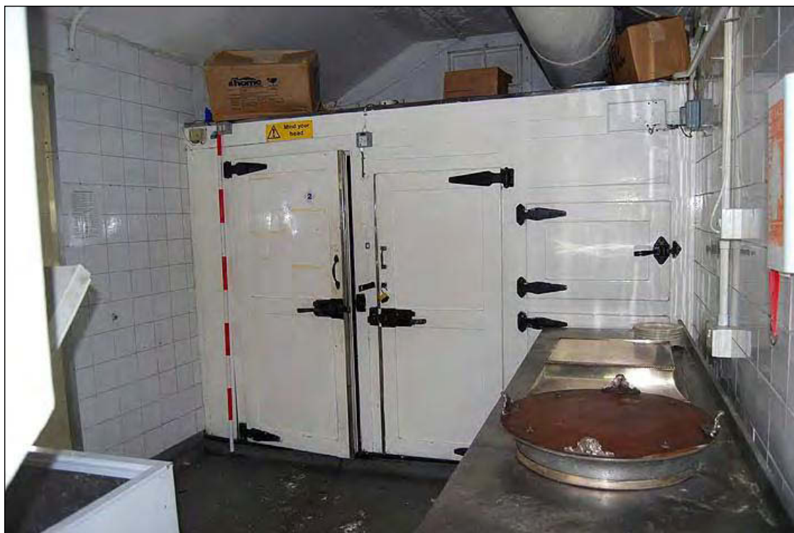
Plate 35: 1930s walk-in refrigerator attached to kitchen
