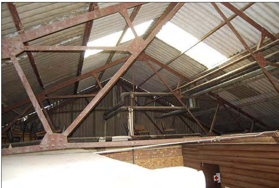
Plate 47: steel roof trusses
