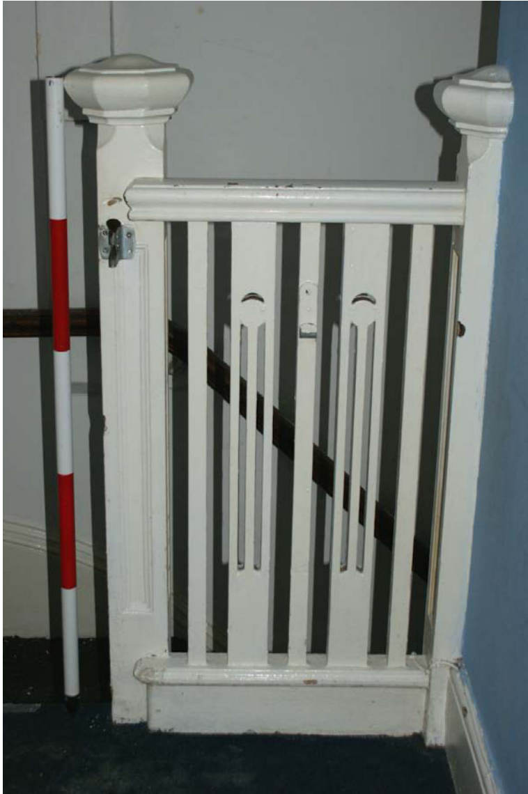
Plate 19: The decorative balustrade at the top of the stairs
