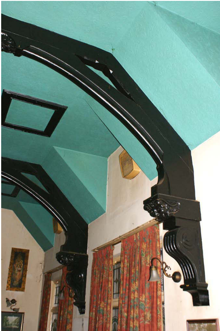
Plate 11: Detail of the decorative trusses, resting on brackets
