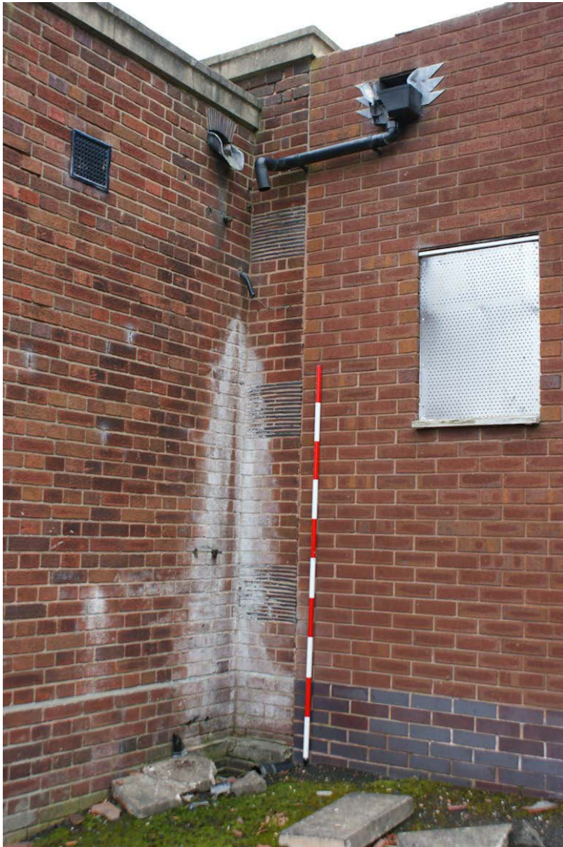
Plate 27: Building break between original structure and the men's toilets extension
