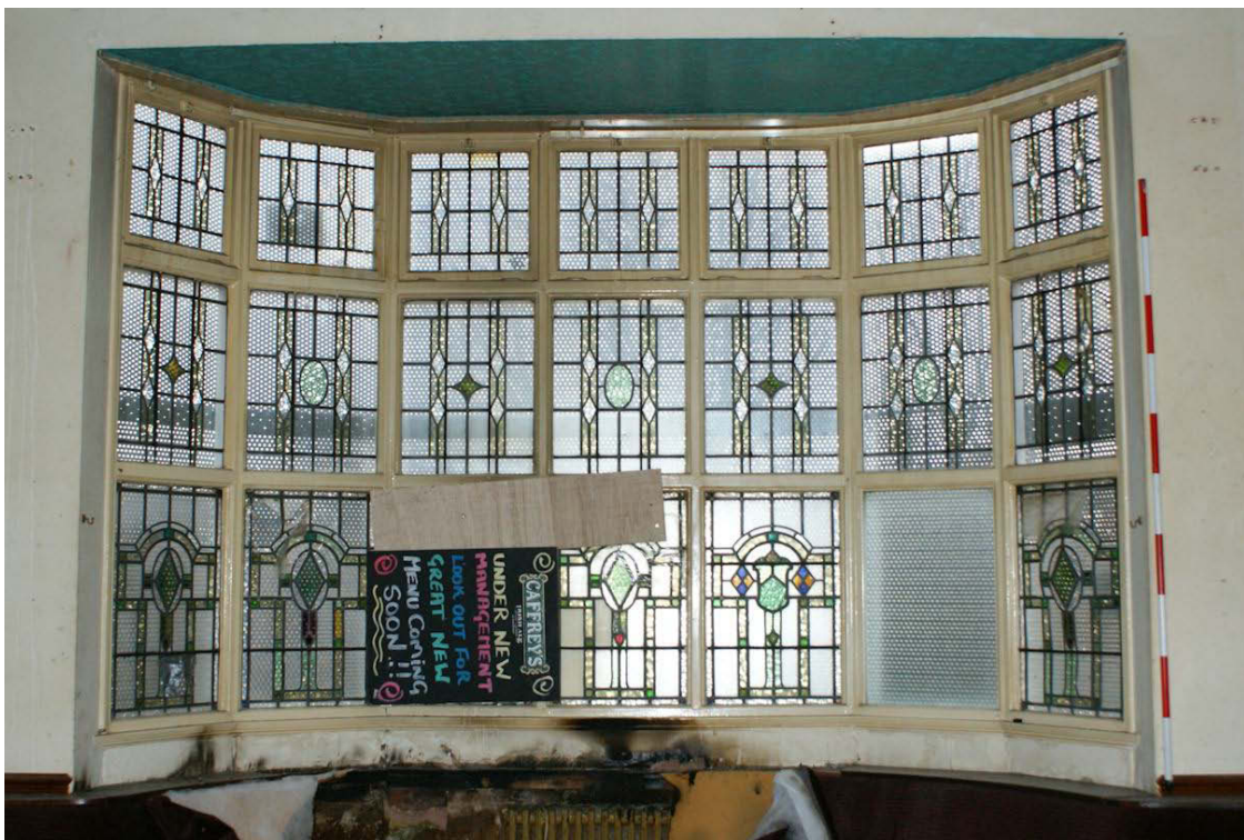
Plate 13: Detail of the large bay window with leaded lights and stained glass
