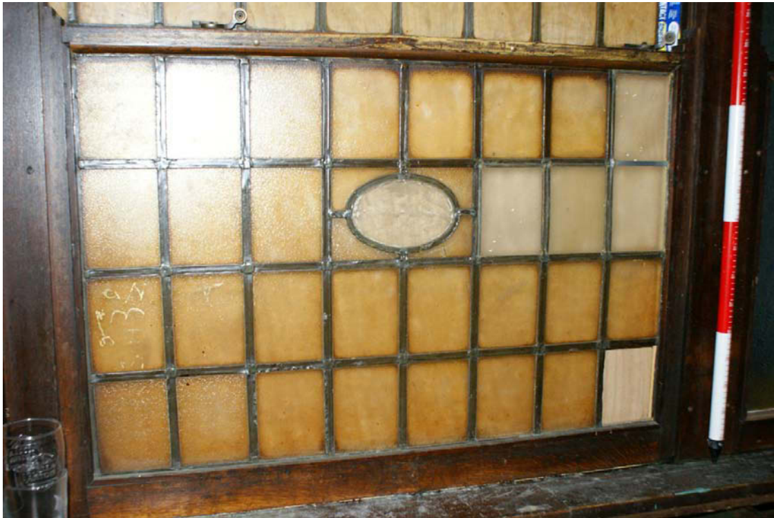
Plate 22: The sash window providing a serving hatch for the verandah
