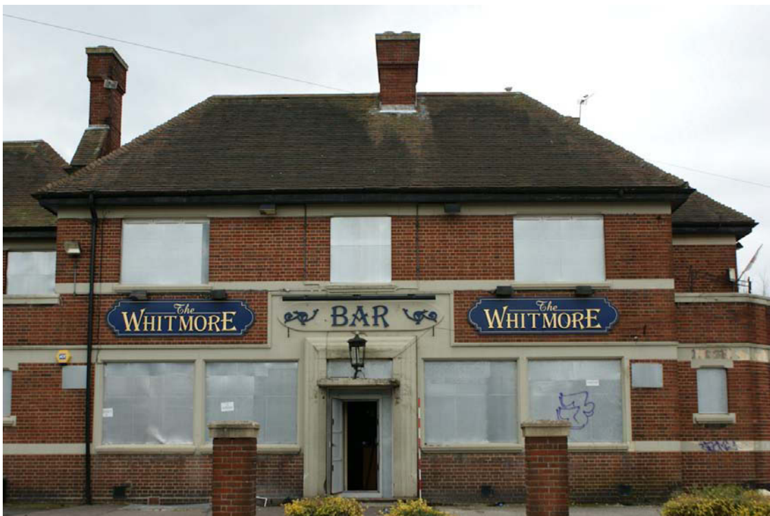
Plate 2: NW elevation of The Whitmore, and main entrance off Sadler Road
