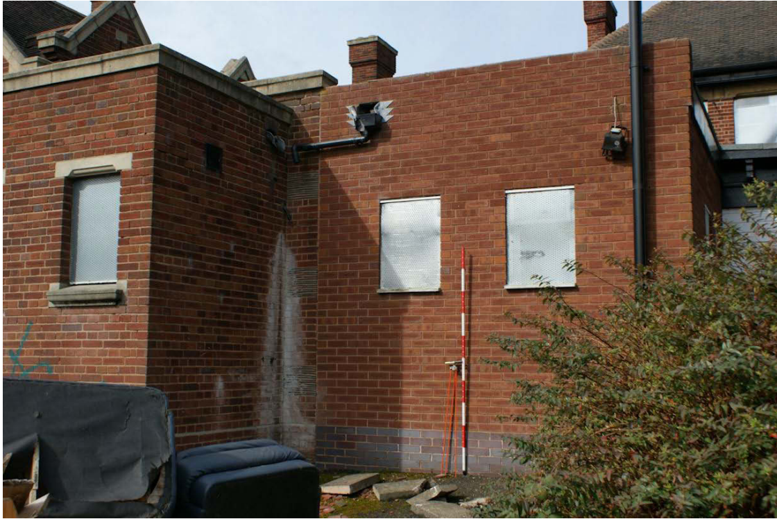
Plate 26: Extension creating the new men's toilets
