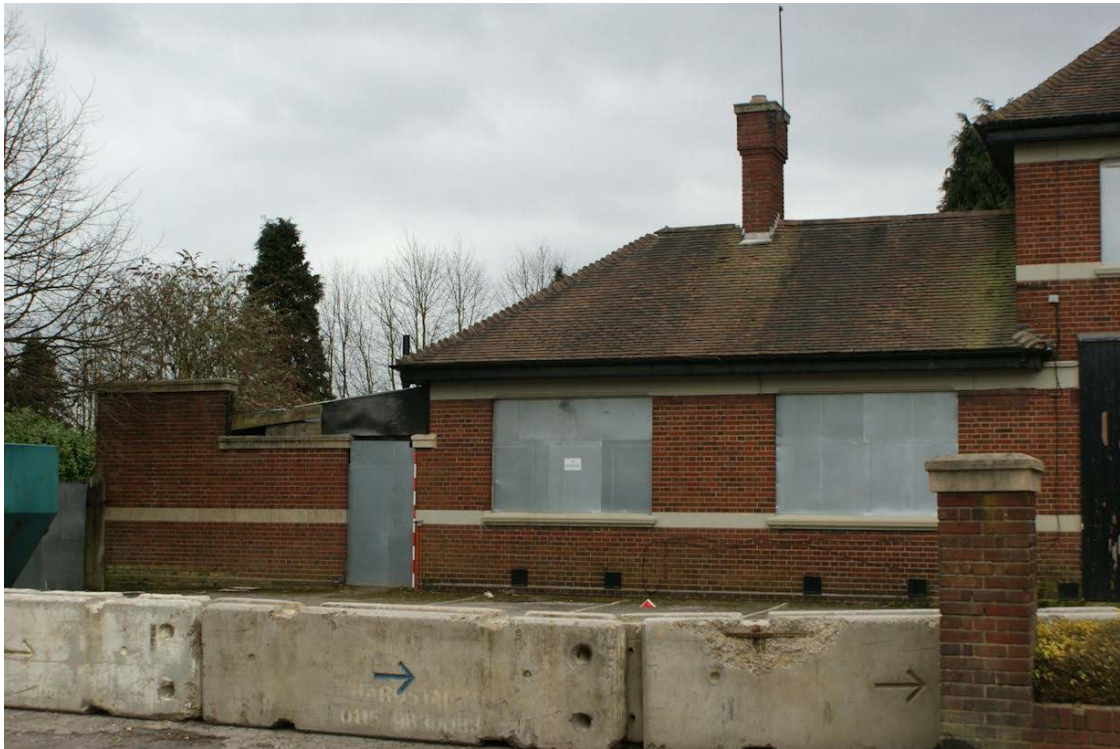
Plate 9: Northern elevation of the single storey hipped structure and private yard
