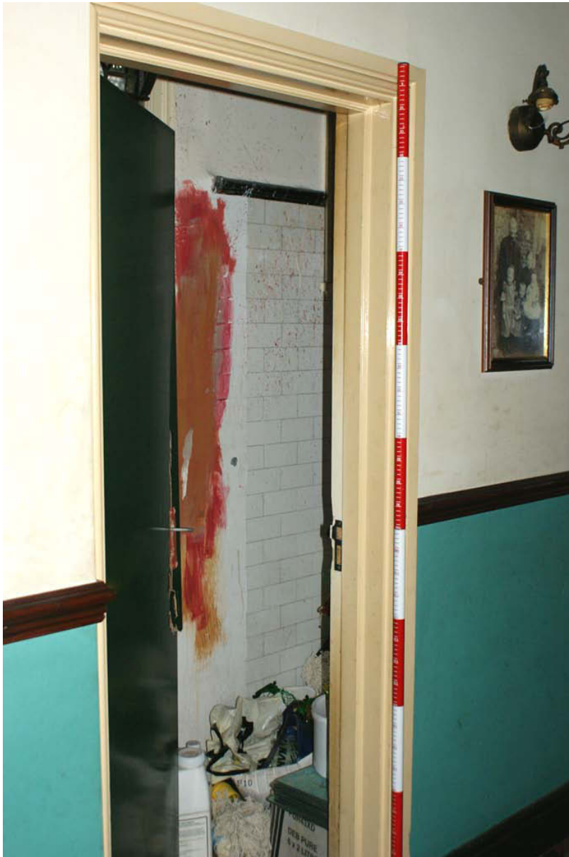
Plate 29: Former ladies toilets, reduced to a cleaning cupboard
