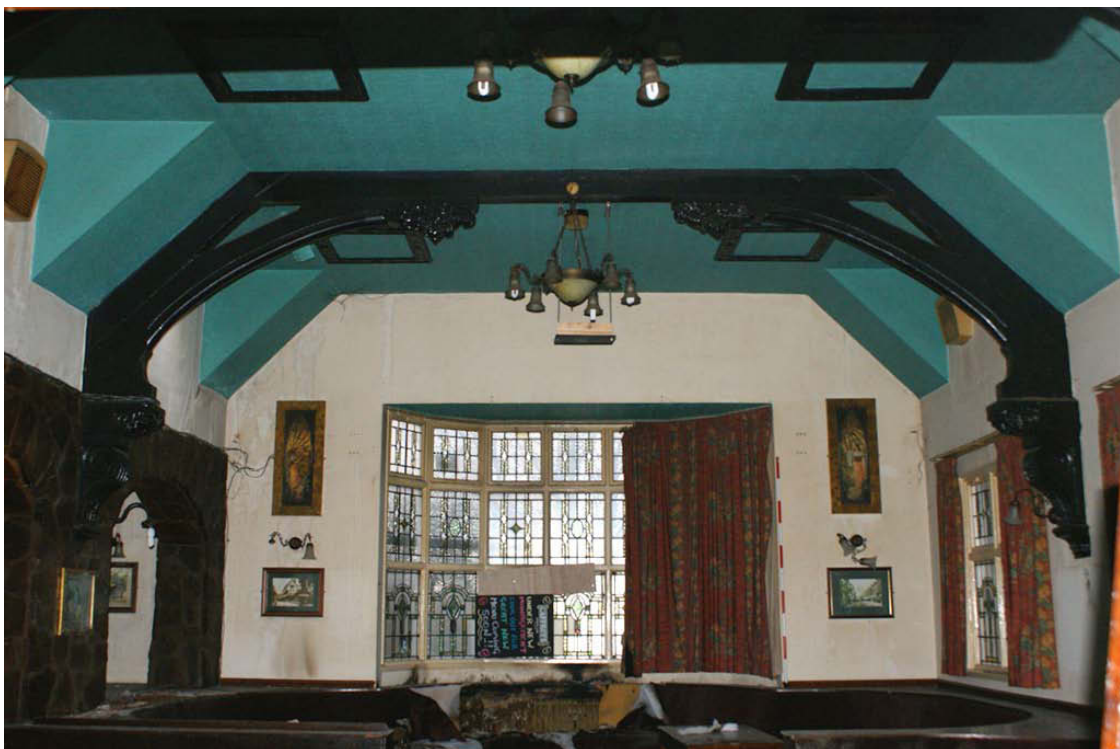
Plate 10: The large function room which was open to the roof and had decorative raised trusses
