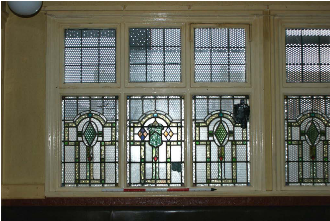
Plate 14: Example of a window within the public areas with its leaded lights and stained glass design
