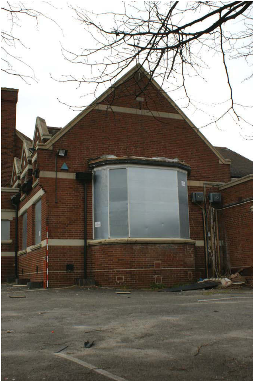
Plate 8: Detail of the southern elevation and bay window of the large function room
