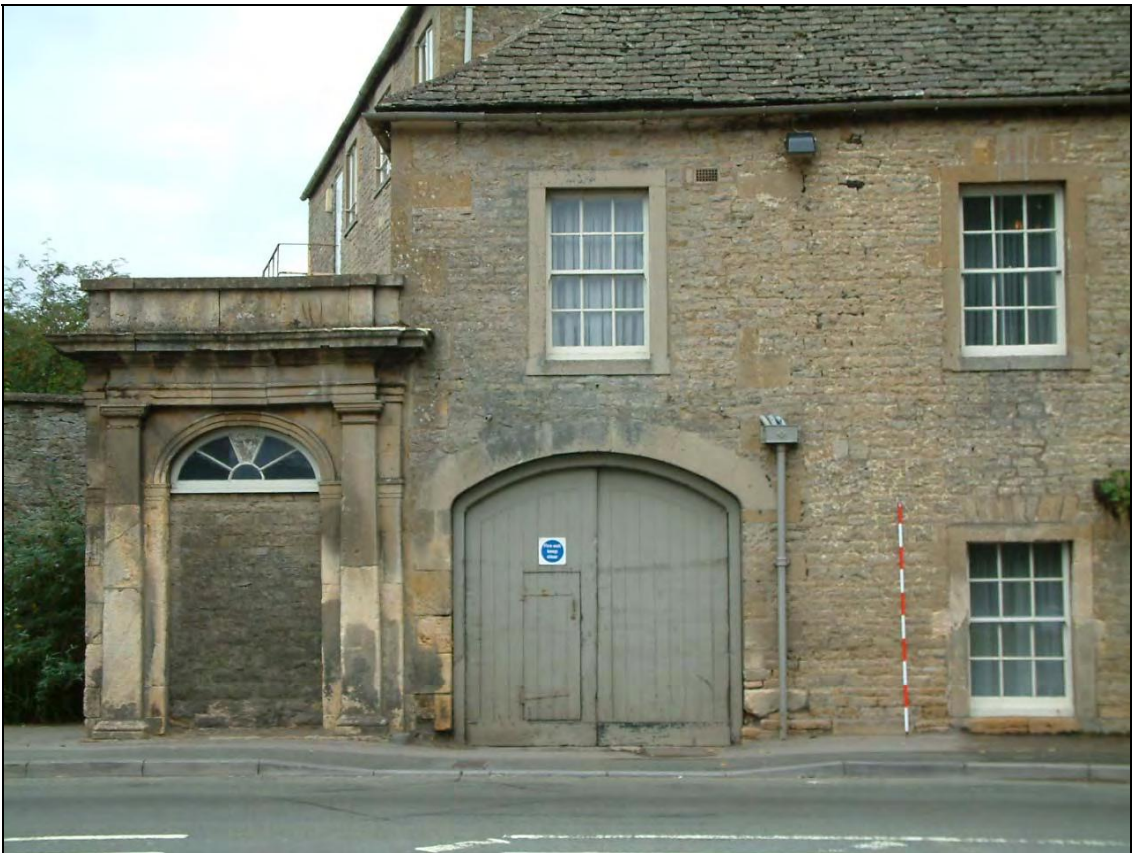
Plate 30: Added arch on Fosse Way elevation
