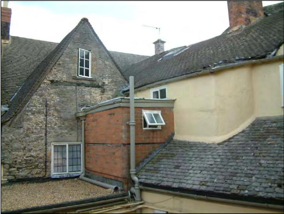
Plate 9: Seventeenth century gable at first floor
