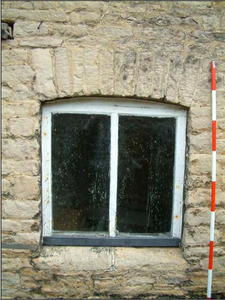
Plate 21; Window of 'the barn' extension
