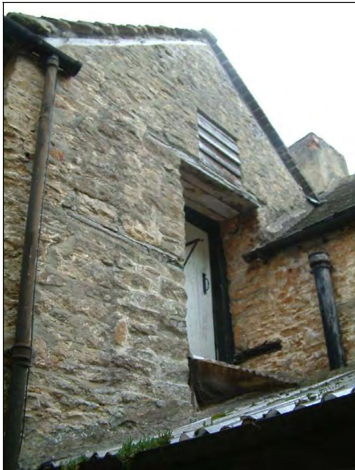
Plate 14: First floor door in gable of 'the barn'.
