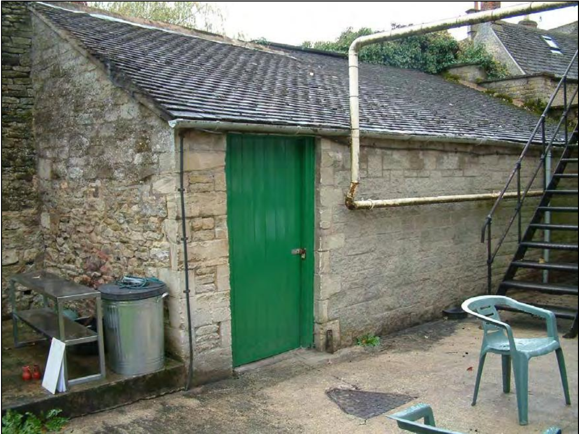
Plate 29: Shed behind Kent House
