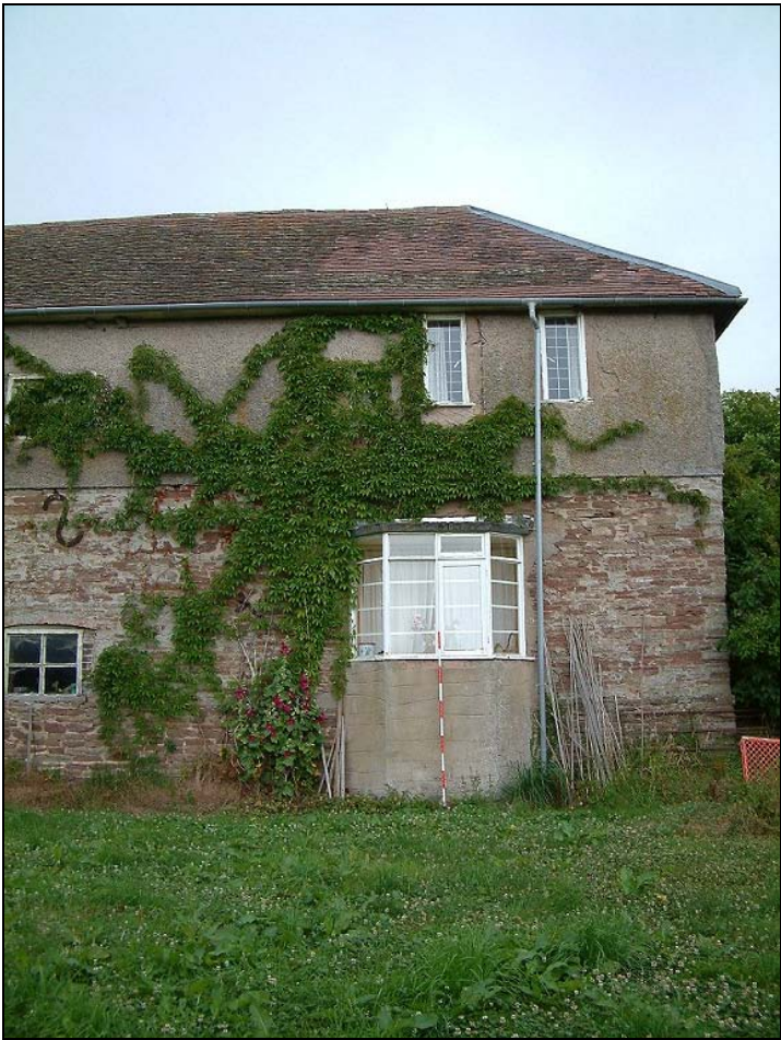
Plate 12: Added bay window to converted section of barn
