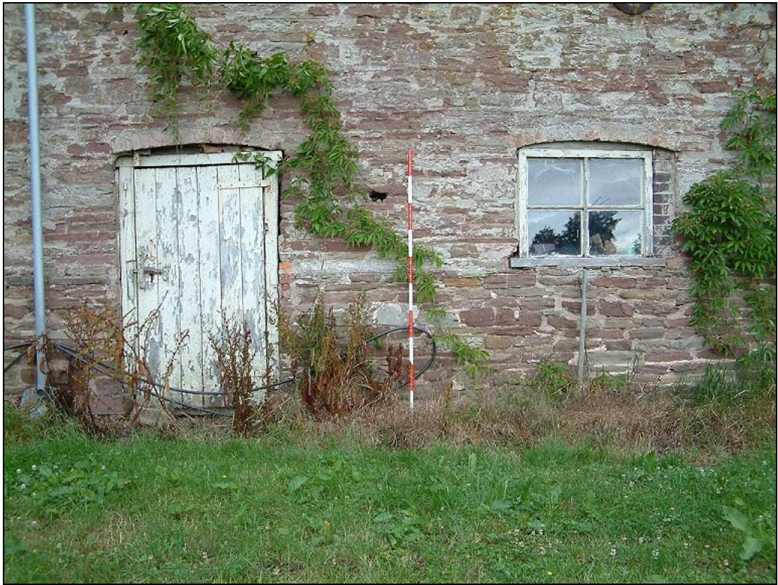
Plate 13: Inserted windows in barn
