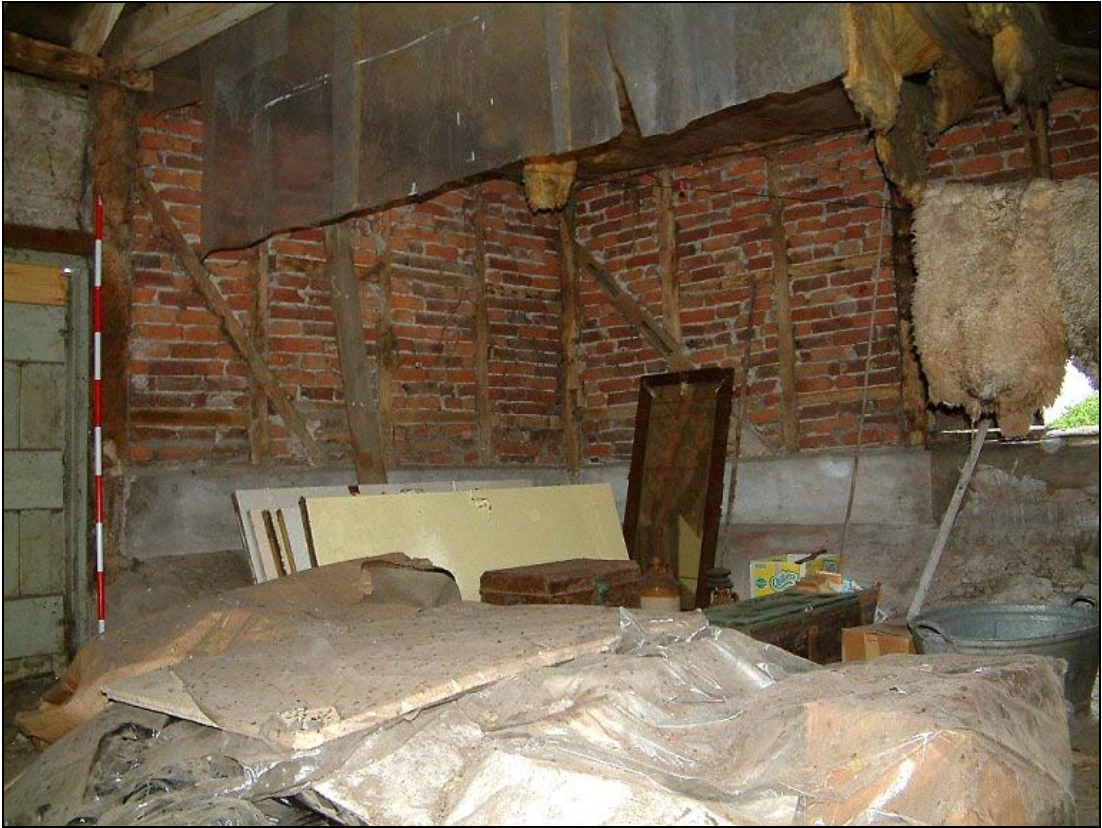
Plate 3: First floor timber-framing
