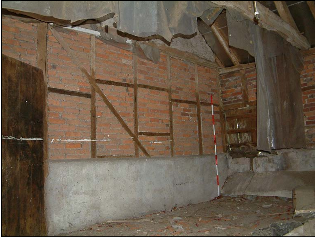
Plate 9: Inserted dividing wall in barn
