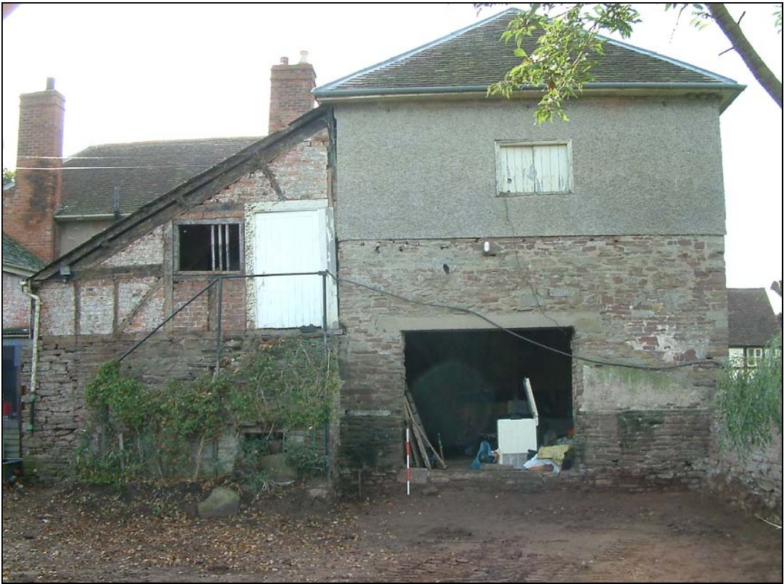
Plate 4:Lean-to extension to barn
