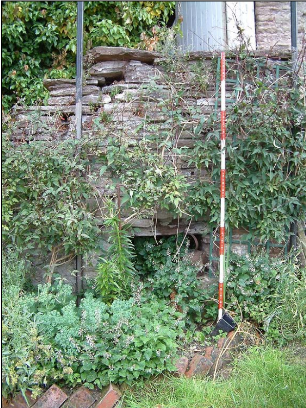
Plate 7: Kennel below stairs
