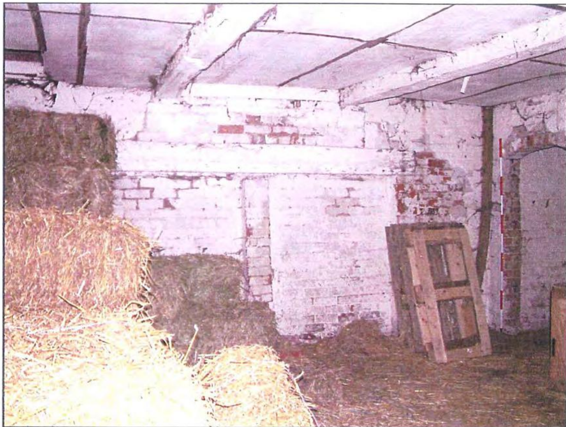
Plate 8: Central section interior ground floor, showing hay storage and blocked west opening
