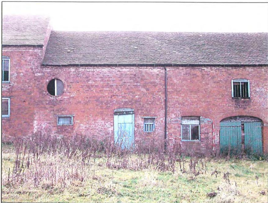
Plate 18: West section, east half, from the north showing the pitching eye
