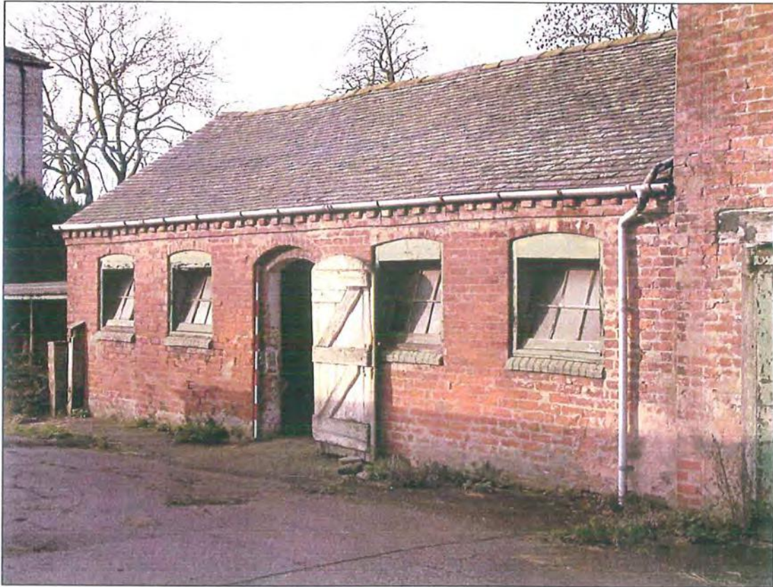
Plate 1: Southern section of the west range from the north-east
