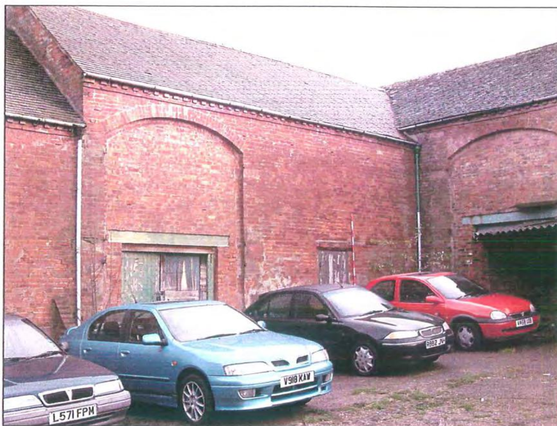
Plate 29: North range east section from the south west
