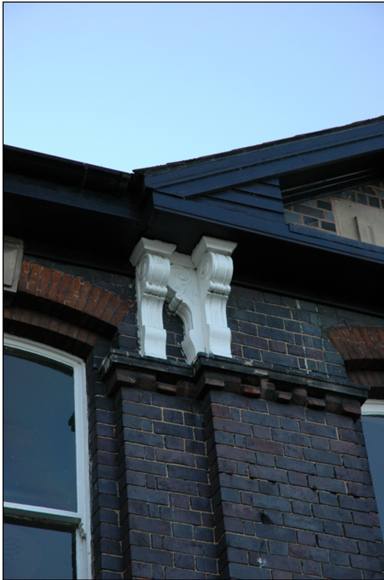
Figure 12: Eaves brackets
