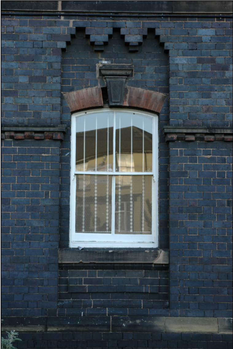
Figure 9: Sash window on Tipton Police station
