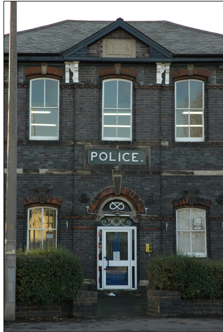
Figure 13: Front entrance bay
