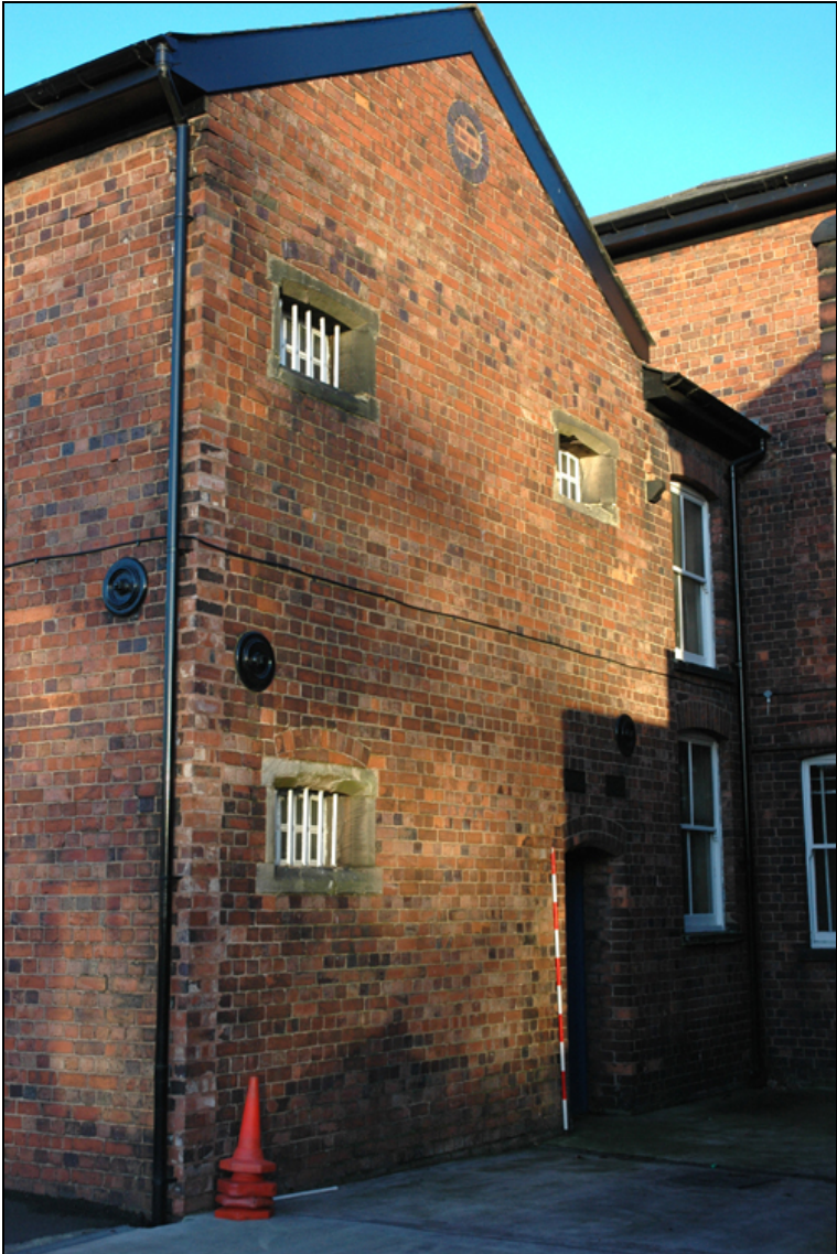
Figure 14: Two storey cell block
