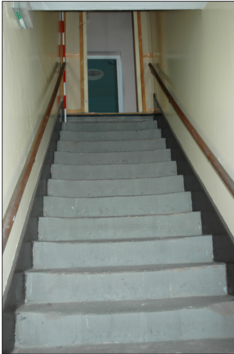
Figure 34: Magistrate's Court staircase
