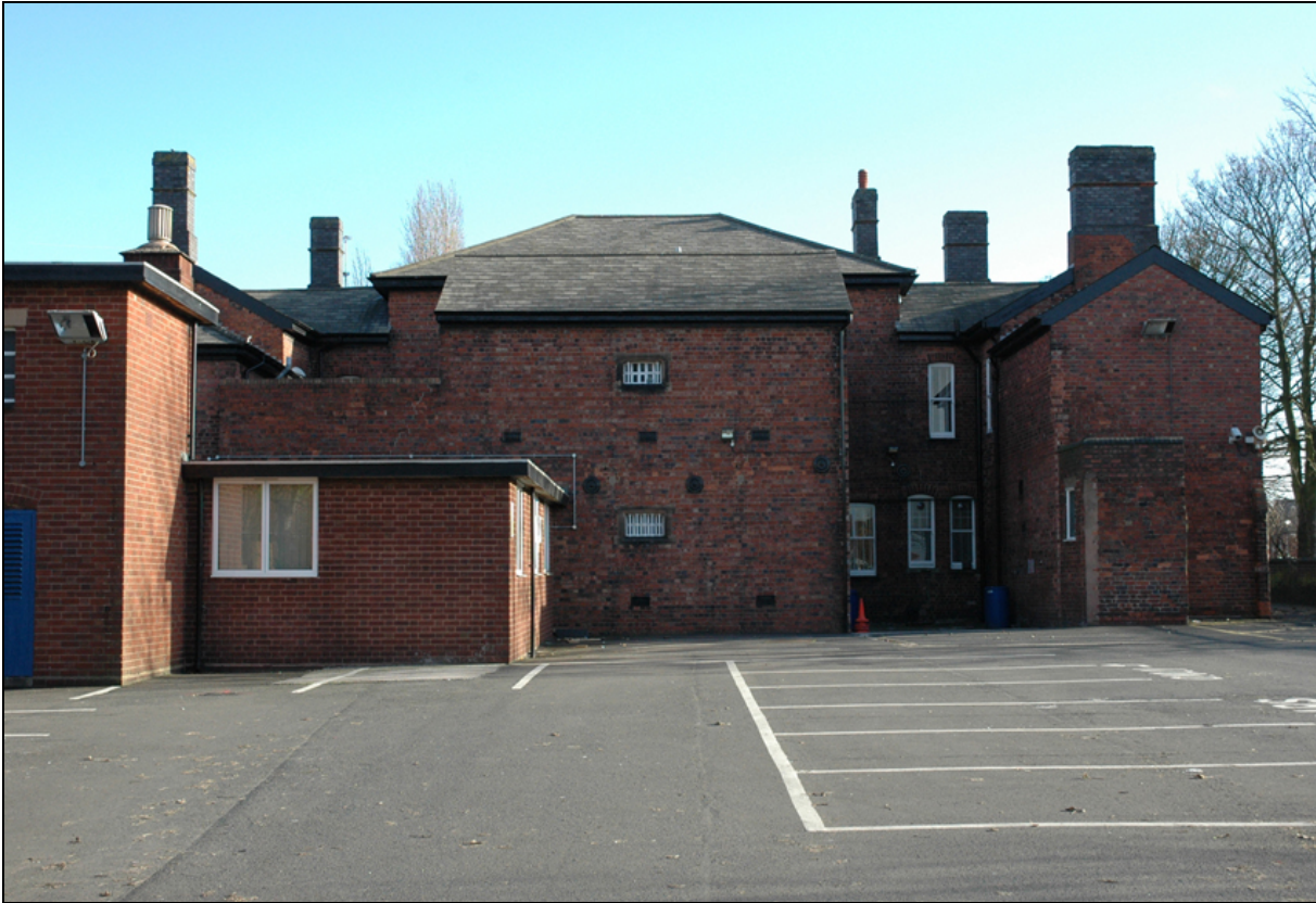
Figure 42: Extensions to rear of cells
