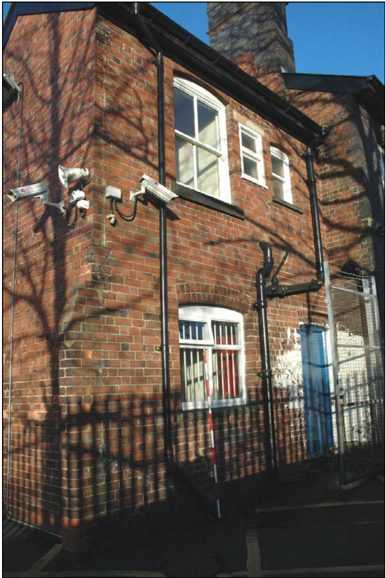
Figure 37: south wing extension
