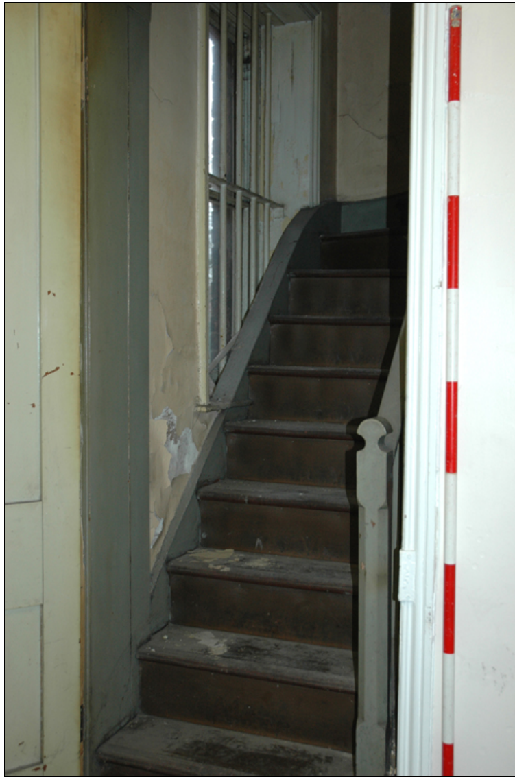
Figure 27: Staircase to Court from Offices
