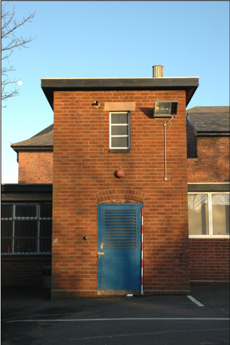
Figure 43: Boiler room extension
