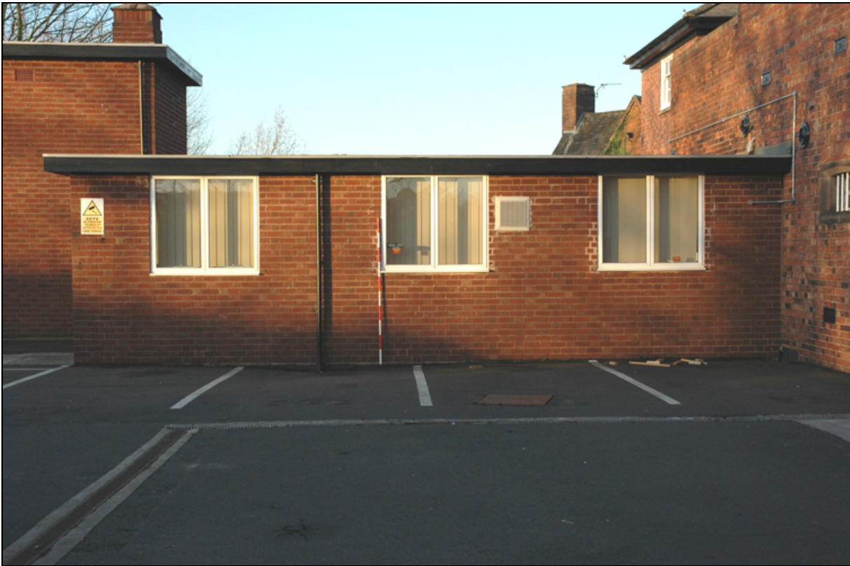
Figure 44: Parade room and office extension
