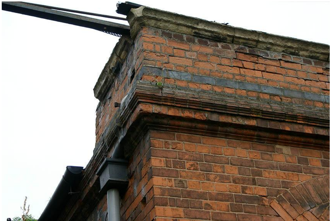
Plate 13: Building 6 cornice and parapet
