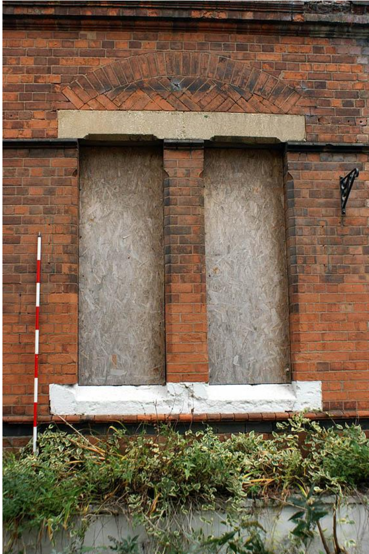
Plate 10: Building 6 window showing cill string course
