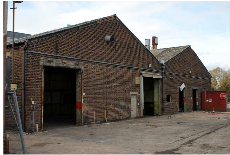
Building 9 from the south east
