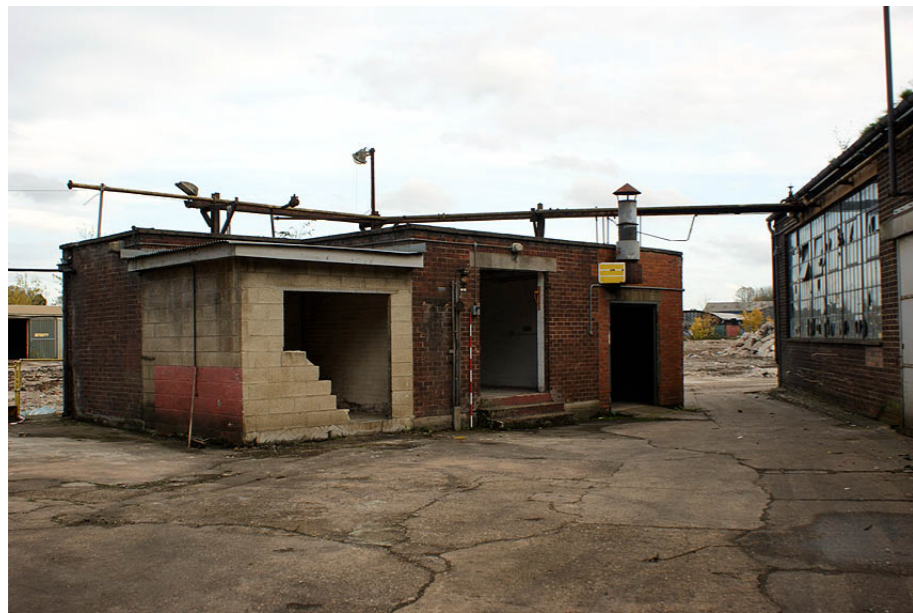
Building 15 from the south west
