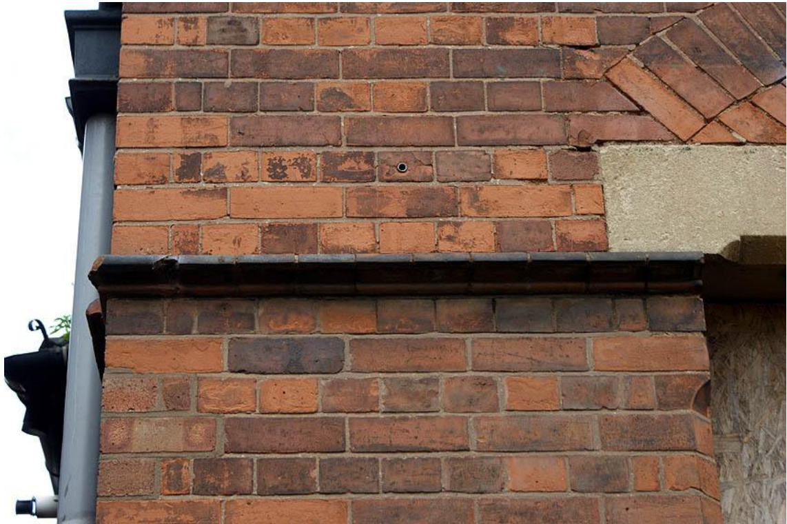
Plate 11: Building 6 showing lintel string course
