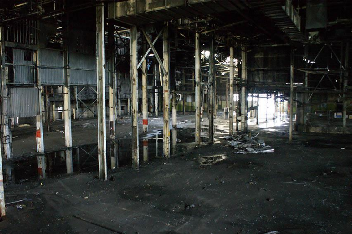
Plate 23: Stanchions in interior of building 7
