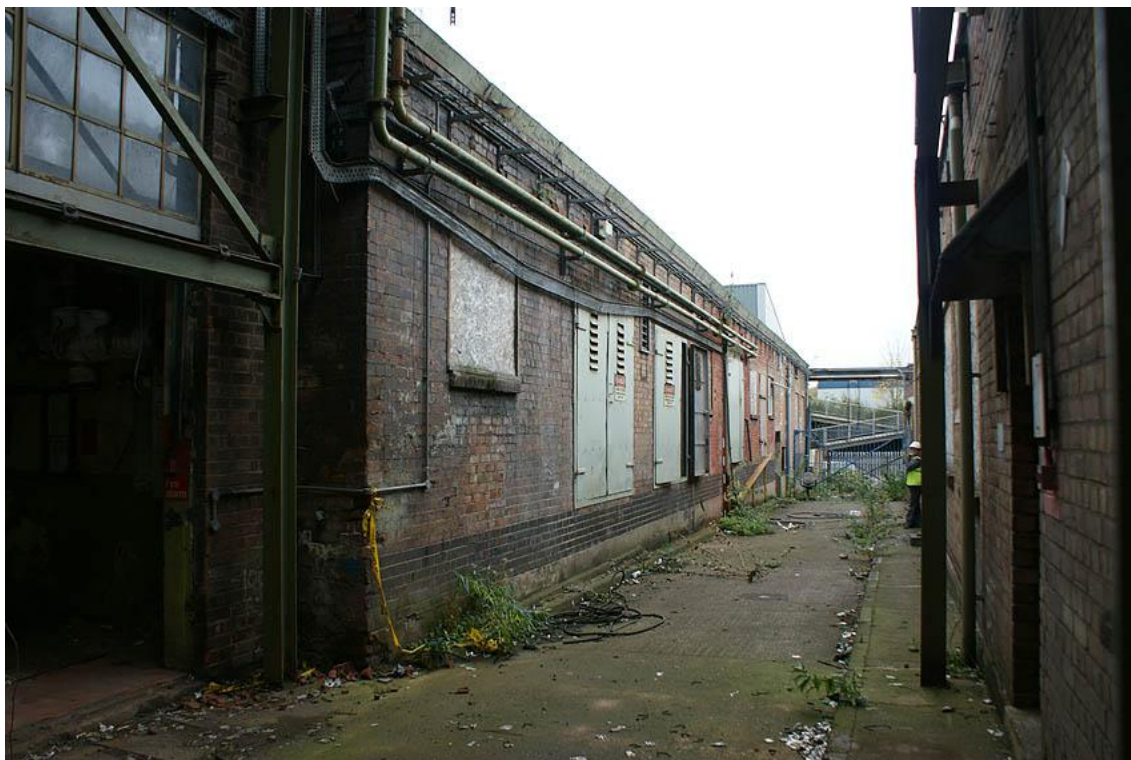
Plate 41: Exterior of building 7, wall of 1901 stove room
