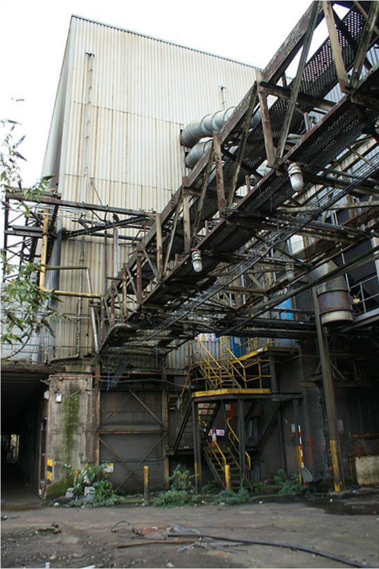
Plate 22: Walkways and stairways on exterior of building 7
