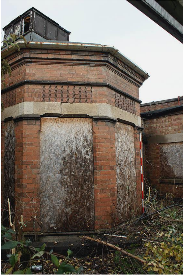
Plate 16: Building 6 bay window from the south east
