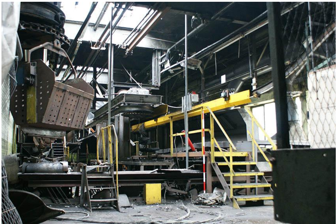
Plate 26: Bridge-way between building 7 and the maintenance building
