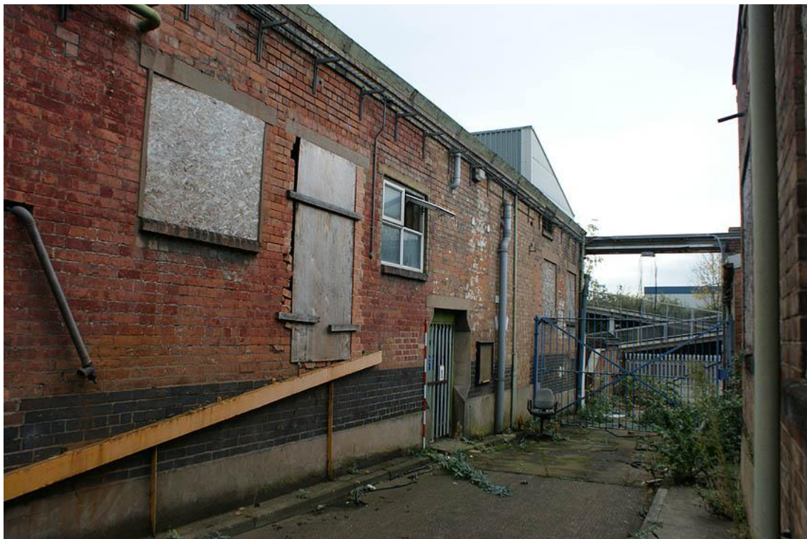
Plate 44: Historic north wall of building 7
