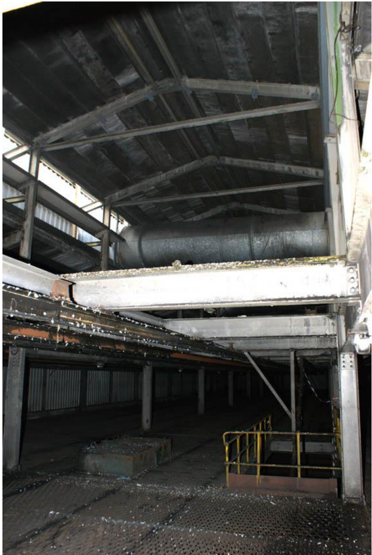
Plate 32: Stanchions and joists in interior of maintenance building
