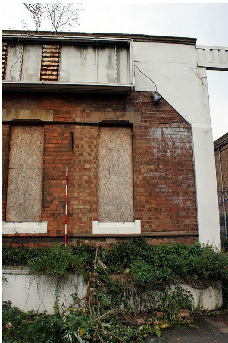
Plate 14: Building 6 extension from the west
