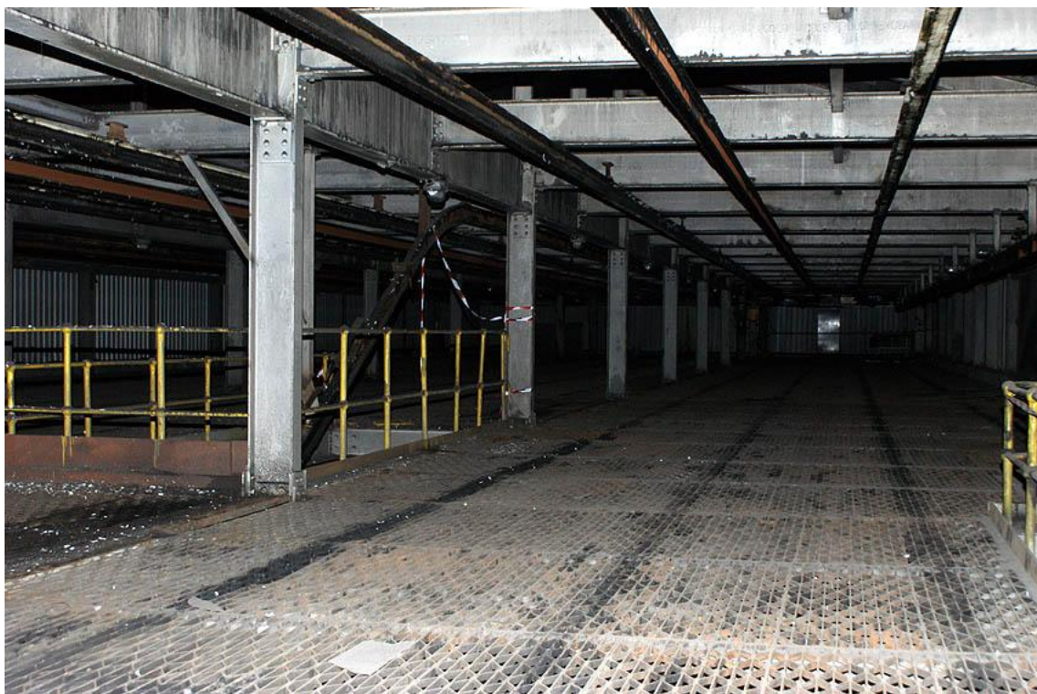
Plate 34: Interior 3 rd floor of maintenance building
