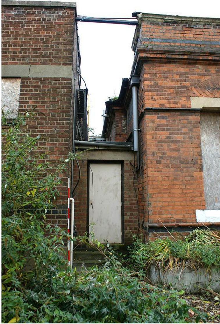
Plate 19: Link between building 5 (left) and building 6 (right)
