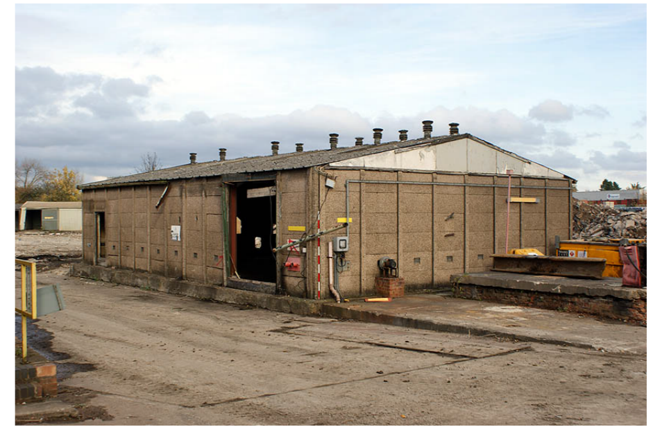
Building 10 from the south west
