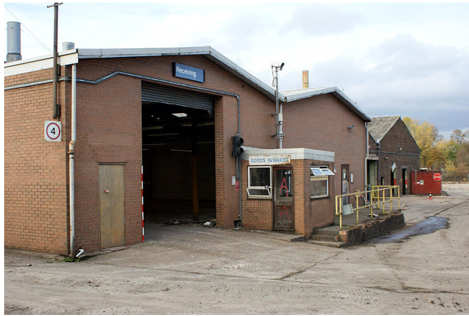
Building 8 from the south east
