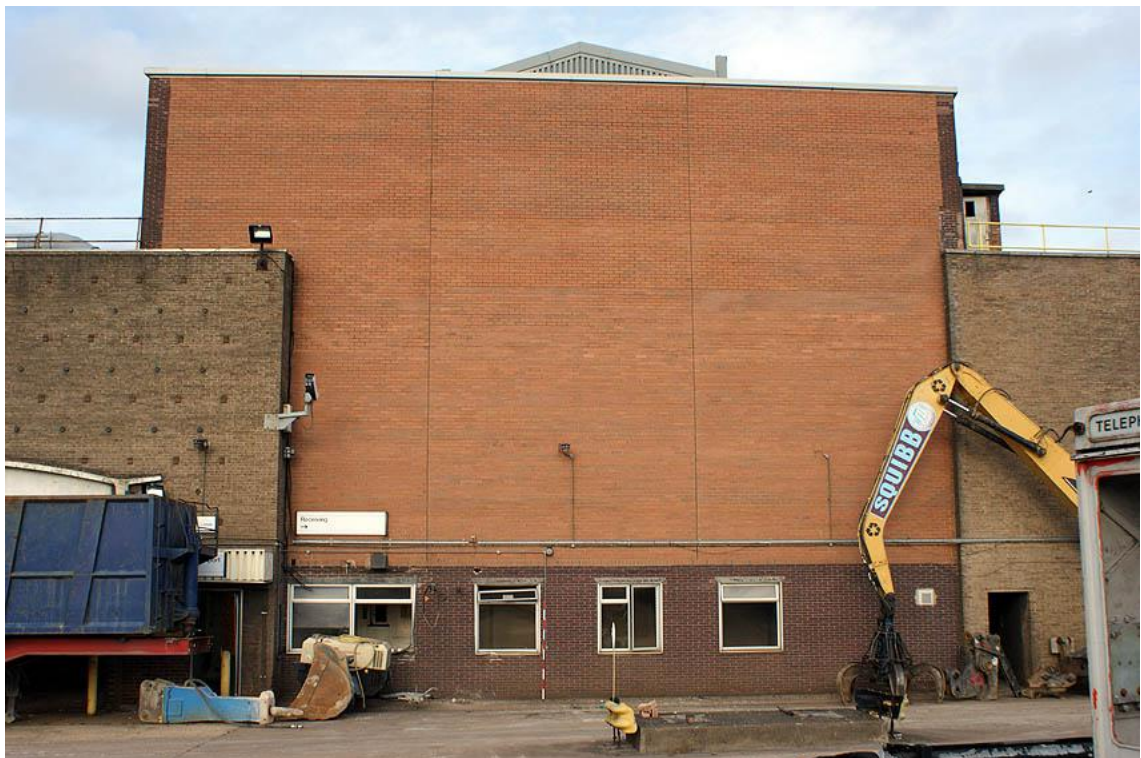
Plate 28: Maintenance building, south gable, from the south
