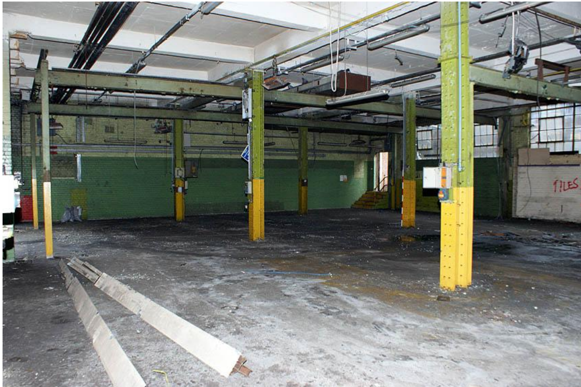
Plate 33: Interior ground floor of maintenance building
