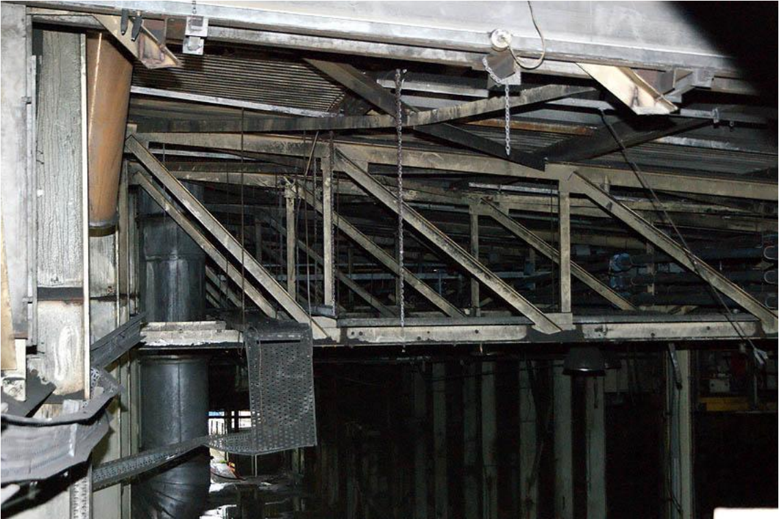
Plate 24: Trusses in interior of building 7
