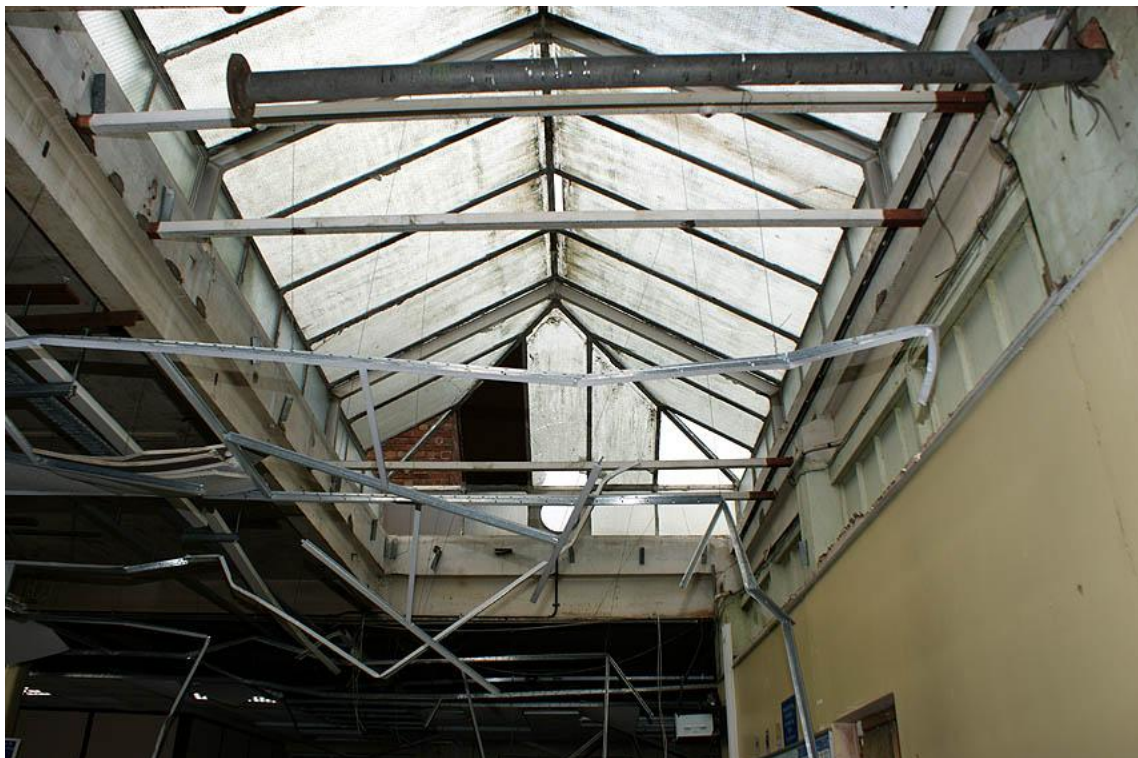
Plate 6: Skylight in building 5
