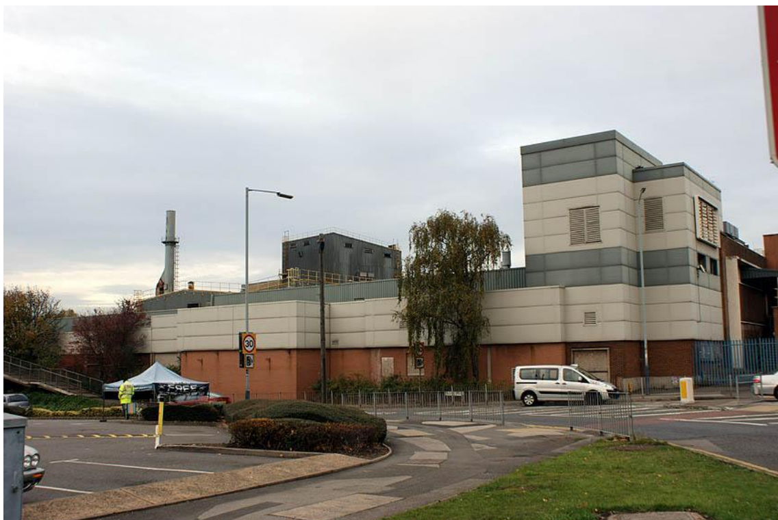
Plate 21 Building 7 from the west
