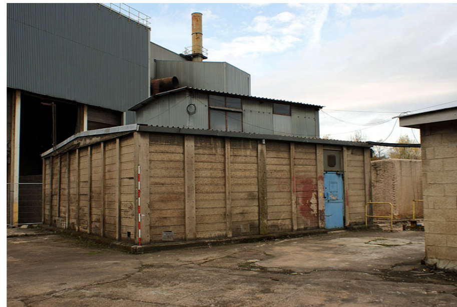
Building 16 from the south east
