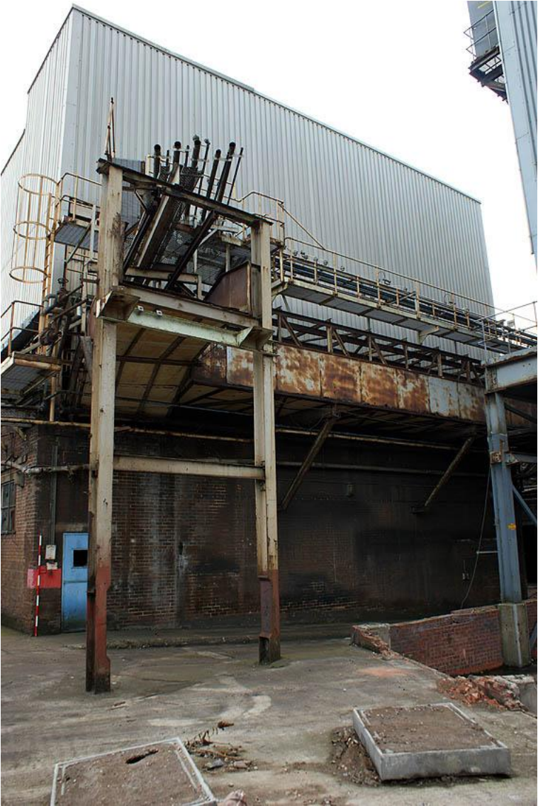
Plate 31: North gable of the maintenance building
