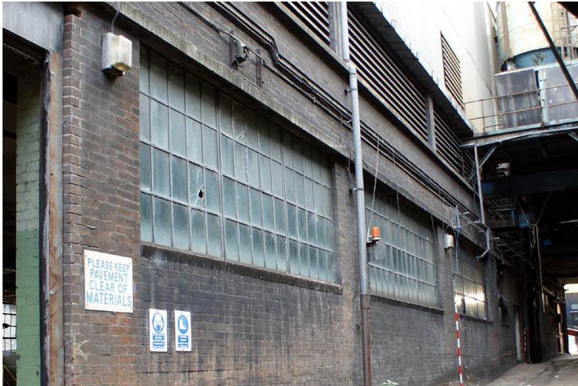
Plate 29: Maintenance building, windows on the west wall, from the north west
