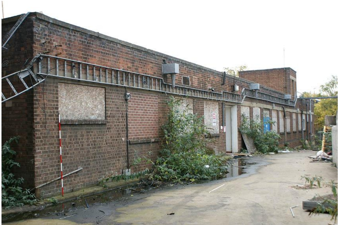
Plate 1: Building 5 from the north east
