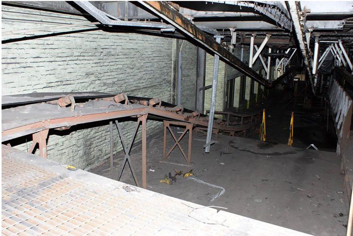
Plate 39: Conveyor belt on second floor of maintenance building
