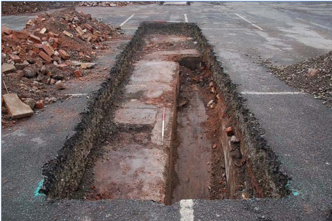
Plate 3 Trench 2 looking North showing modern 20 th Century structure and truncation by a service trench to the north.
