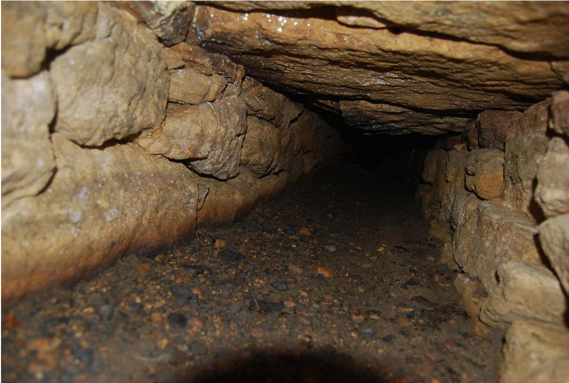
Plate 1; Sample view of stone culvert construction, looking west
