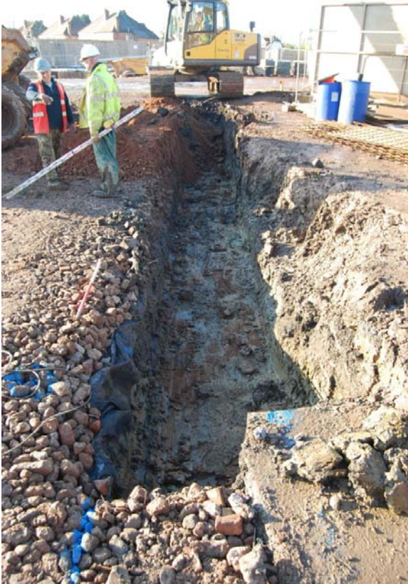
Plate 2 Excavation of footings
