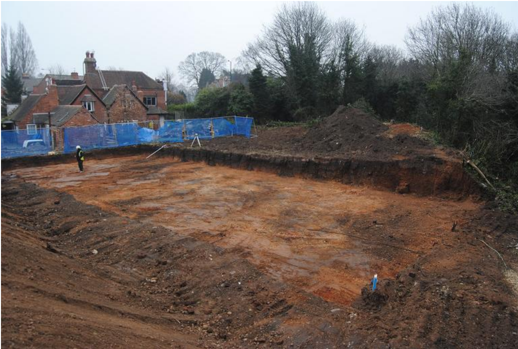
Plate 1 Trench 2 looking east
