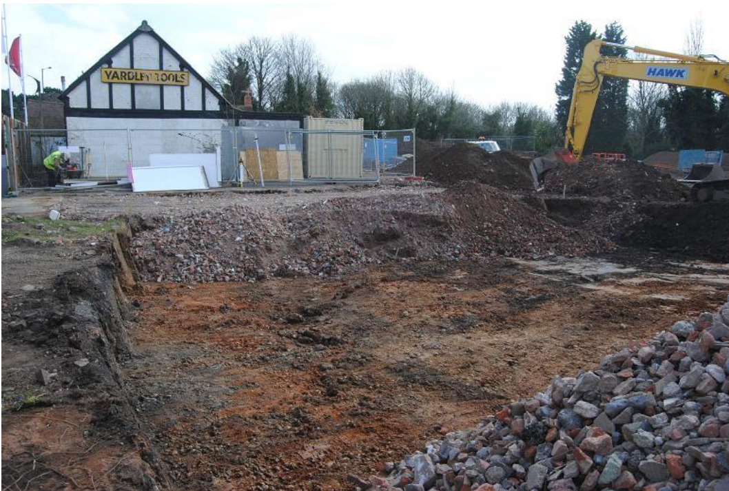
Plate 2 Trench 4 looking south east
