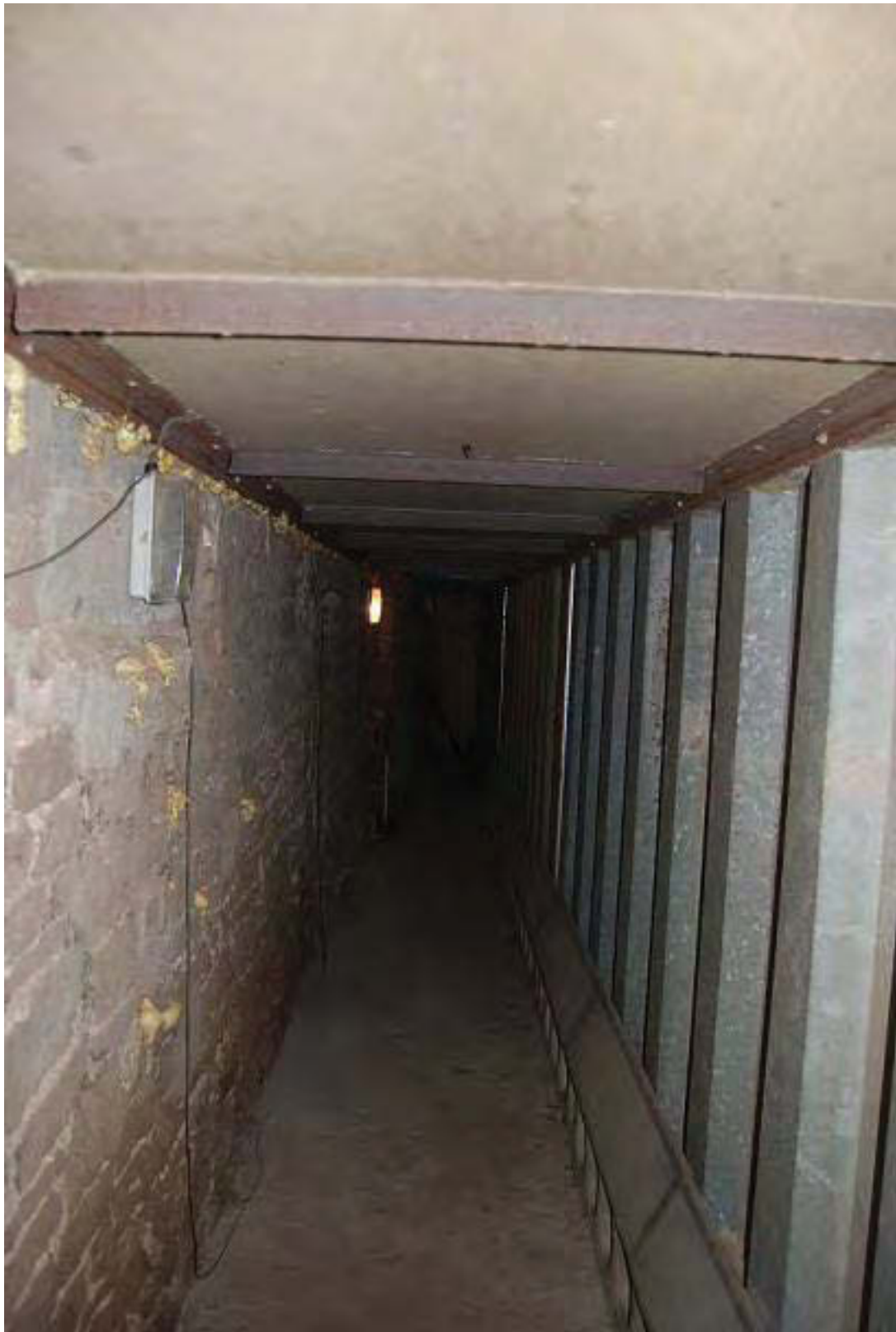
Plate 5 Wall of historic barn on left to be exposed. Wall of modern barn on right to be demolished
