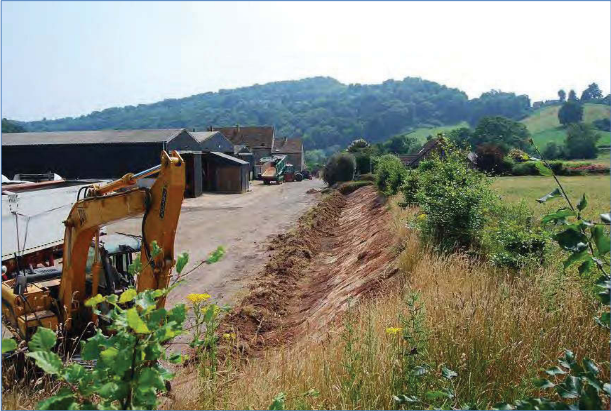
Plate 9 Western bank exposed looking south towards existing barns and priory buildings
