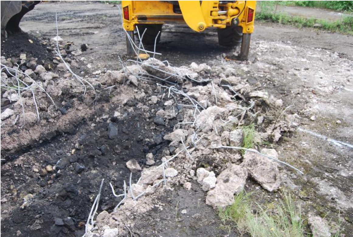
Plate 15 Excavation of Trench 4 showing the extensive reinforced concrete, looking north
