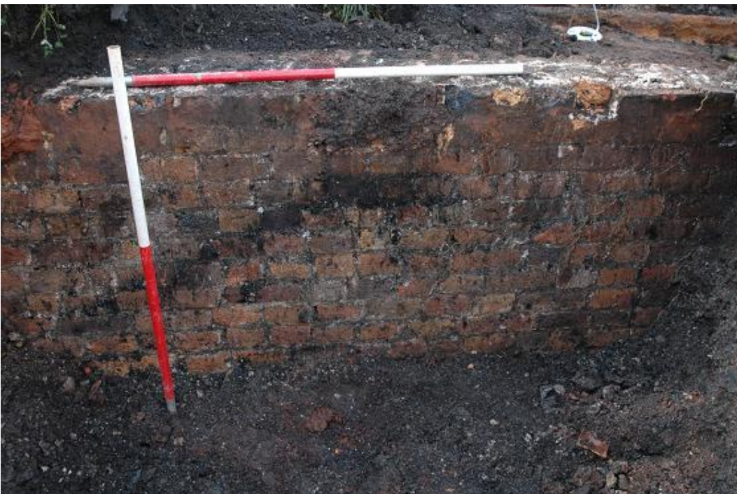
Plate 22 Wall 3001, looking south-west
