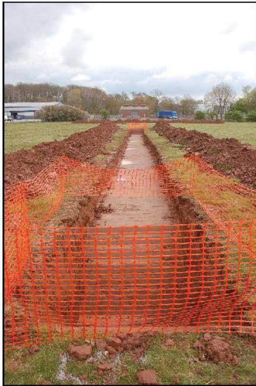
Plate 7 Trench 5 overall, looking south-east
