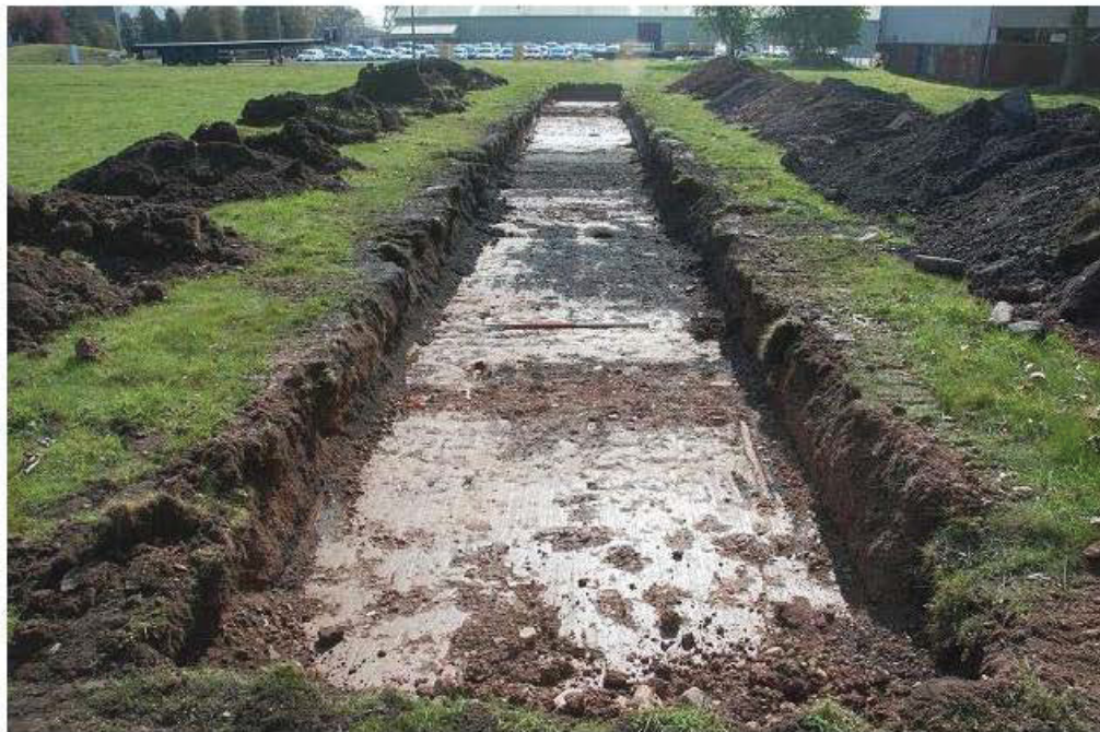
Plate 22 Trench 18 excavated, looking east
