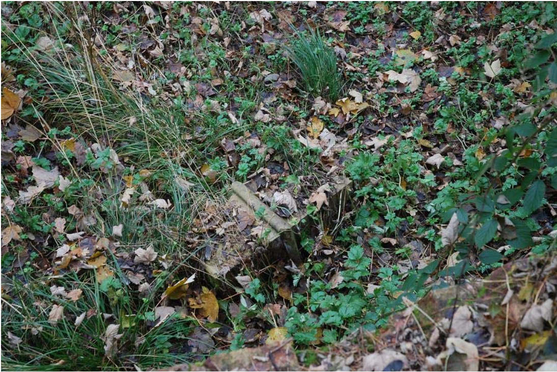
Plate 11: Vandalised pediment knocked off Sutton's Bridge
