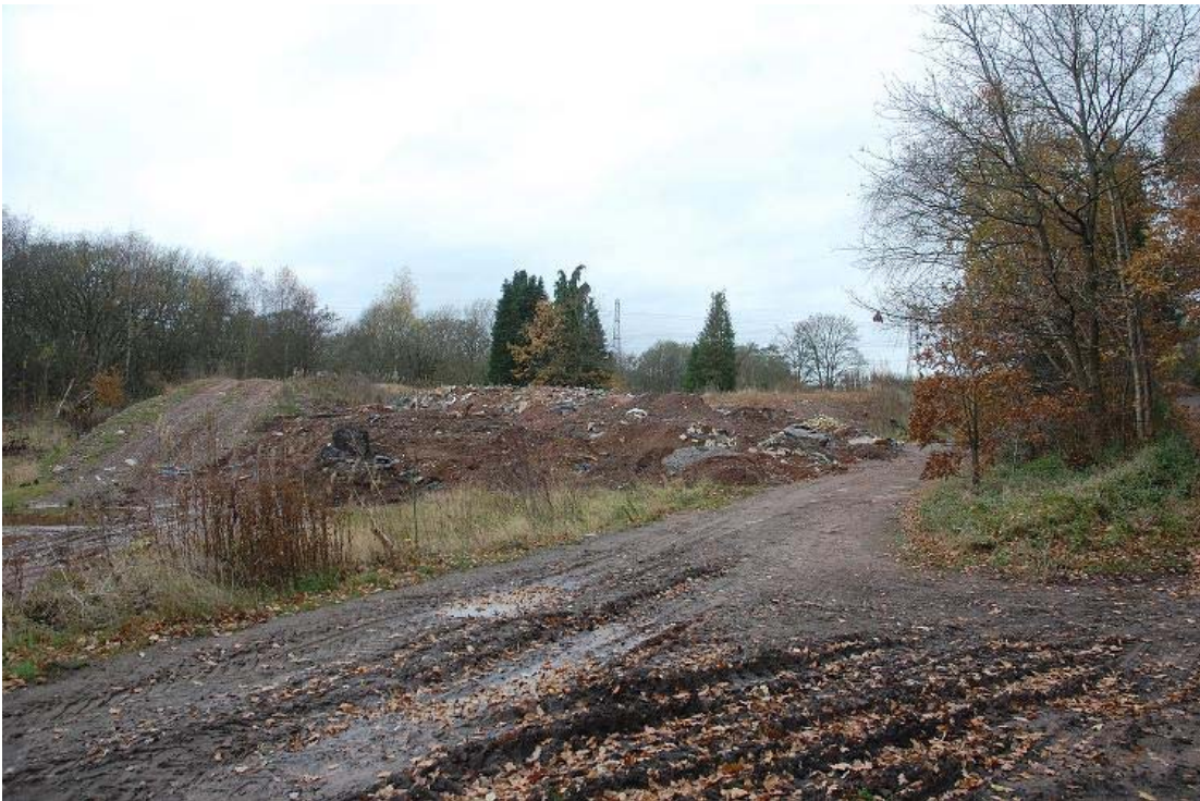
Plate 13: Demolition rubble on the site of former hospital buildings
