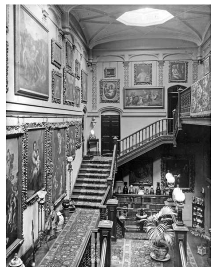
Staircase hall in 1897
