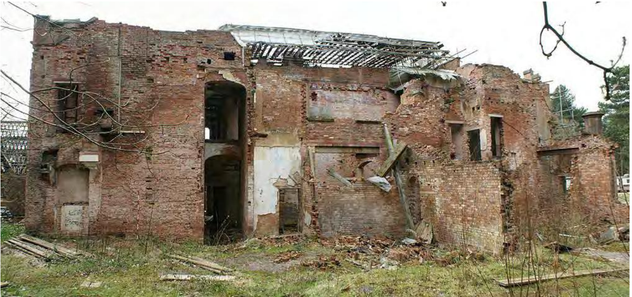
Plate 5: East elevation of Great Barr Hall
