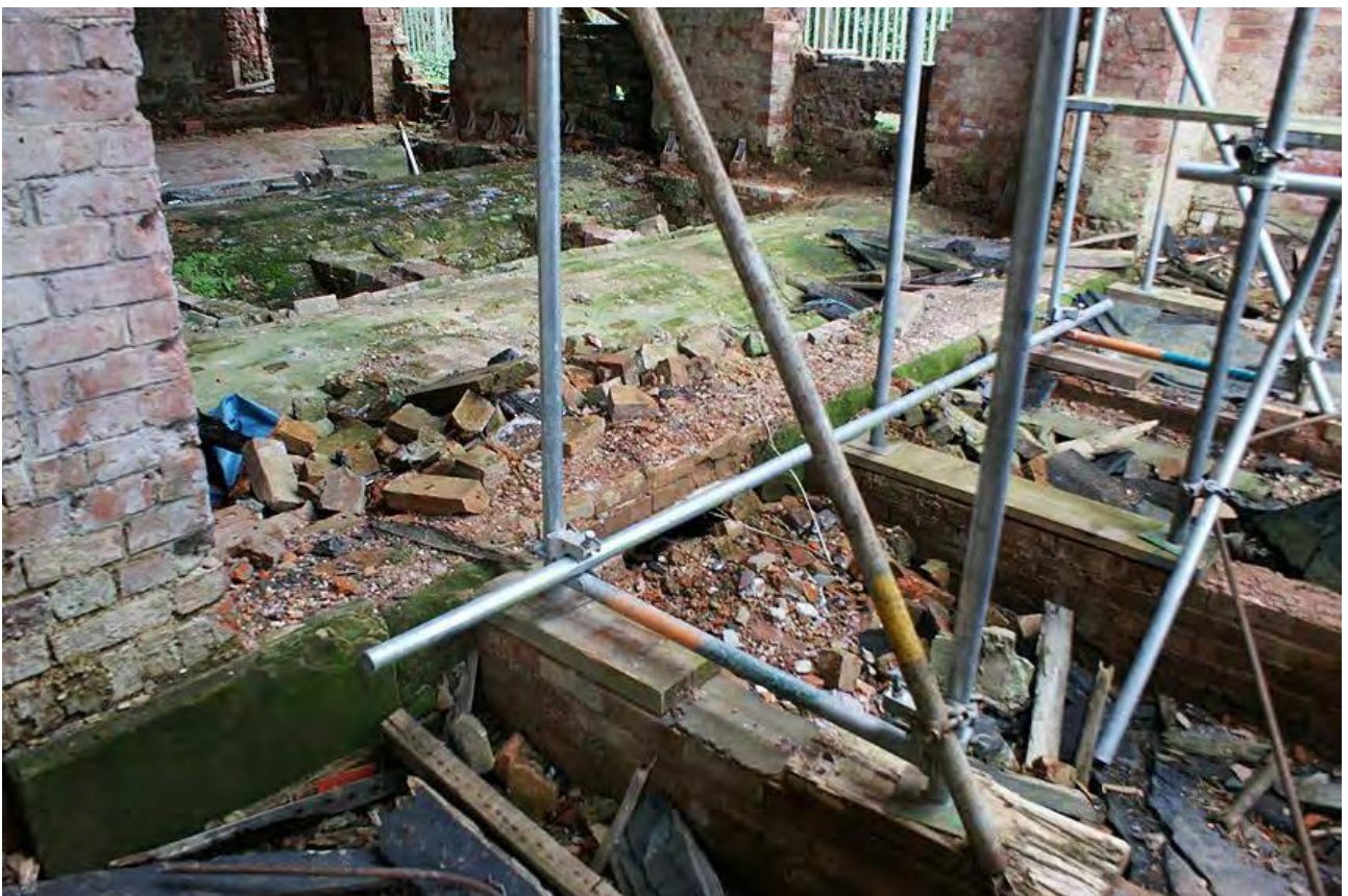
Plate 8: Original 1777 foundations of the west wall
