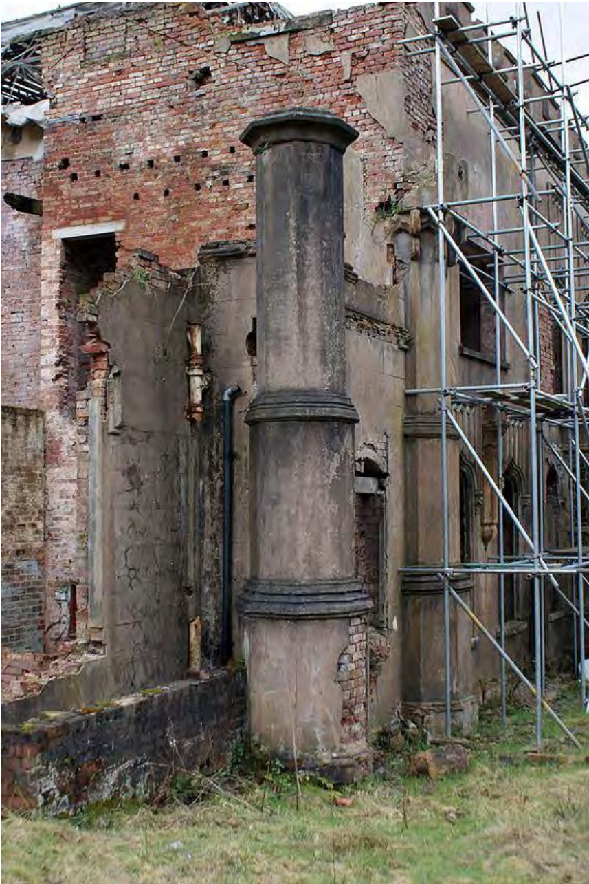
Plate 9: One of 1840s original polygonal buttresses
