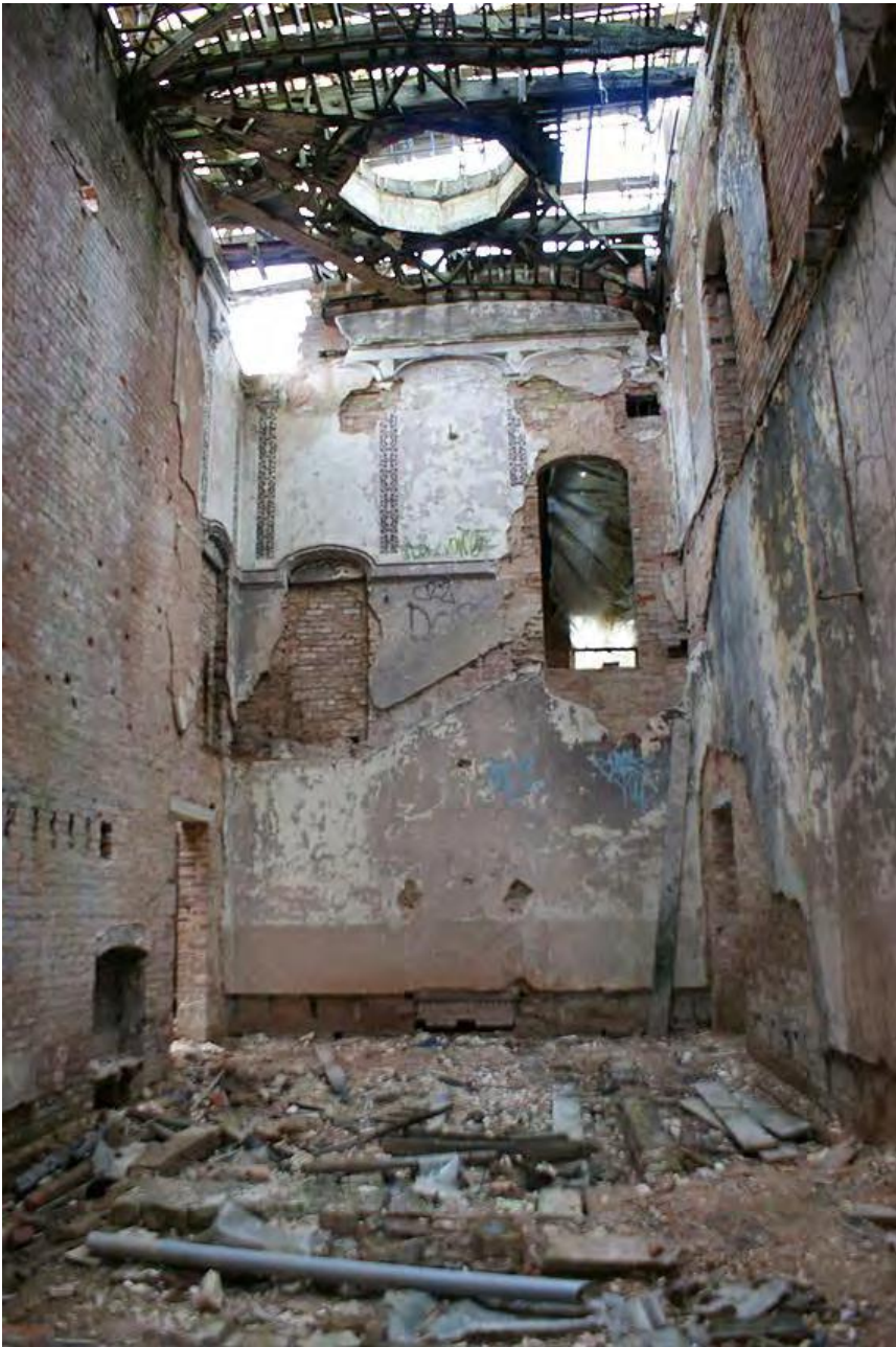
Plate 11: Interior of staircase hall
