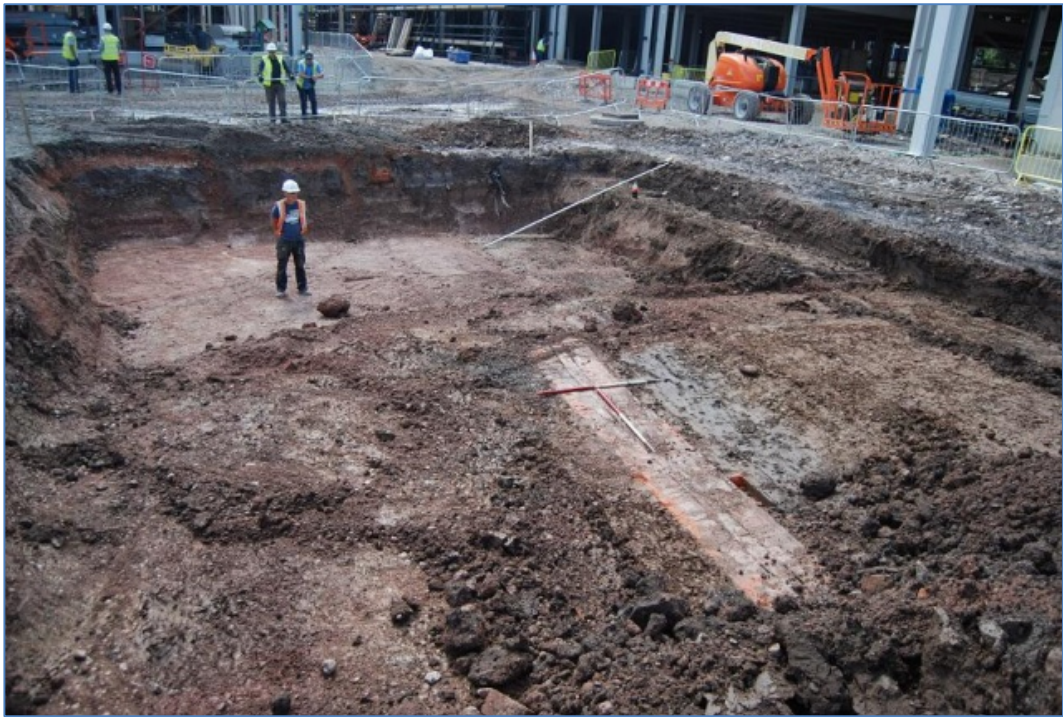
Plate 8 Attenuation tank excavation. View south.
