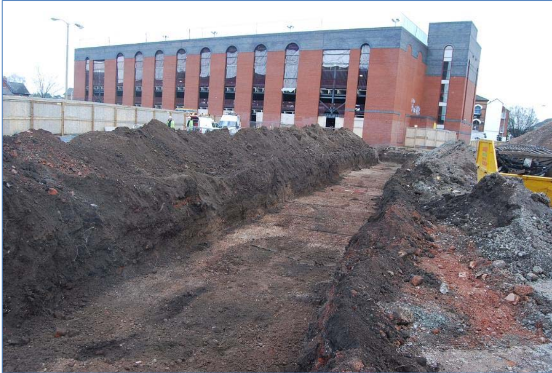
Plate 9 Monitoring Units 27-30 footings (trench 5). View northeast.
