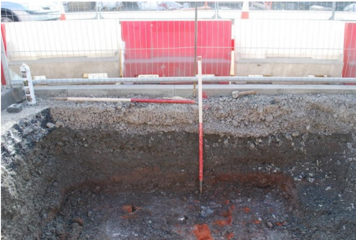
Plate 10 North-facing section of tree pit in central reservation.
