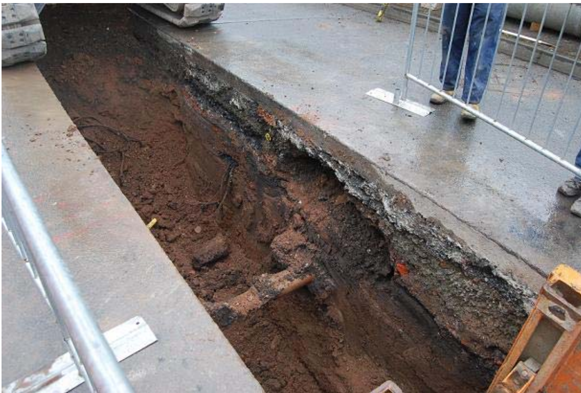
Plate 2 North facing section of trench 1, showing truncation by modern services. View South-east.
