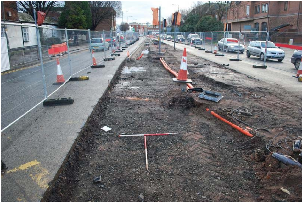
Plate 5 Ground reduction of Blueschool Street central reservation view East.
