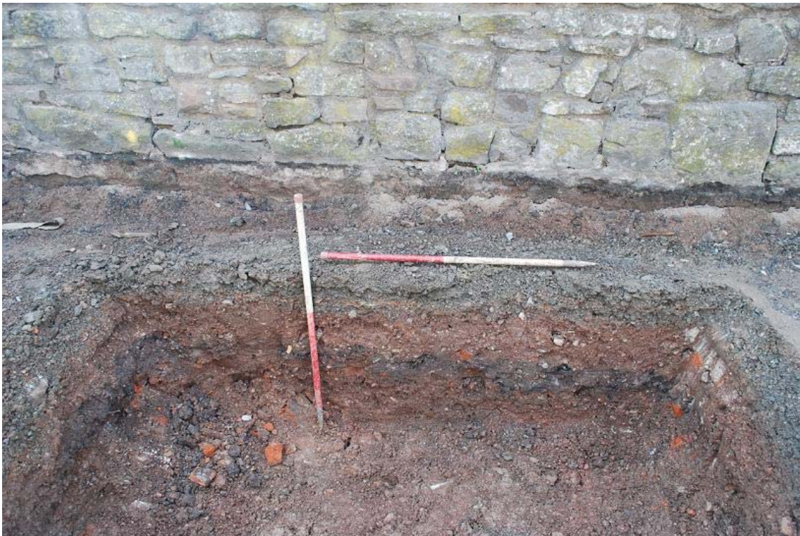
Plate 12 North facing section of Tree pit within Newmarket Street (Trench 7) showing made ground service trench backfill.
