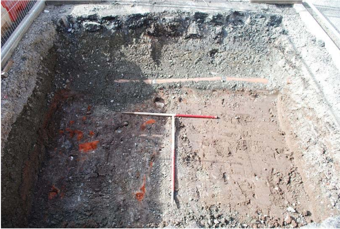
Plate 9 Example of Tree pit 1 in plan showing made ground, a service trench. View west.
