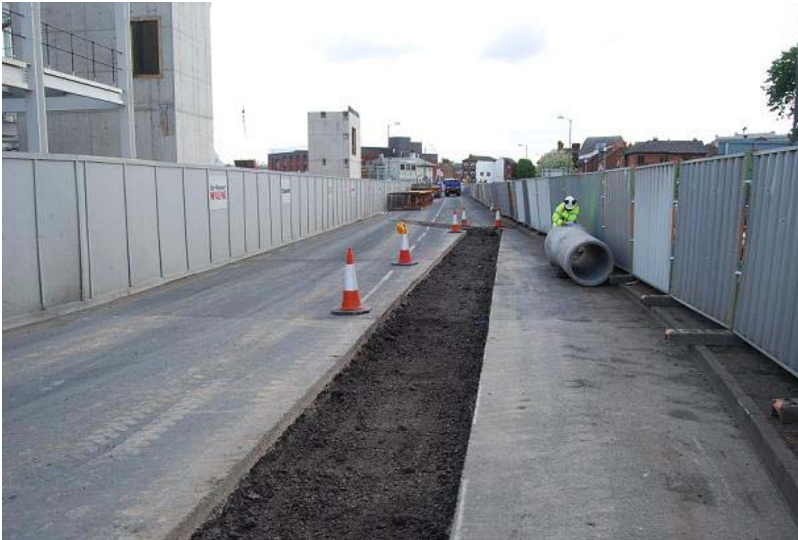
Plate 1 Tarmac stripped before excavation commenced. View North-east
