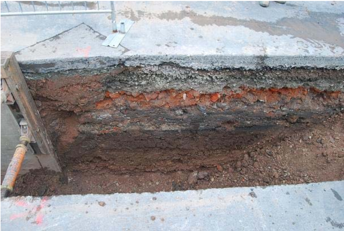
Plate 3 South facing section of trench 1.
