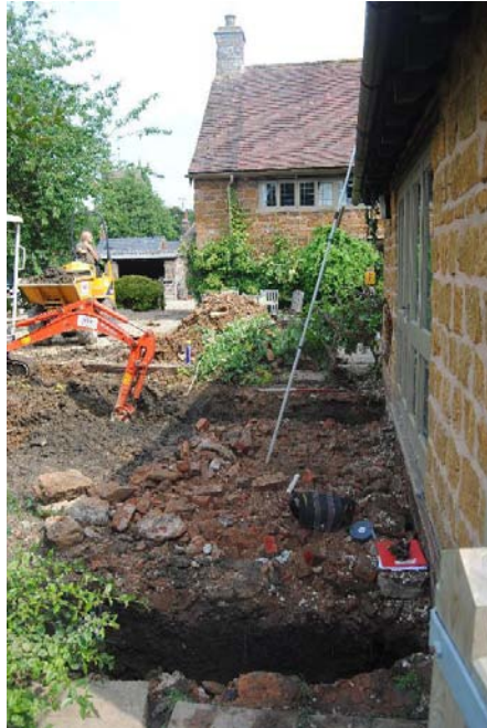
Plate 1 The site looking south-east
