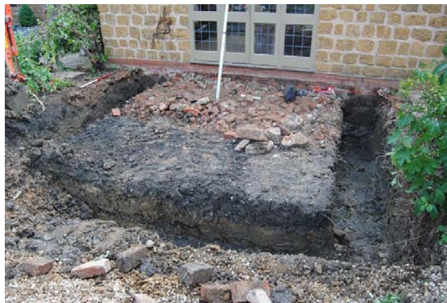
Plate 2 The excavated area looking south
