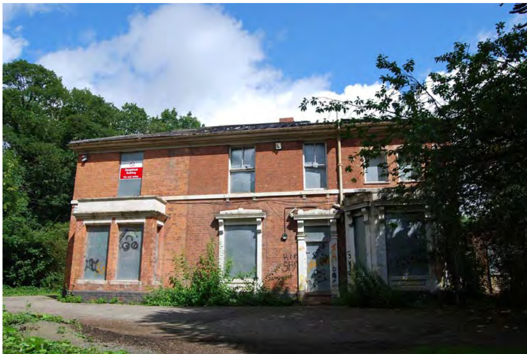
Plate 16: Saltwells House before demolition facing north
