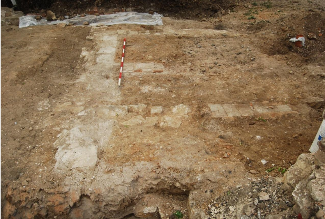
Plate 5: Wall 137 (left) returning to north as wall 140 (bottom), and abutted by walls 125, 134, and 135 (running left to right, from top to bottom); facing west
