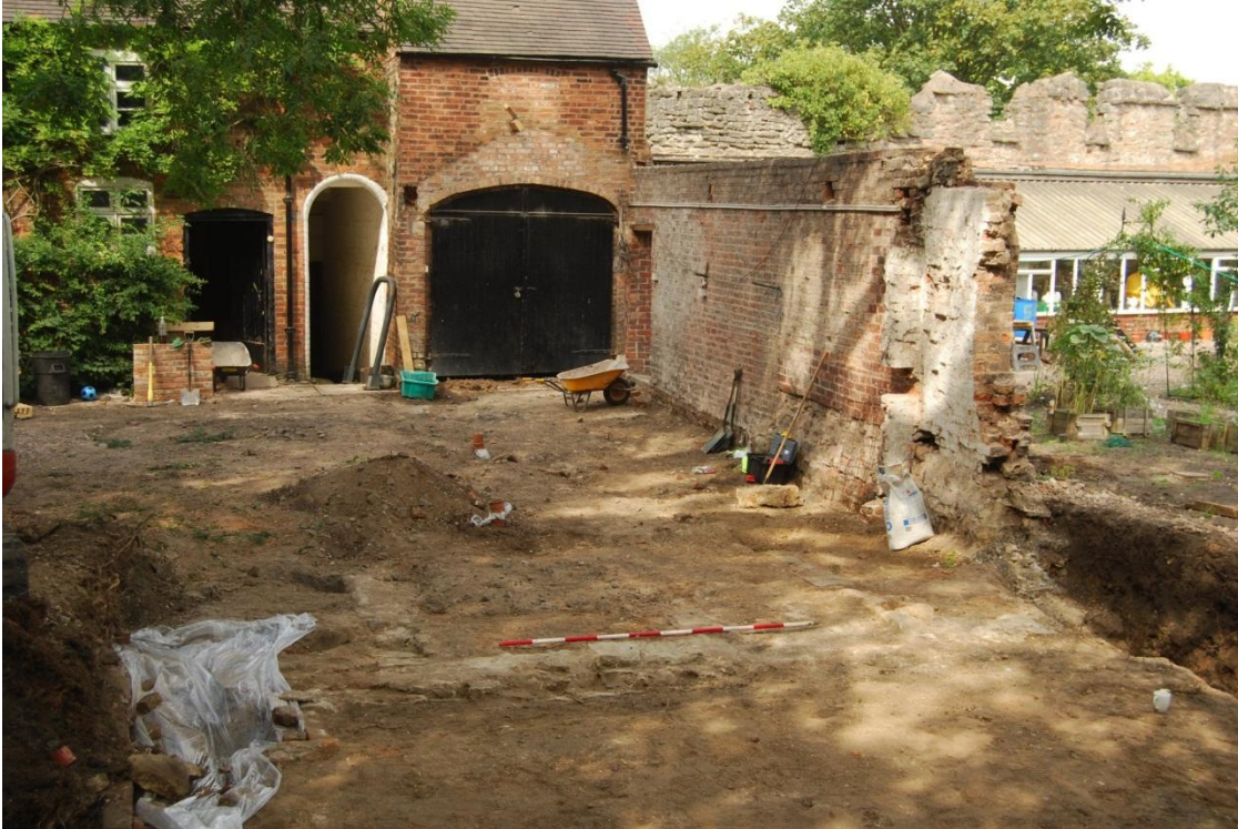
Plate 6: Walls 137 (foreground) and wall 140 (right), beneath wall 141, facing north-east
