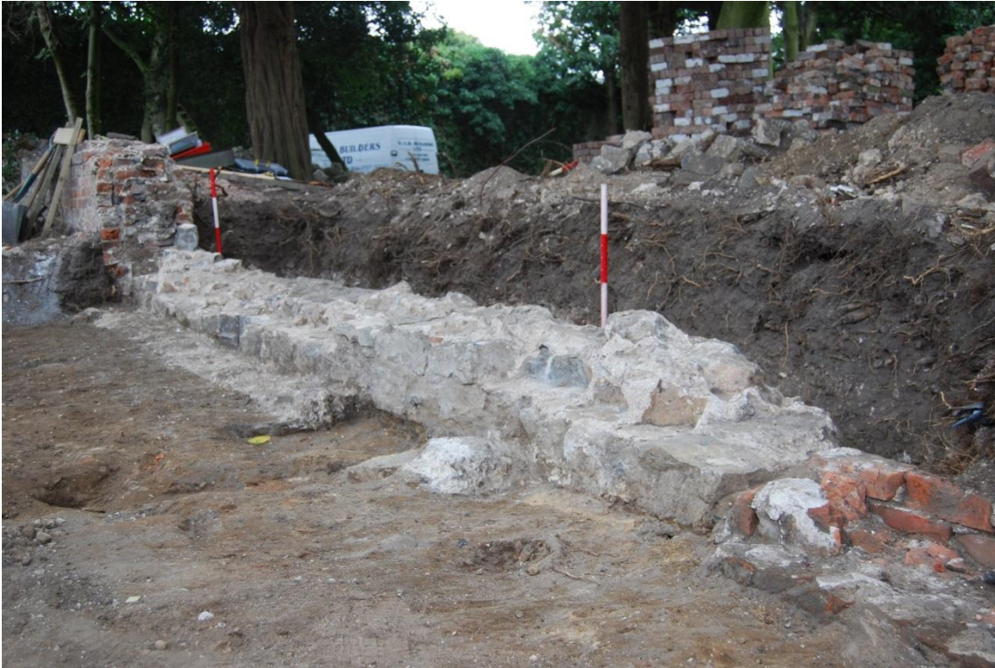
Plate 1: Wall 101, facing south-west
