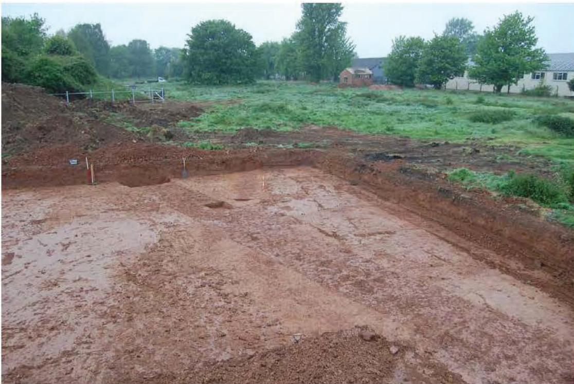
Plate 20: Ditches 8206 and 8208 in Trench 82, facing north-west
